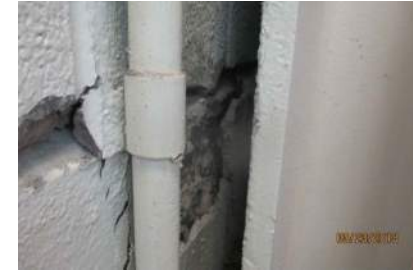
Existing Structural Condition
