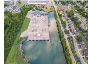
Conner Creek CSO Facility
