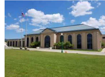
Water Works Park Water Treatment Plant
