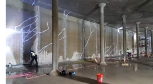
Imlay Booster Station: Sealing interior wall cracks
