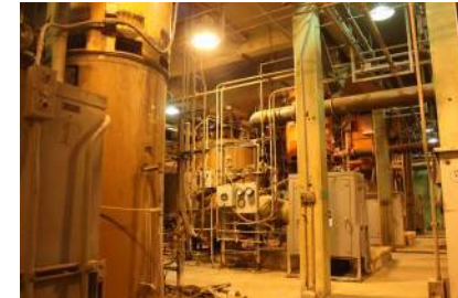
SFE Building, Basement
