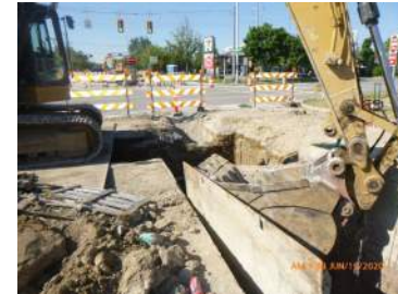
Construction on Merriman Rd.
