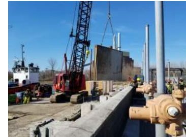
Effluent Relief Gate Repair
