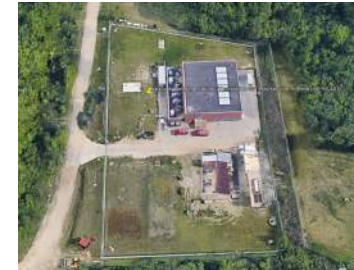
Existing Ypsi station
