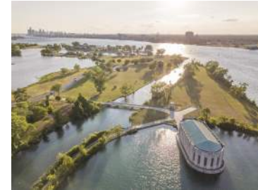
Belle Isle Intake
