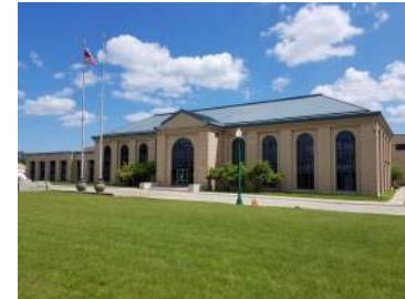
Water Works Park Water Treatment Plant
