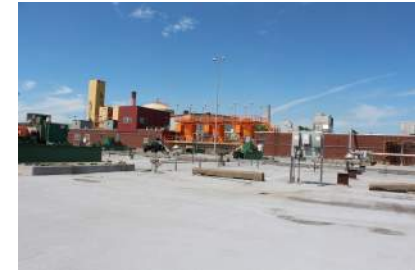
Aeration Basin 4, and ILP's 3, 4, and 7
