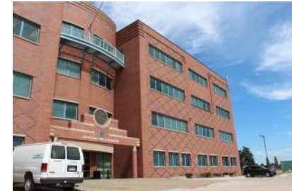
New Administration Building
