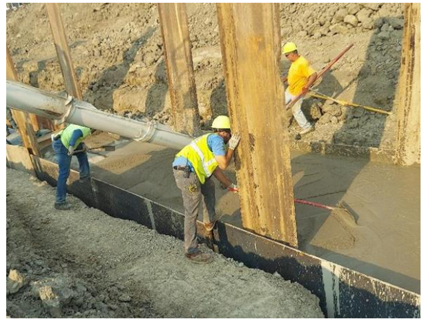
Pouring controlled low-strength material around installed steel pipe
