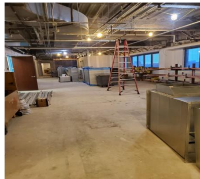
Duct work and drywall installation
