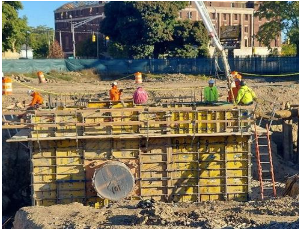
Crews pouring concrete for the reinforced walls at vault V-14
