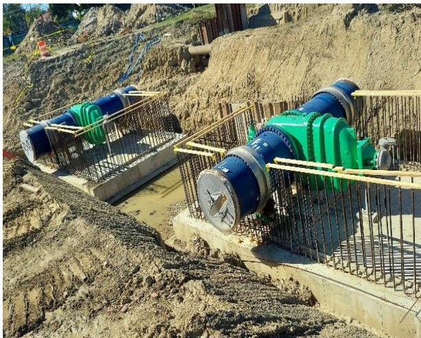
48" Gate Valves installed in vaults V-16 and V-17 with vault construction underway
