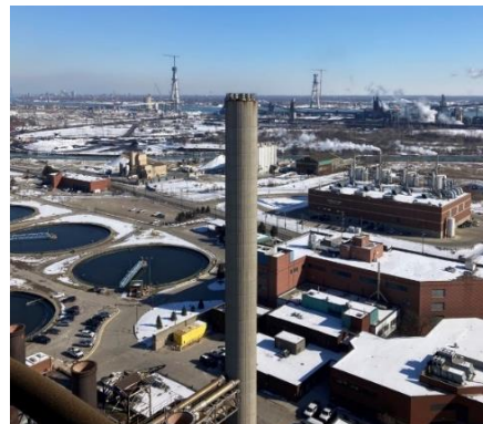
Photo from the top of the tall stack taken while servicing the radio (Note: adjacent tall stack, US Steel Facility on Zug, Gordie Howe Bridge and Canada).
