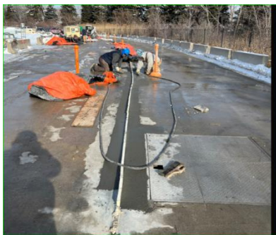
Shunt Channel Joint Repairs at HS
