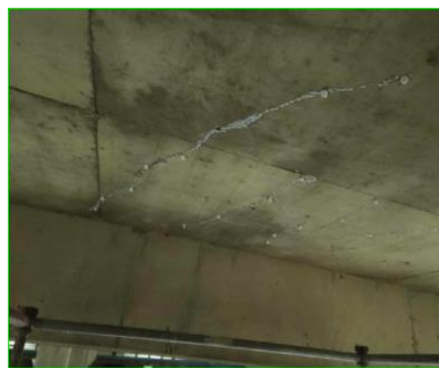
Ceiling Crack Repairs at OKW Basin
