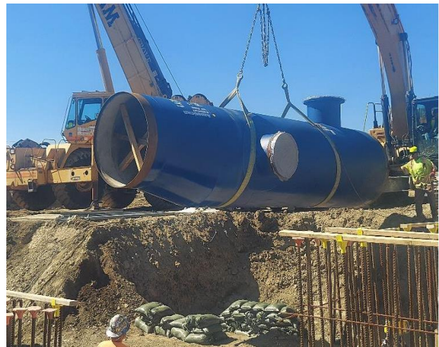
Installation of 72" steel pipe segment with access manhole
