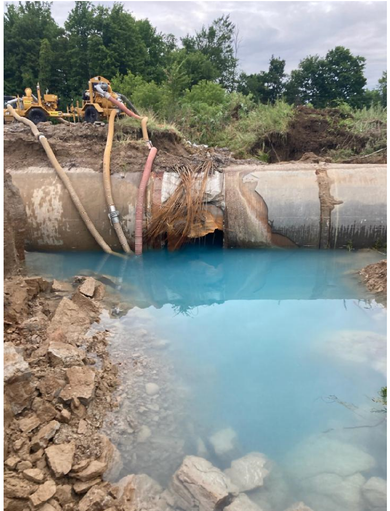
Figure 8 - Pumping water at break site
