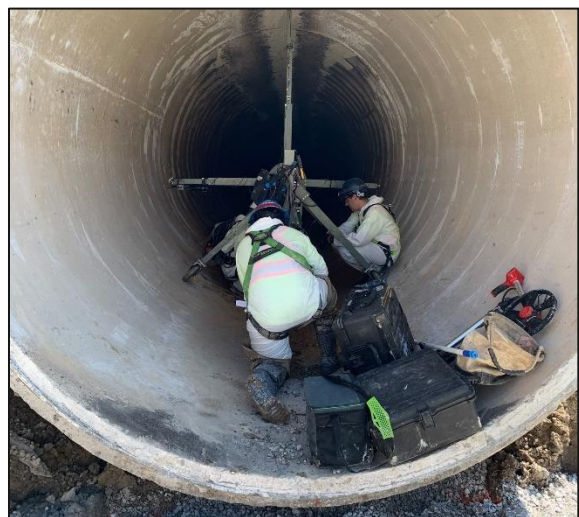
Figure 6. PICA crew completing the assembly of the NFT tool during the inspection of the East leg.
