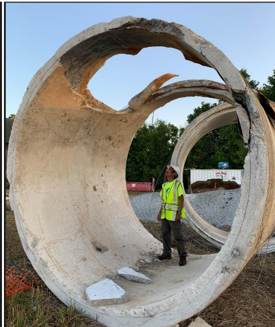
Figure 4b. PICA closely inspecting the inside of the ruptured pipe.
