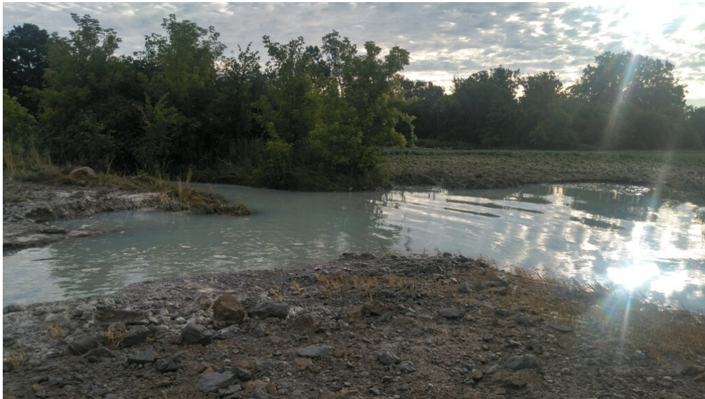
Figure 4 – Water main break on 120-inch Transmission Main, approximately 1/2 mile west of LHWTP
