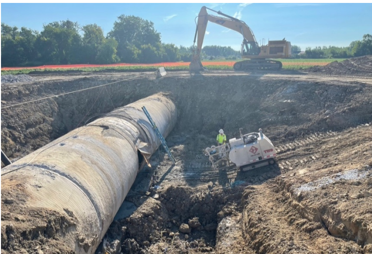
Figure 9 - Wire cutting and lifting section of main
