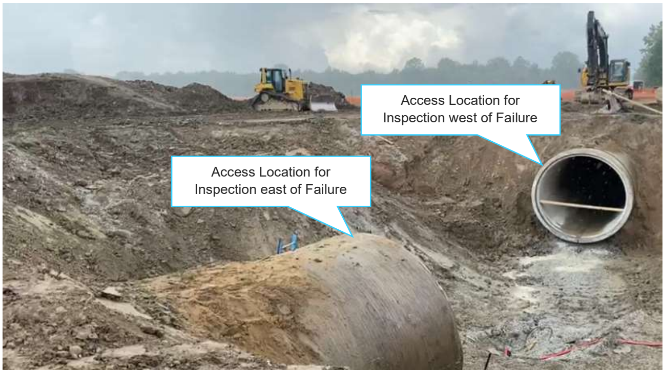
Figure 1.2: Primary Access for the Inspection was the Failure Location
