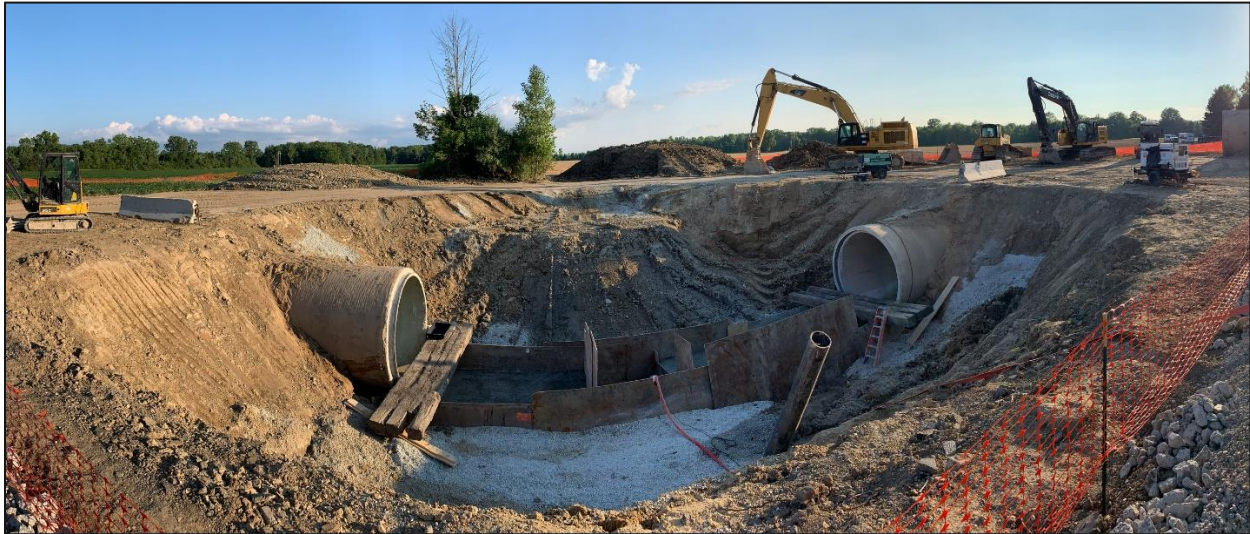
Figure 5. Panoramic image of the excavation, (looking south) prior to the concrete base pour and repairs.
