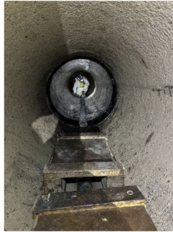
Looking E at Pipe 262 installed layers
