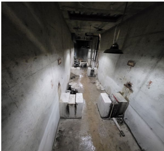
Demolished chain guards, gear, and saw cut concrete pedestals south drywell (basins #3 and #4)
