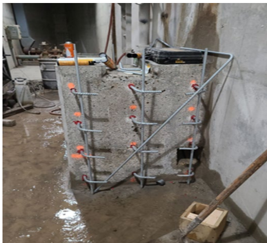
Concrete modifications to existing pedestals for pedestals south drywell (basins #3 and #4) new motors and drives
