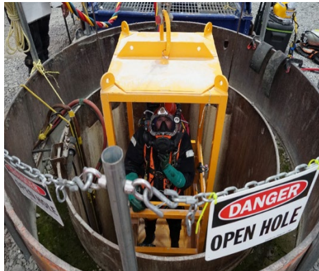
Diver being lowered into Northeast shaft to complete connection to tunnel
