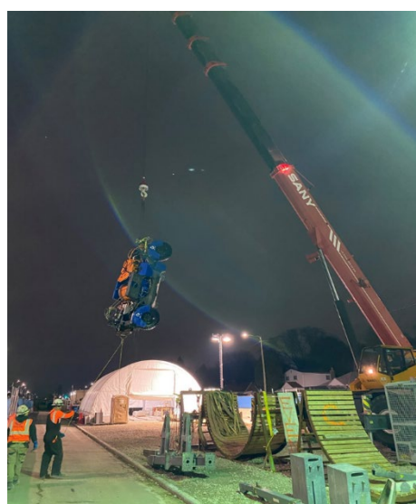
Rigging of vehicle used to move liner plate in the tunnel
