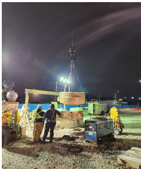
Removal of the Springwells 8-foot diameter core
