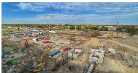
CIP#115001 Water Works Park Water Treatment Plant – Yard Piping #3 Photo submitted by: Jacob Magnum of Water and Field Services
