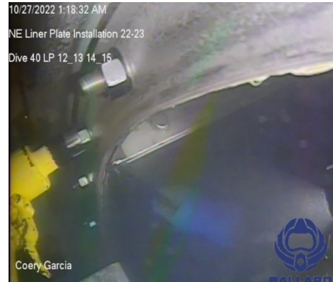
Bolting of Northeast liner plate Sections Nos. 22 and 23
