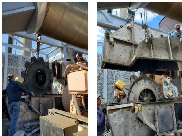
The new impeller for ID Fan 7 is being installed on the roof of Complex II. This job required the use of a 120-ton crane to lift the parts to the roof of the 5-story building
