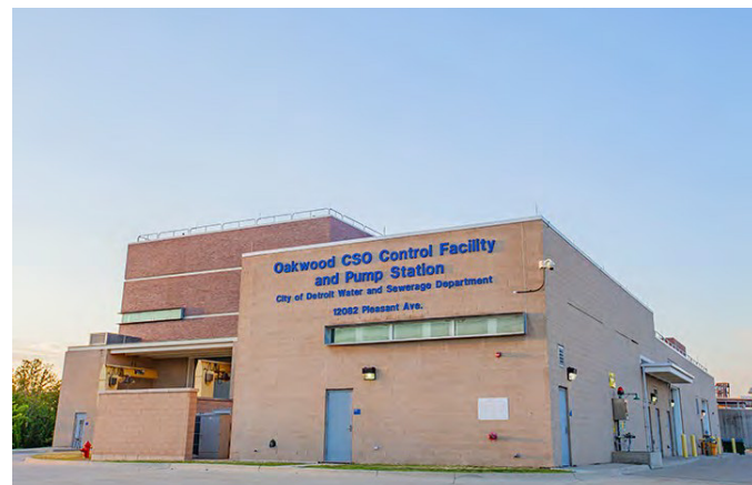
Figure 42. Oakwood CSO RTB
