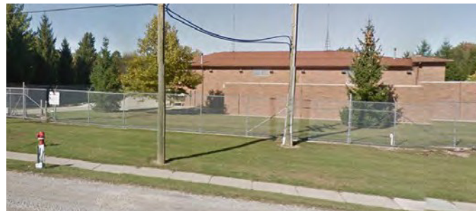
Figure 33. Rochester Pump Station
