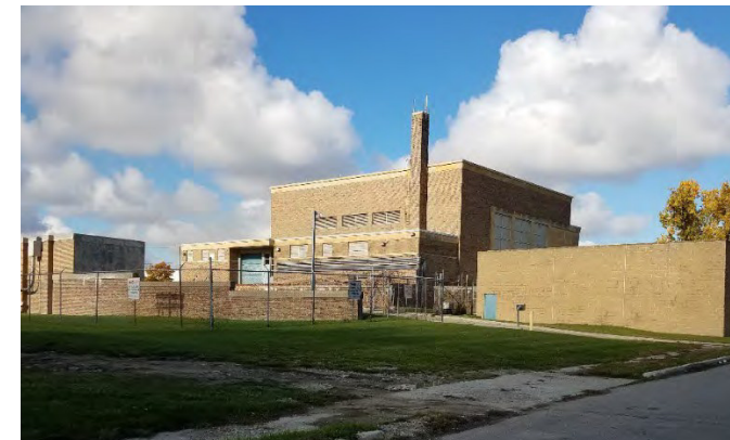
Figure 59. Freud Pump Station
