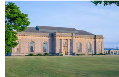
Water Works Park High Lift Pumping Station
