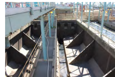
Pump Station 2, Grit channels
