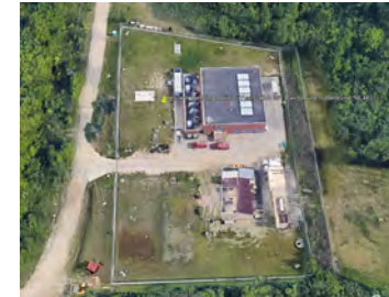
Existing Ypsi station
