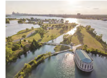
Belle Isle Intake
