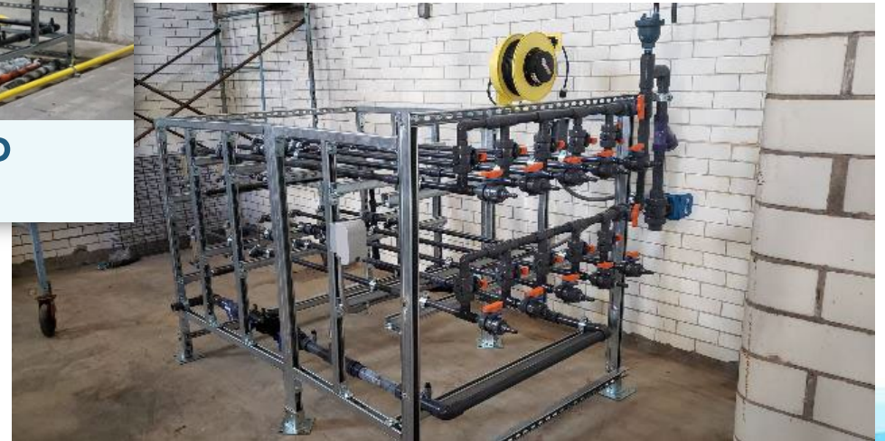
Water Works Park WTP
