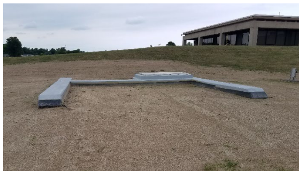
Lake Huron WTP reservoir access hatch AFTER
