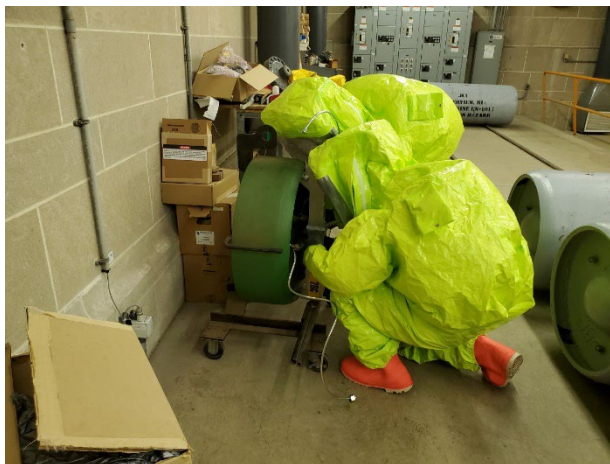
Second entry team installing B Kit device on tank end
