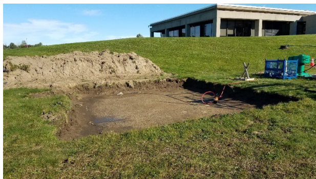
Lake Huron WTP reservoir access hatch BEFORE
