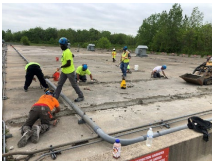
Joint repairs at Hubbell-Southfield
