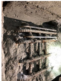
Conner Creek corbel repair
