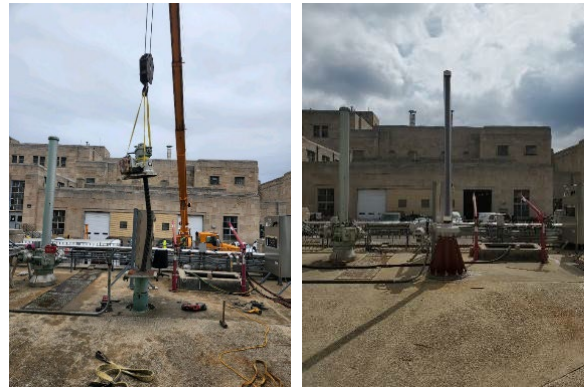
Left: Old stem during removal showing bend. Right: New stem and actuator
