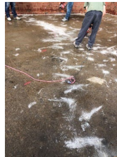
Baby Creek crack injection
