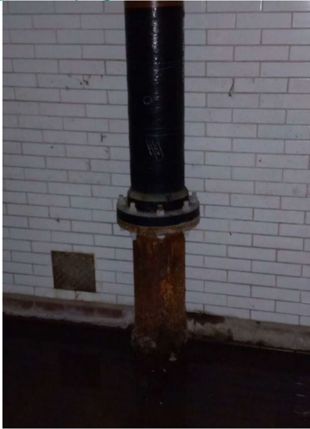
Figure 65: Vacuum System Piping New pipe transition to old pipe (heavy surface corrosion)
