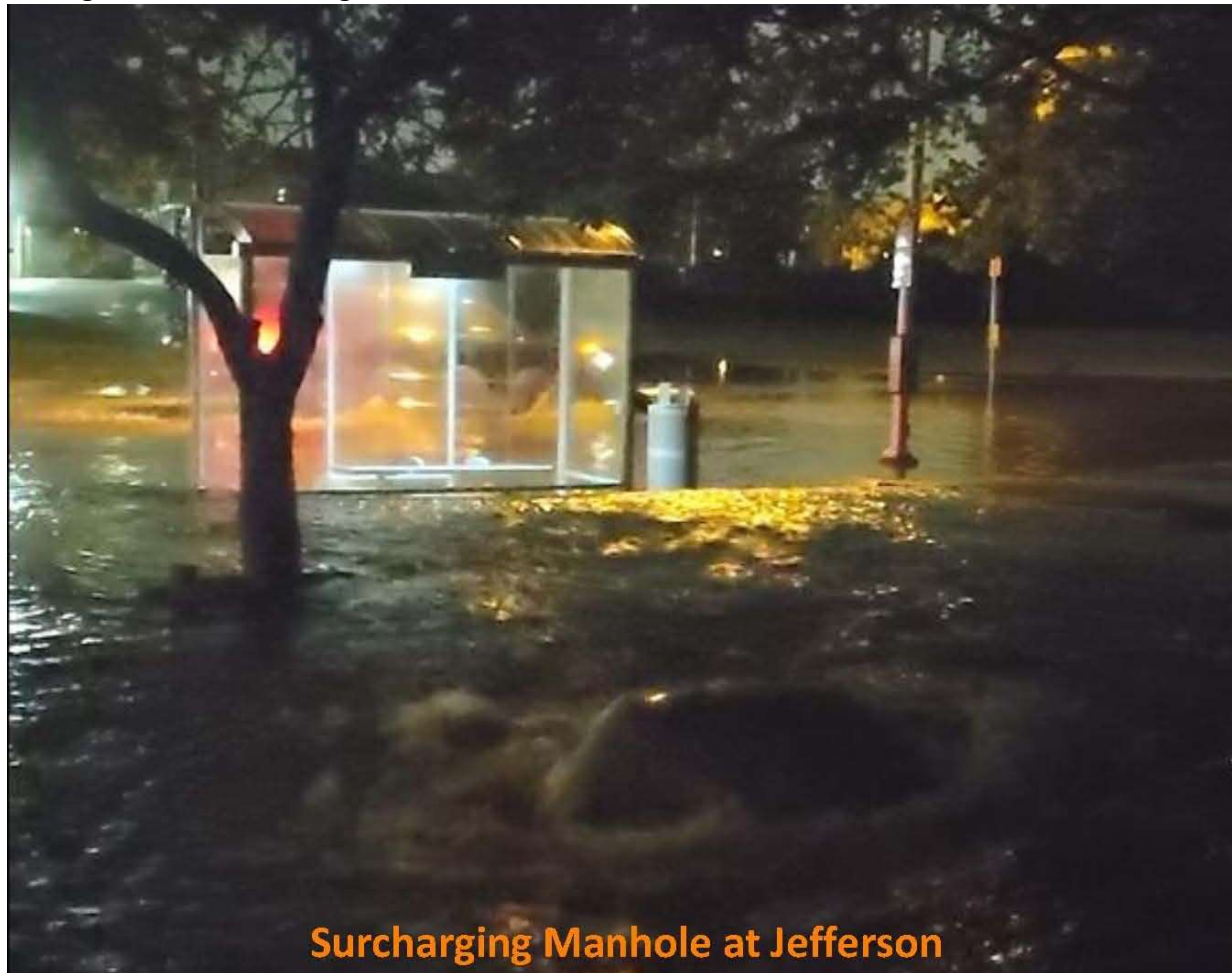
Figure 44. Overflowing Manhole at Grosse Pointe PS for the Storm of June 25-26, 2021
