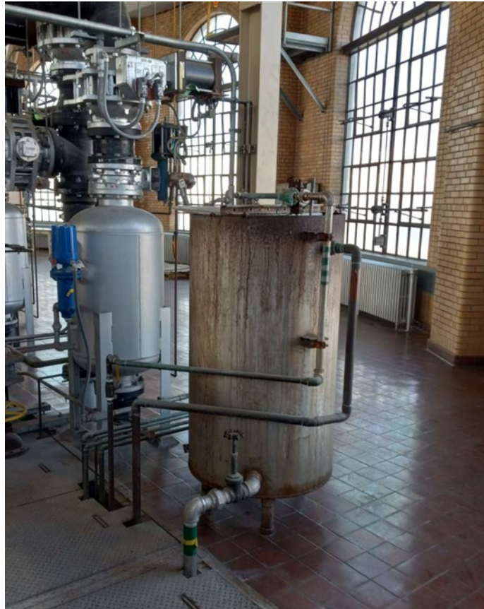
Figure 64: Seal Water Tank ~250 gallons (one tank for eight stormwater pumps)
