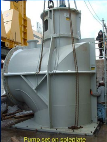
Pump set on soleplate
