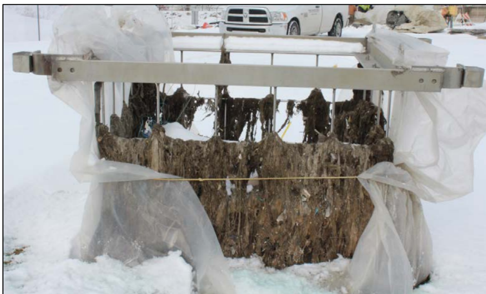
Figure 4-2. CCPS Influent Basket Screens Located at Both Inlets to the Sanitary Wet Well.
