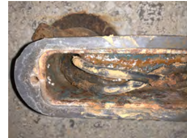
Leaking Conduit in Drain Vault
