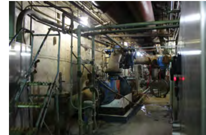
Sludge Feed pump in Complex A
