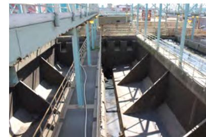
Pump Station 2, Grit channels
