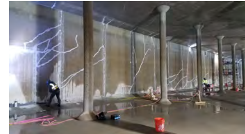
Imlay Booster Station: Sealing interior wall cracks
