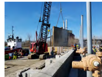
Effluent Relief Gate Repair
