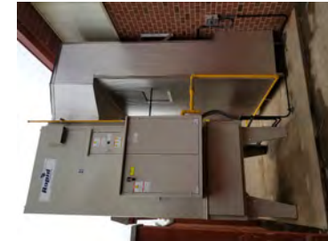
New Air Handling Unit
