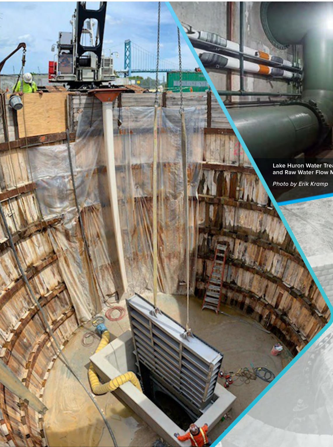
Lowering the Control Gate into Grand Connection Tunnel
