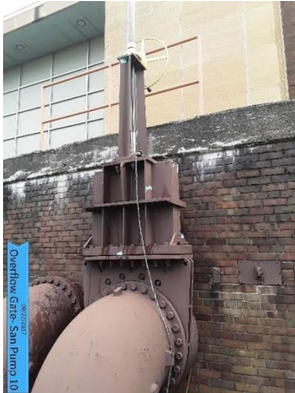
Figure 26: Existing Pump 10 Overflow Gate Valve to the Discharge Channel
