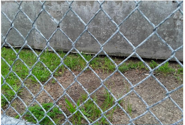
BUILDING- MAIN- Connor Creek Sewage Station - Transformer Containment Pad
