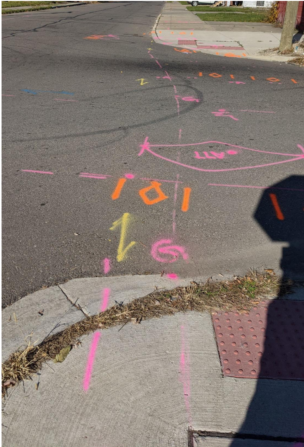
Photograph 5: Gas man and communications duct back crossing Freud Street at Conner Street looking north.
