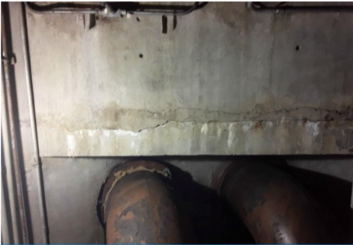
08/23/2017 G- MAIN- Freud Sewage Station - Lowest Level - Sump - 4th down from top floor
