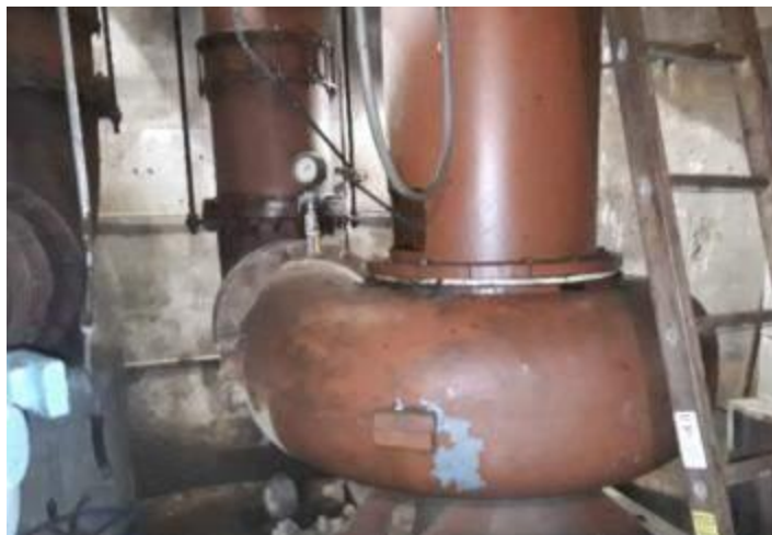
Figure 7: Existing Sanitary Pump
