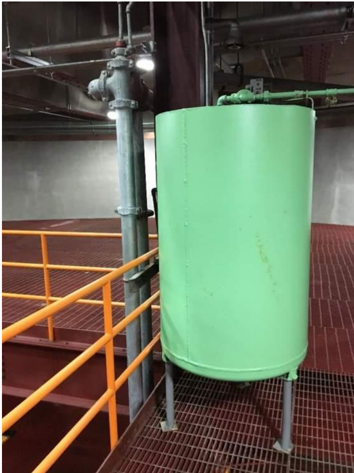
Figure 29: Seal Water System Break Tank
