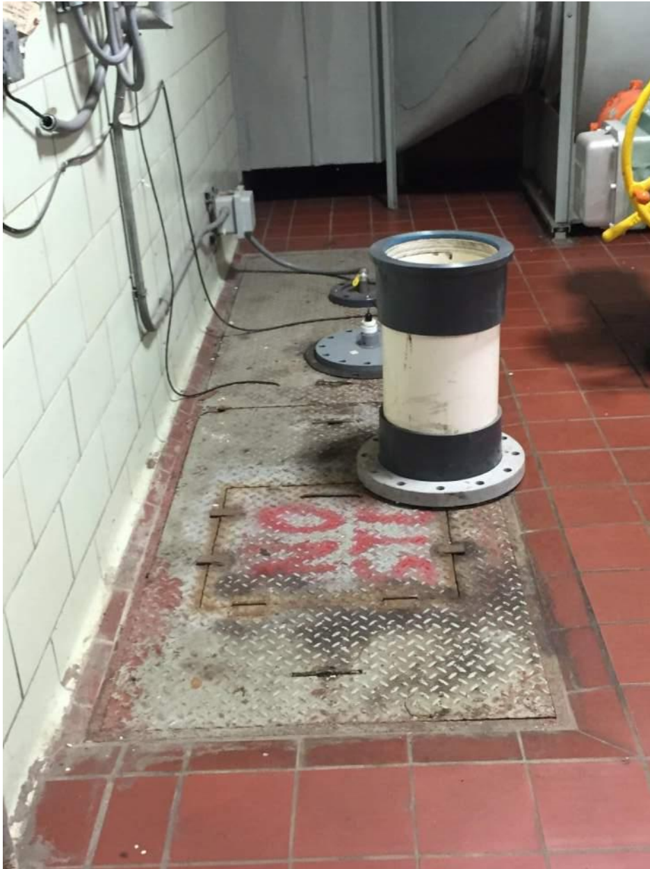
Figure 3: Existing Floor Hatch
