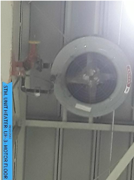
STM. UNIT HEATER- UH-4- MOTOR FLOOR 08/22/2017
