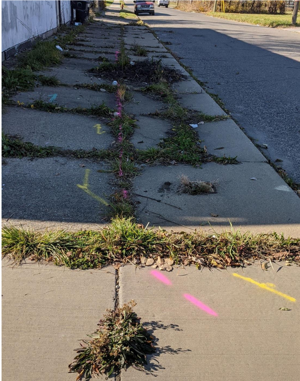
Photograph 9: Gas main along Freud Street west of Conner Street looking west.
