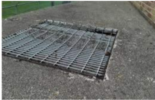
Figure 14: Existing West Exterior Top Slab
