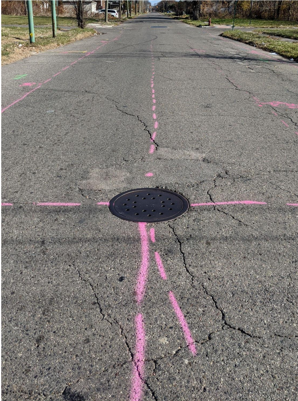
Photograph 11: Storm sewer along Freud Street and alley looking east
