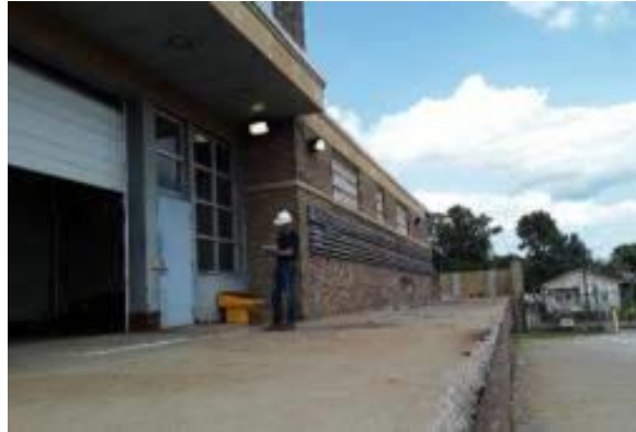
Figure 15: Existing South Exterior Top Slab
