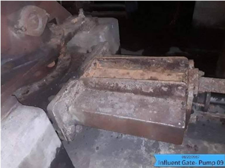
Figure 22: Existing Sanitary Pump Influent Gate Valve
