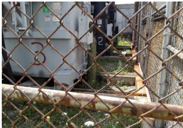
Figure 11: Existing Transformer Foundation
