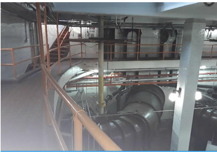
08/23/2017 DING- MAIN- Connor Creek Sewage Station - Second Floor Perimeter Walkways
