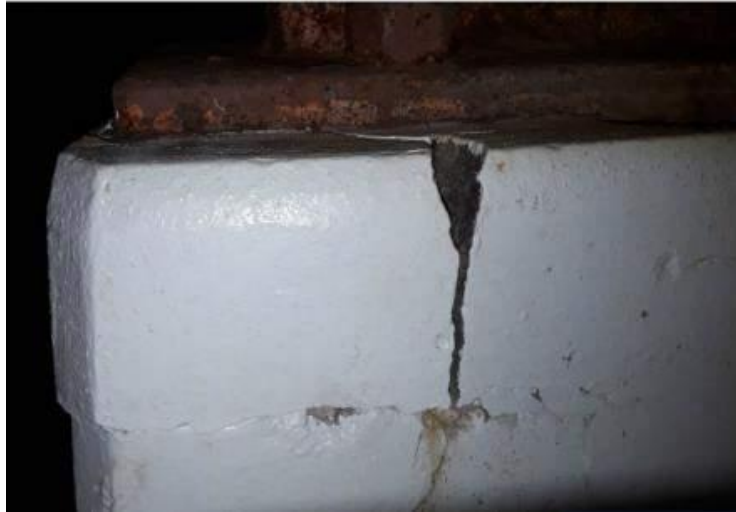
Figure 9: Existing Damaged Concrete Support Pier
