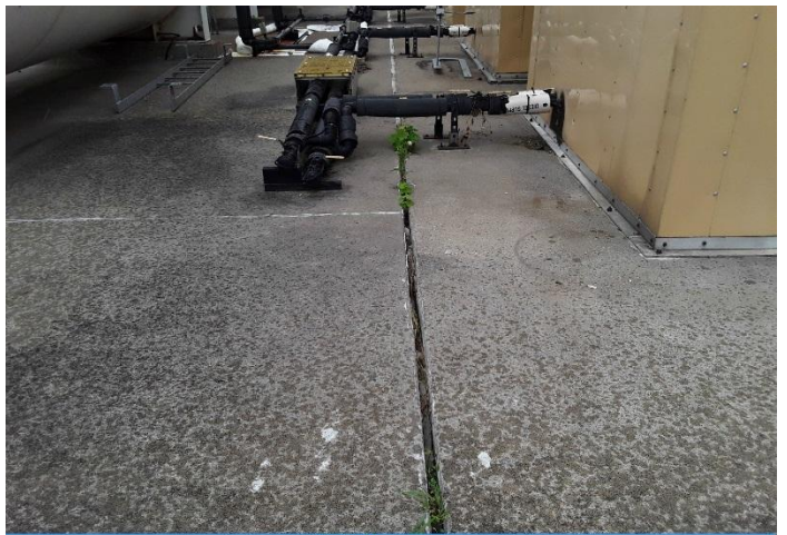
08/22/2017 G- MAIN- Connor Creek Sewage Station - Generator and Diesel Fuel Storage Pad
