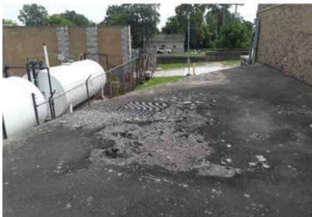
Figure 13: Existing East Exterior Top Slab
