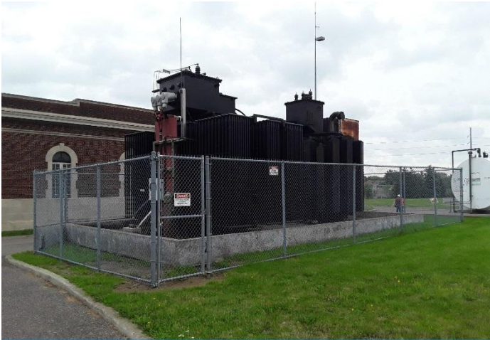
BUILDING- MAIN- Connor Creek Sewage Station - Transformer Containment Pad
