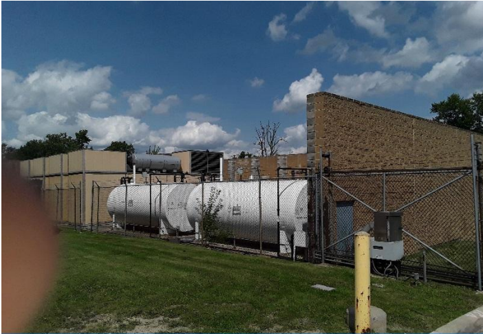
08/23/2017 reud Sewage Station - Generator Pad- Diesel Storage Tanks and Perimeter Wall
