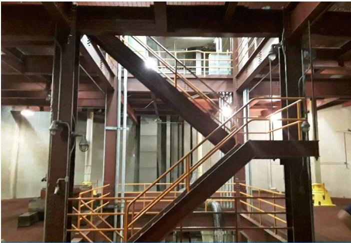
BUILDING- MAIN- Freud Sewage Station - Third Floor - 2nd down from top floor
