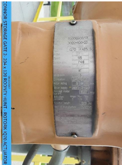
08/22/2017 CONNOR STORAGE GATE 2- 204 x 120 RODNEY HUNT - ROTORK IQ70 ACTUATOR
