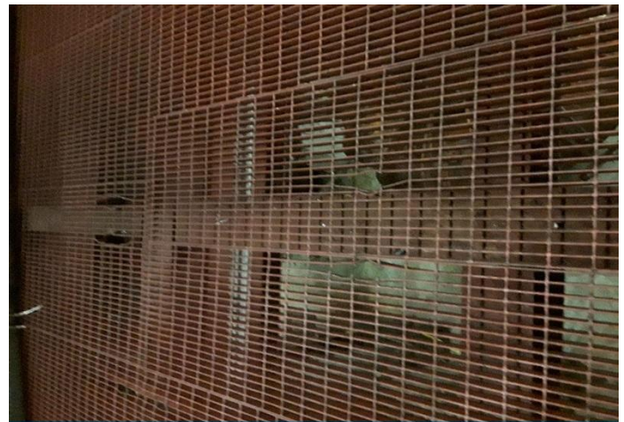
BUILDING- MAIN- Freud Sewage Station - Third Floor - 2nd down from top floor
