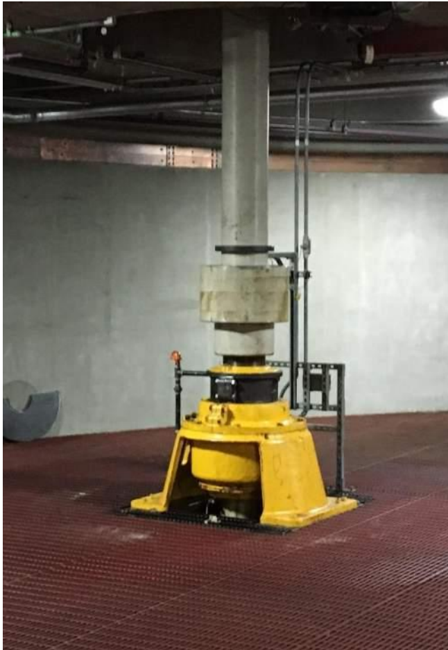
Figure 18: Existing Stormwater Pump Steady Bearing Assembly
