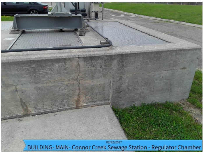
BUILDING- MAIN- Connor Creek Sewage Station - Regulator Chamber
