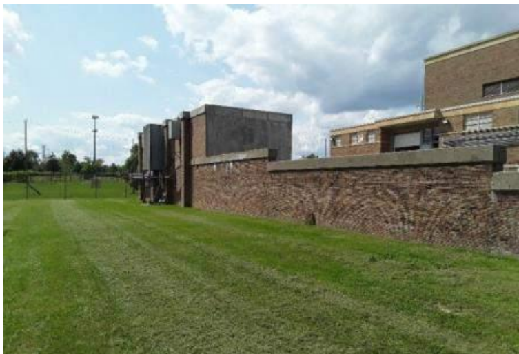
Figure 12: Existing South Site Retaining Wall
