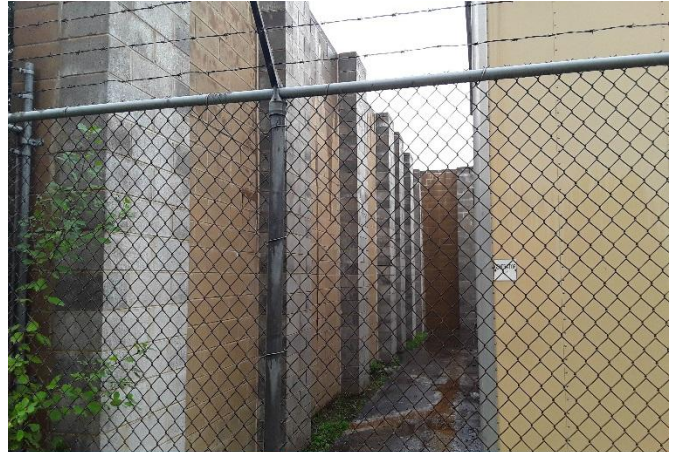
08/22/2017 reud Sewage Station - Generator Pad- Diesel Storage Tanks and Perimeter Wall
