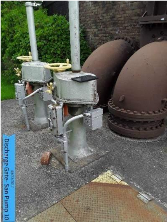
Figure 27: Existing Pump 9 and 10 Discharge Gate Valve
