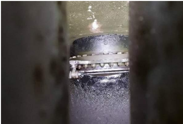
Figure 25: Existing Pump 10 Flap Gate
