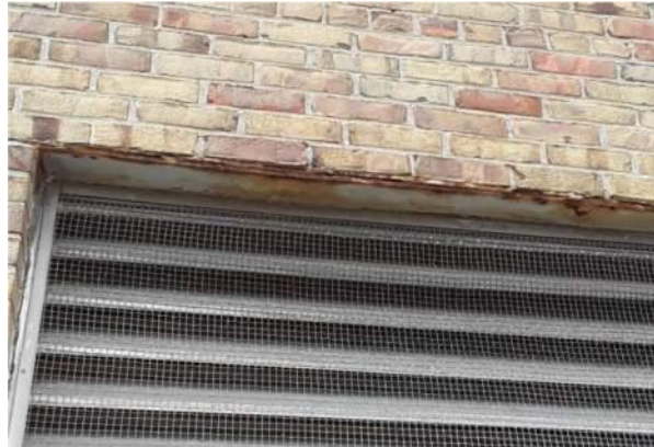
Figure 4: Existing Steel Lintel
