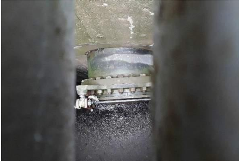
Figure 24: Existing Pump 9 Flap Gate
