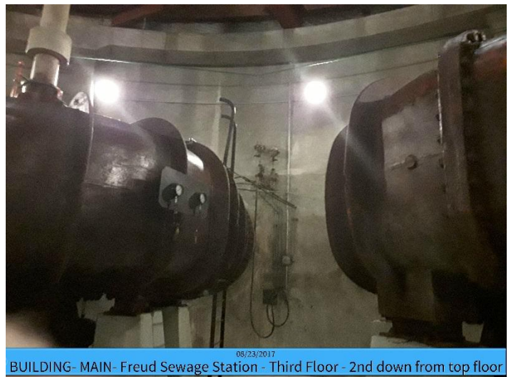
BUILDING- MAIN- Freud Sewage Station - Third Floor - 2nd down from top floor
