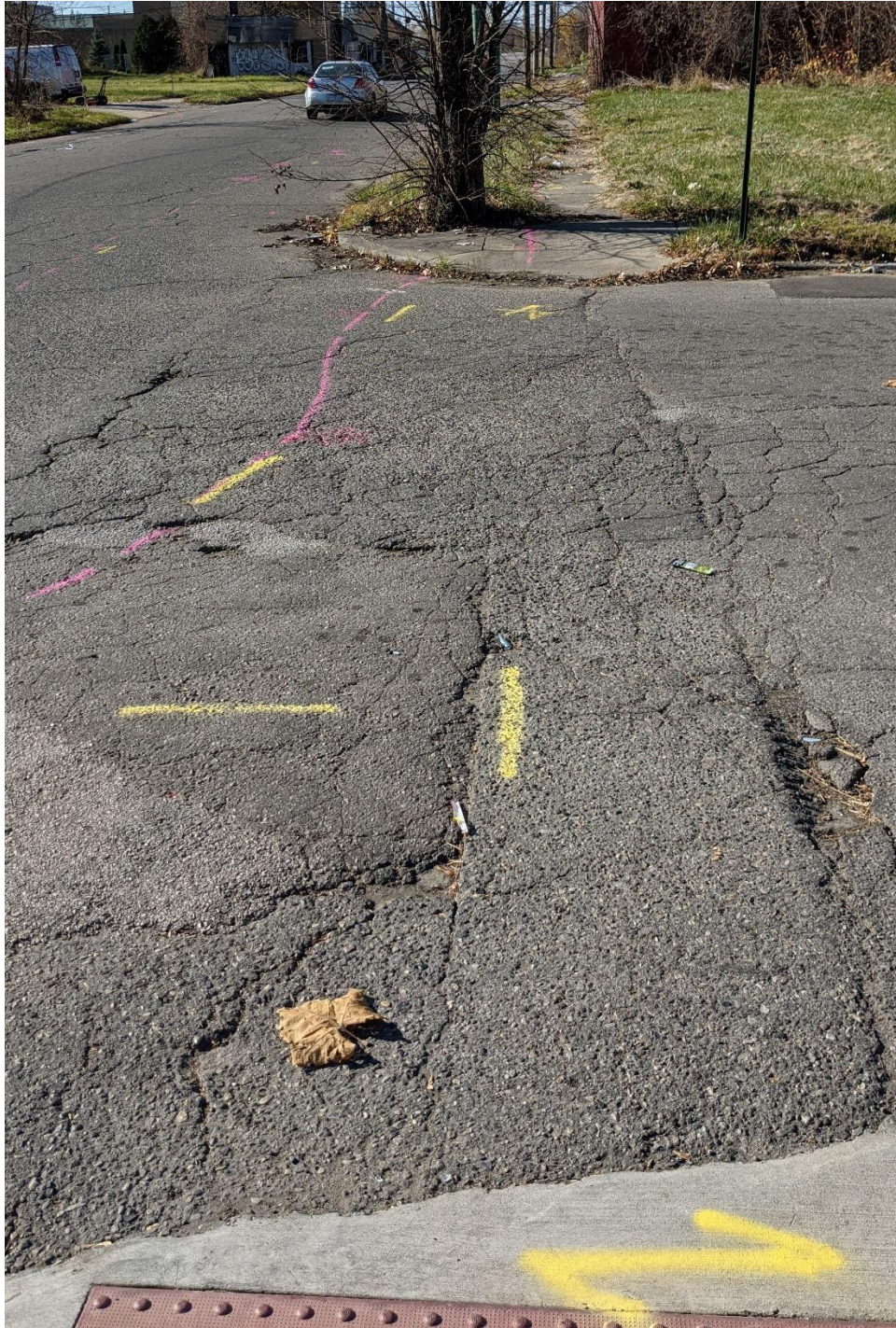
Photograph 8: Gas main along Freud Street at Navahoe Street looking west
