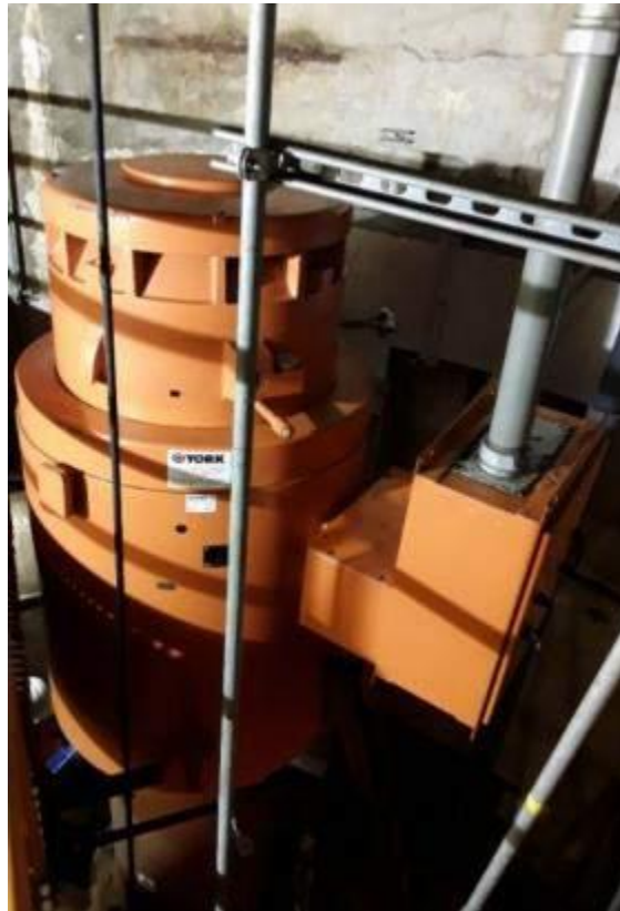
Figure 8: Existing Sanitary Motor
