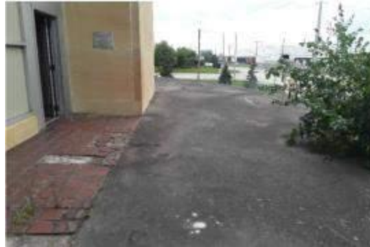
Figure 16: Existing North Exterior Top Slab
