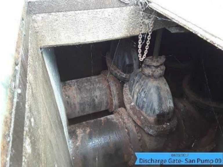
Figure 28: Existing Pump 9 and 10 Discharge Gate Valve
