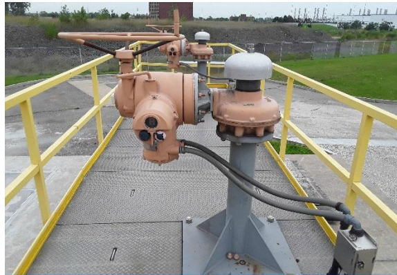
08/22/2017 CONNOR STORAGE GATE 2- 204 x 120 RODNEY HUNT - ROTORK IQ70 ACTUATOR
