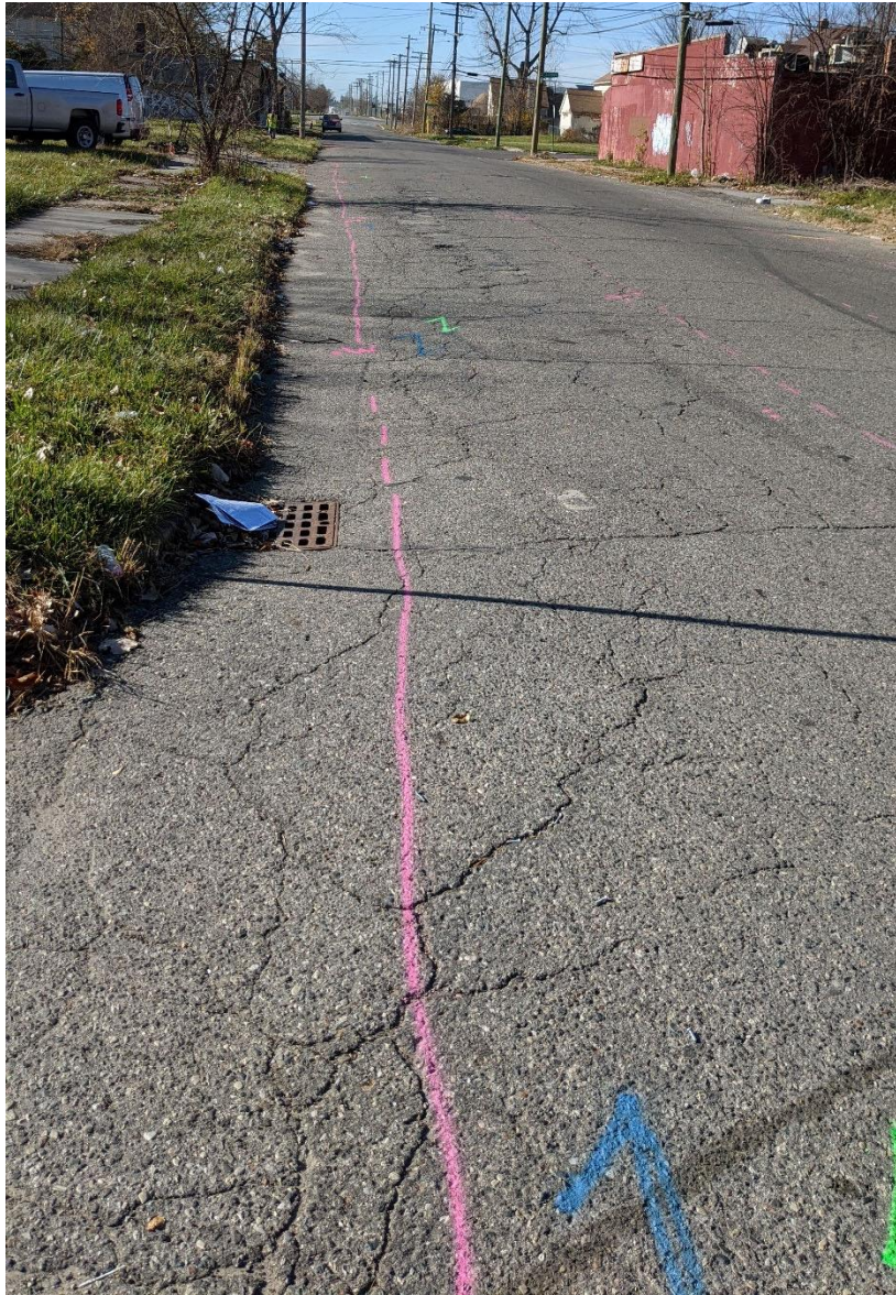
Photograph 1: 16" Watermain along Freud Street looking west.
