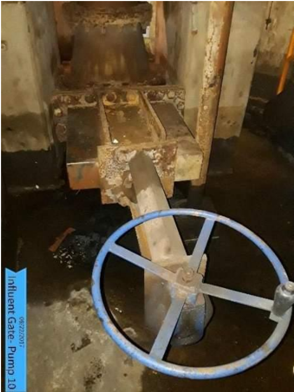
Figure 23: Existing Sanitary Pump Influent Gate Valve
