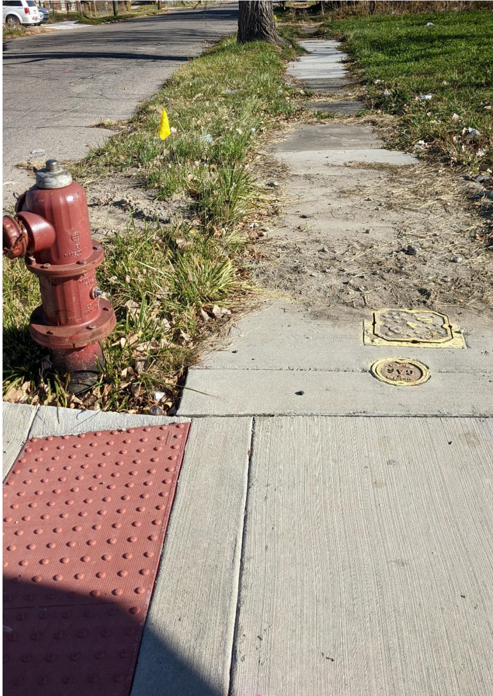
Photograph 6: Gas valve at southeast corner of Freud Street and Navahoe Street looking east.
