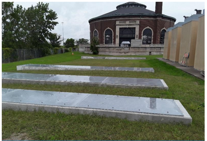
Connor Creek Sewage Station - Gate Structure and Raised Stop Log Structures
