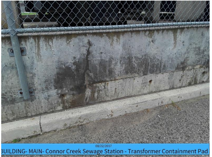
BUILDING- MAIN- Connor Creek Sewage Station - Transformer Containment Pad
