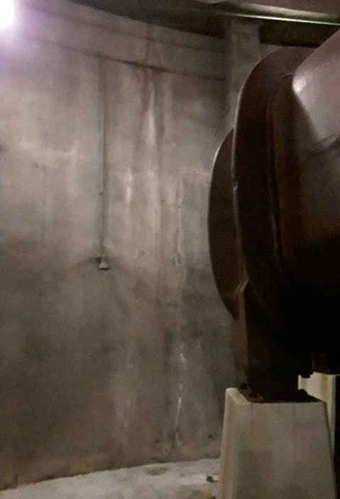
BUILDING- MAIN- Freud Sewage Station - Third Floor - 2nd down from top floor 08/23/2017
