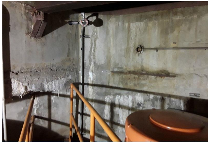
08/23/2017 G- MAIN- Freud Sewage Station - Lowest Level - Sump - 4th down from top floor
