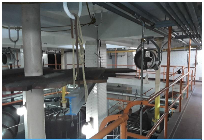
08/23/2017 DING- MAIN- Connor Creek Sewage Station - Second Floor Perimeter Walkways
