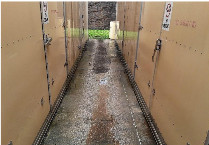
08/22/2017 reud Sewage Station - Generator Pad- Diesel Storage Tanks and Perimeter Wall
