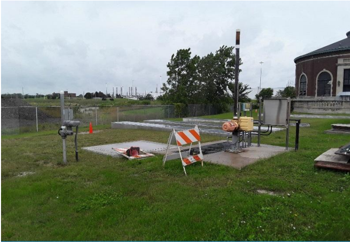
Connor Creek Sewage Station - Gate Structure and Raised Stop Log Structures
