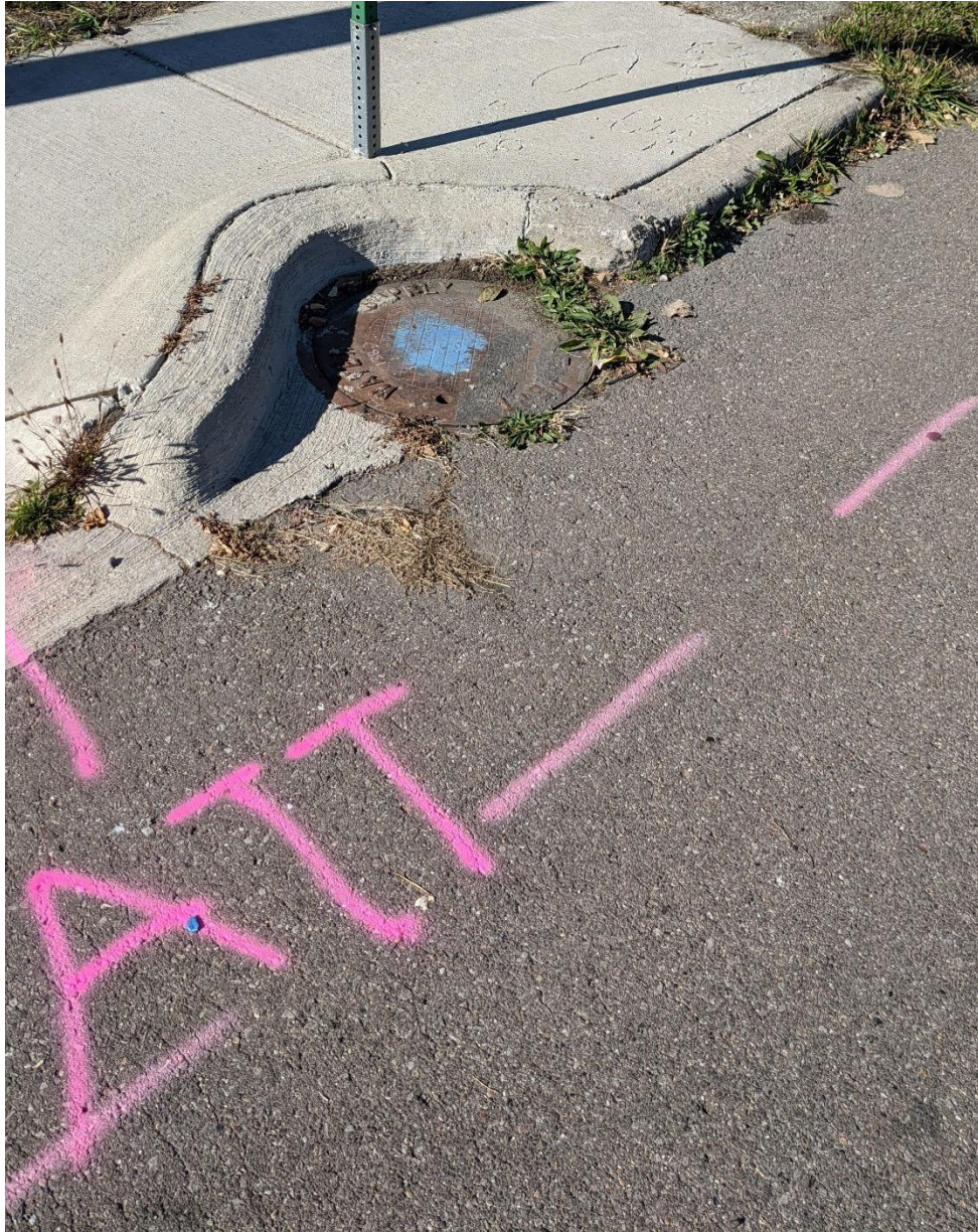
Photograph 3: Water gate valve and ATT communication at northwest corner of Freud Street and Conner Street.
