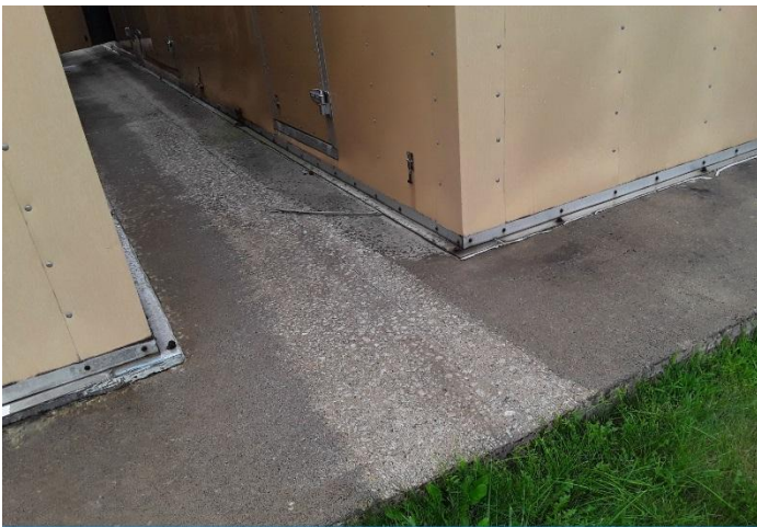
08/22/2017 G- MAIN- Connor Creek Sewage Station - Generator and Diesel Fuel Storage Pad
