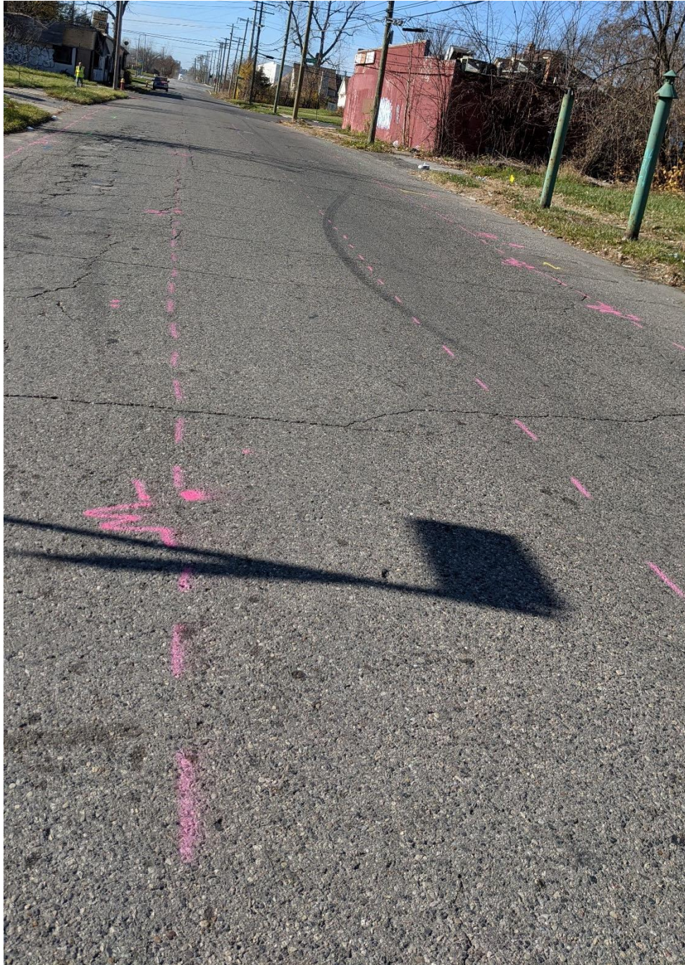
Photograph 2: 24" Watermain, storm sewer, and gas main along Freud Street looking west.
