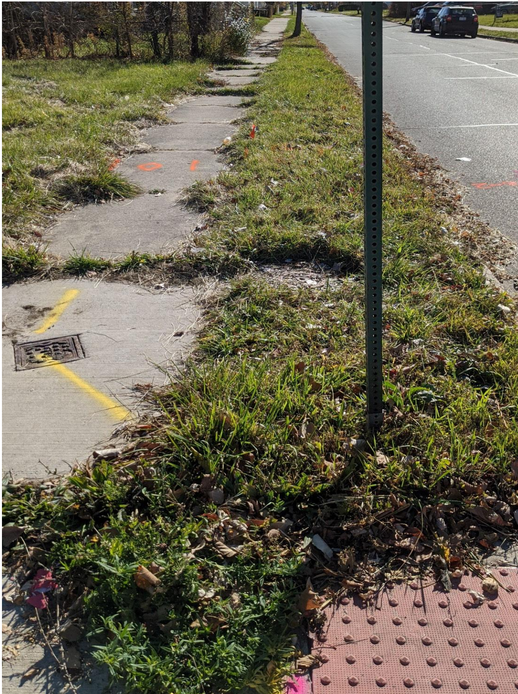
Photograph 7: Gas valve at southeast corner of Freud Street and Conner Street looking south.
