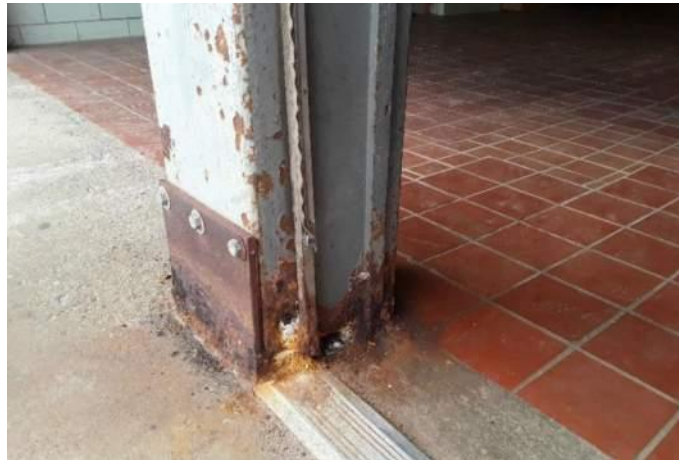
Figure 6: Existing Damaged Column Base
