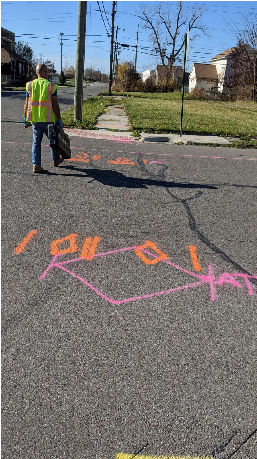
Photograph 4: Communications duct bank crossing Conner Street looking west.
