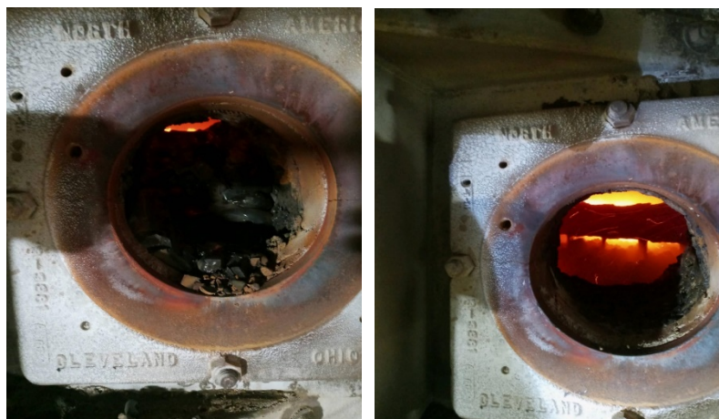
Some burner tunnels were severely impacted by slag and required cleaning. Burners will operate far more efficiently now that the tunnels have been de-slugged.
