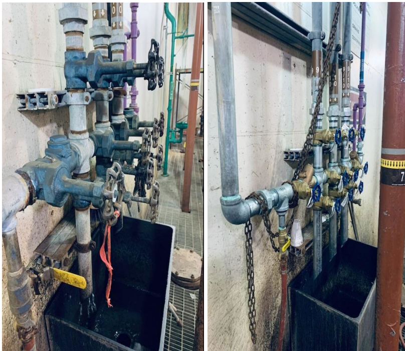
The age of the valves and piping were contributing to frequent leaks and need for repairs. The rebuild should prolong time between repairs minimizing overall downtime.
