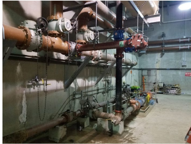
Figure 3: Newly installed piping and valving on residuals lines
