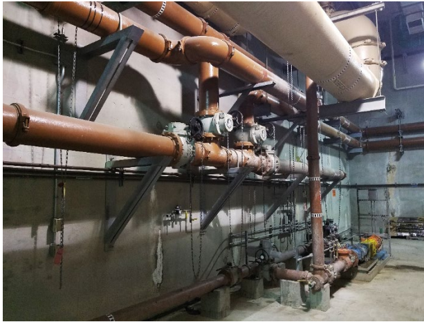
Figure 2: Before condition of residuals transfer piping
