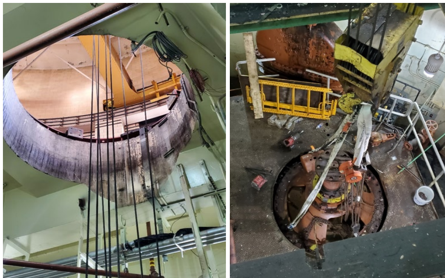
The old pull-out assembly for Main Lift Pump #1 was rigged to the overhead crane in preparation for removal.
