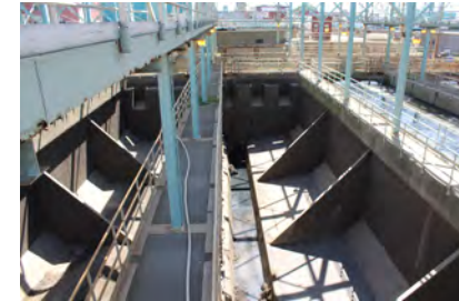
Pump Station 2, Grit channels
