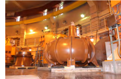
Main Raw Sewage Pumps at Pump Station 2
