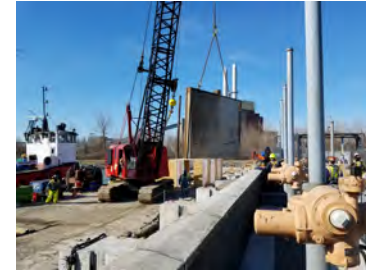
Effluent Relief Gate Repair
