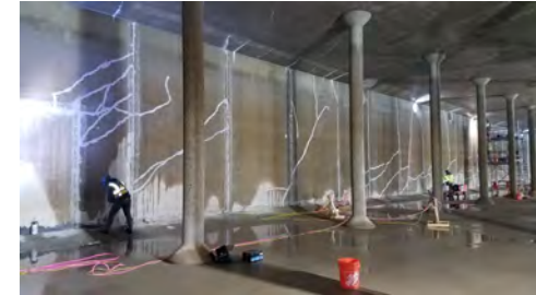
Imlay Booster Station: Sealing interior wall cracks
