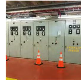
Representative Switchgear to be Replaced under CIP 111001
