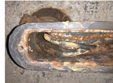
Leaking Conduit in Drain Vault
