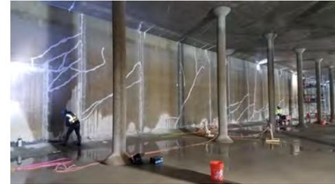
Imlay Booster Station: Sealing interior wall cracks
