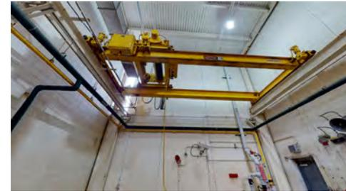
Corroded building crane from failed HVAC system
