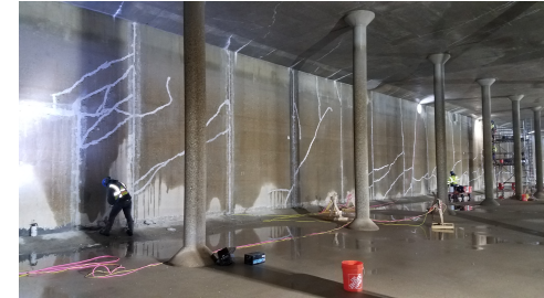
Imlay Booster Station: Sealing interior wall cracks
