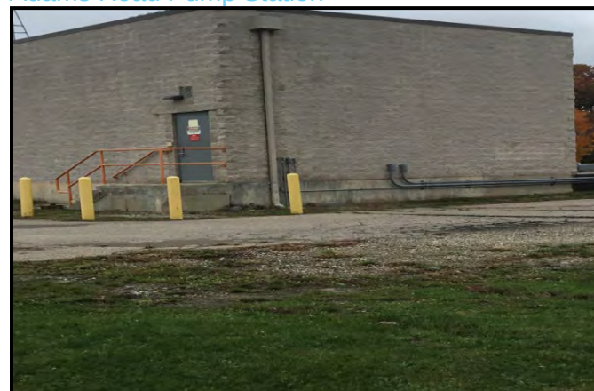
Figure 20. Adams Road Pump Station
