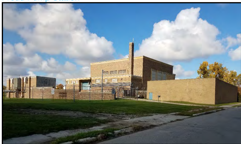
Figure 59. Freud Pump Station
