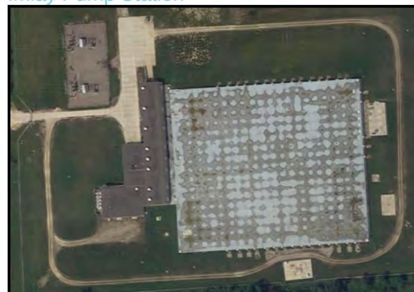
Figure 28. Imlay Pump Station
