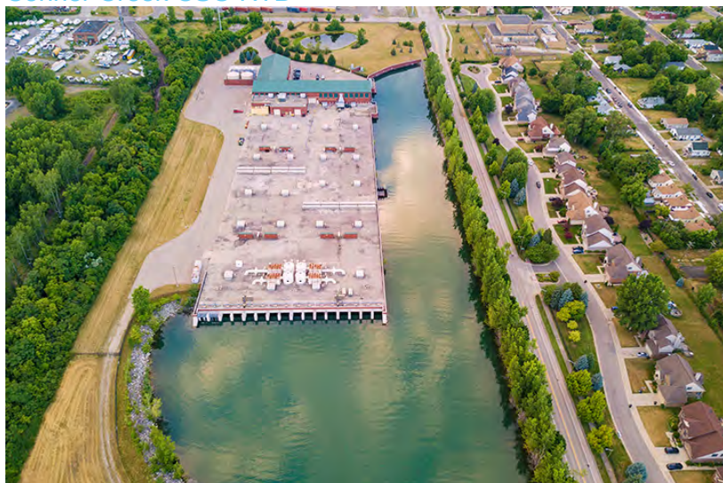
Figure 40. Conner Creek CSO RTB
