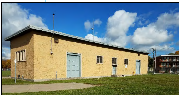
Figure 21. Eastside Pump Station
