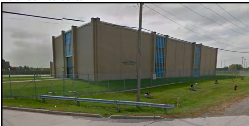
Figure 31. North Service Center
