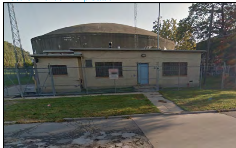
Figure 22. Electric Avenue Pump Station
