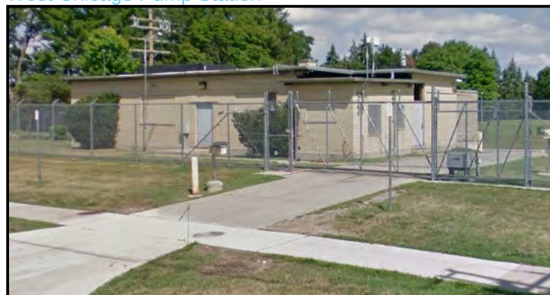
Figure 36. West Chicago Pump Station
