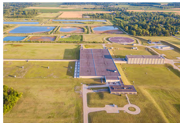
Figure 3. Lake Huron WTP
