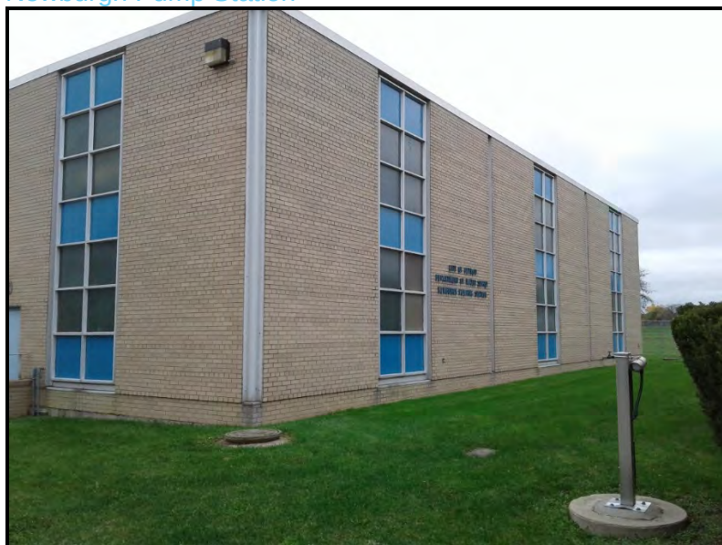
Figure 29. Newburgh Pump Station
