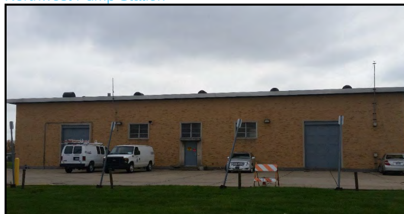
Figure 30. Northwest Pump Station
