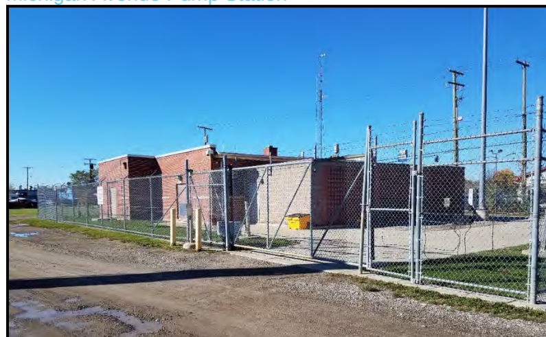
Figure 26. Michigan Avenue Pump Station
