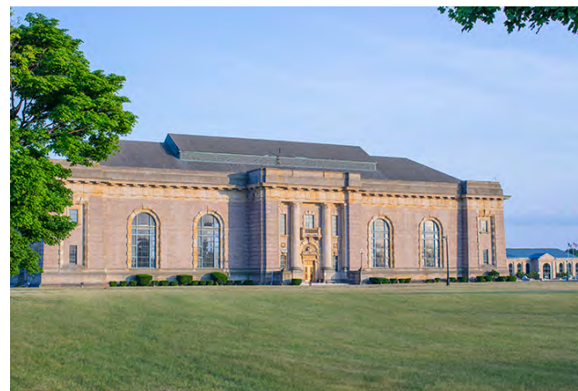
Figure 10. Water Works Park WTP
