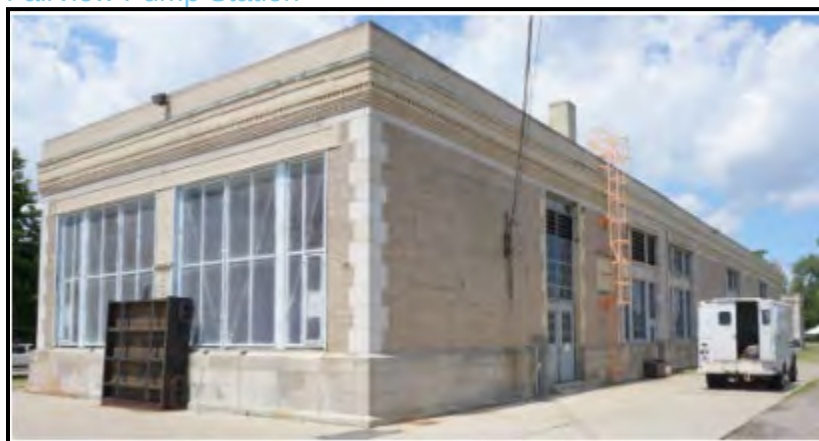
Figure 57. Fairview Pump Station
