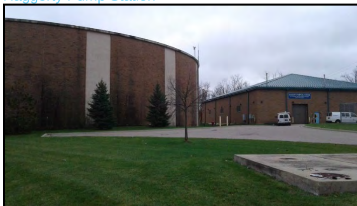
Figure 23. Haggerty Pump Station
