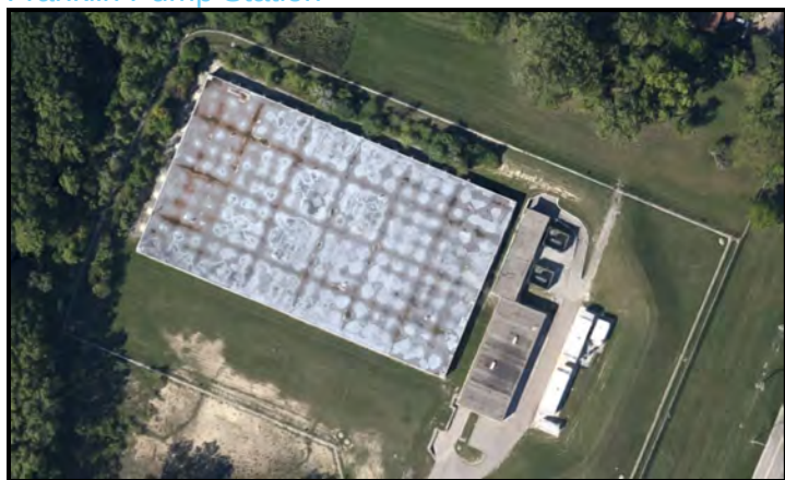
Figure 25. Franklin Pump Station
