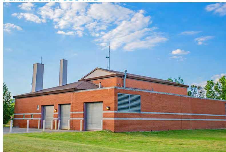
Figure 43. Puritan-Fenkell CSO RTB
