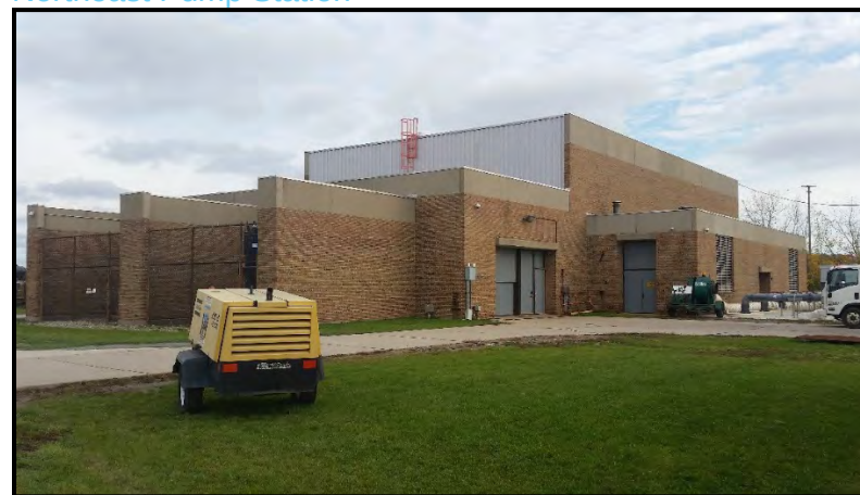
Figure 61. Northeast Pump Station
