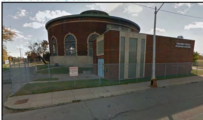
Figure 55. Conner Creek Pump Station
