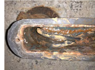
Leaking Conduit in Drain Vault
