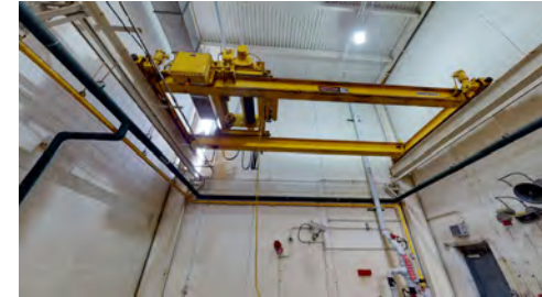
Coroded building crane from failed HVAC system
