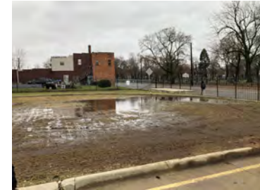
Poor Drainage at Leib
