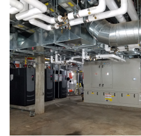
Mechanical Room - New WCHP and Boilers
