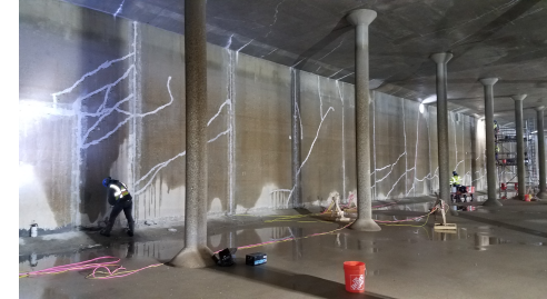
Imlay Booster Station: Sealing interior wall cracks
