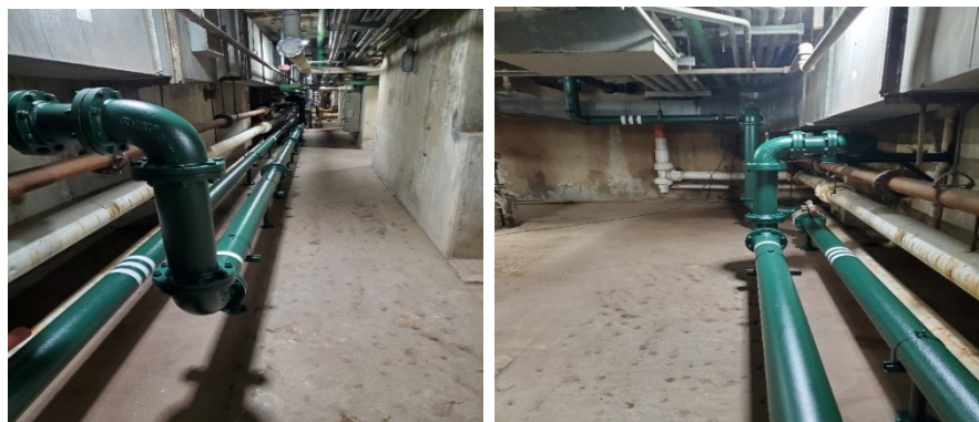
The new secondary water lines installed in the Dewatering Complex 1 basement Also pictured are the old lines that will be removed
