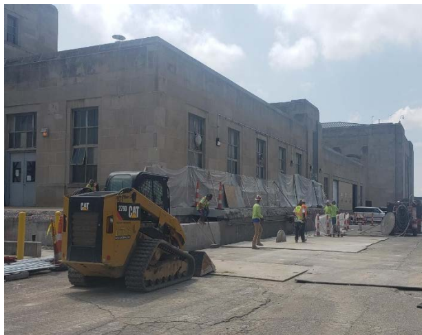
Demolition of existing Loading Dock
