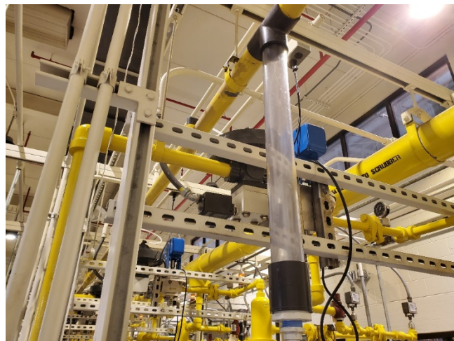
New condensates drain and sight glass on sulfur dioxide scrubber manifold
