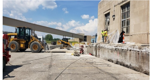
Demolition of Loading Dock
