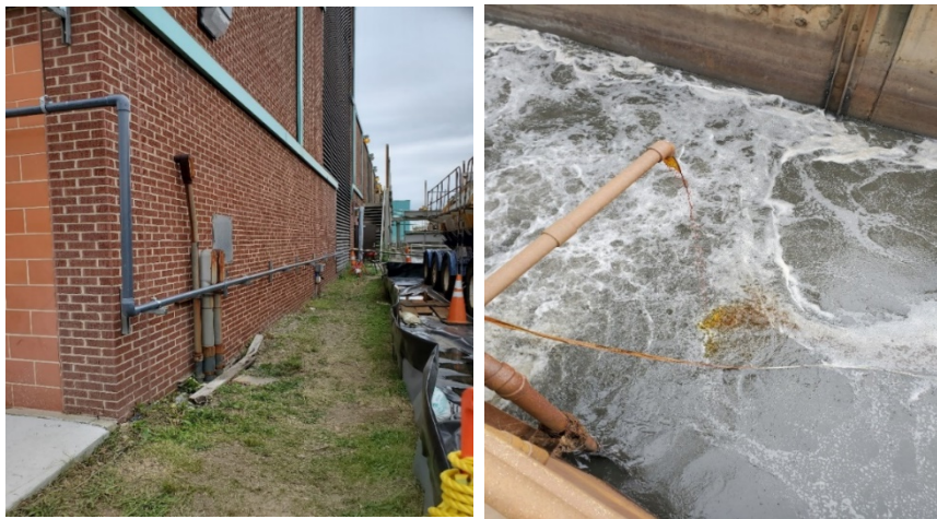
The temporary ferric line routed to the new permanent ferric chloride tanks at Pump Station 2 being tested. These lines will be removed after the completion of the permanent ferric line.
