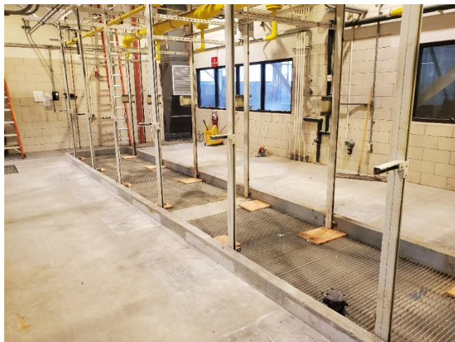
Existing housekeeping pads and wiring removed as a component of selective demolition
