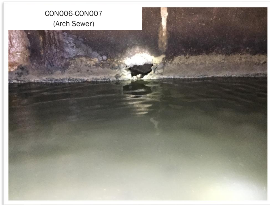
Figure 1-13. Typical Defect - Hole in Sewer Wall
