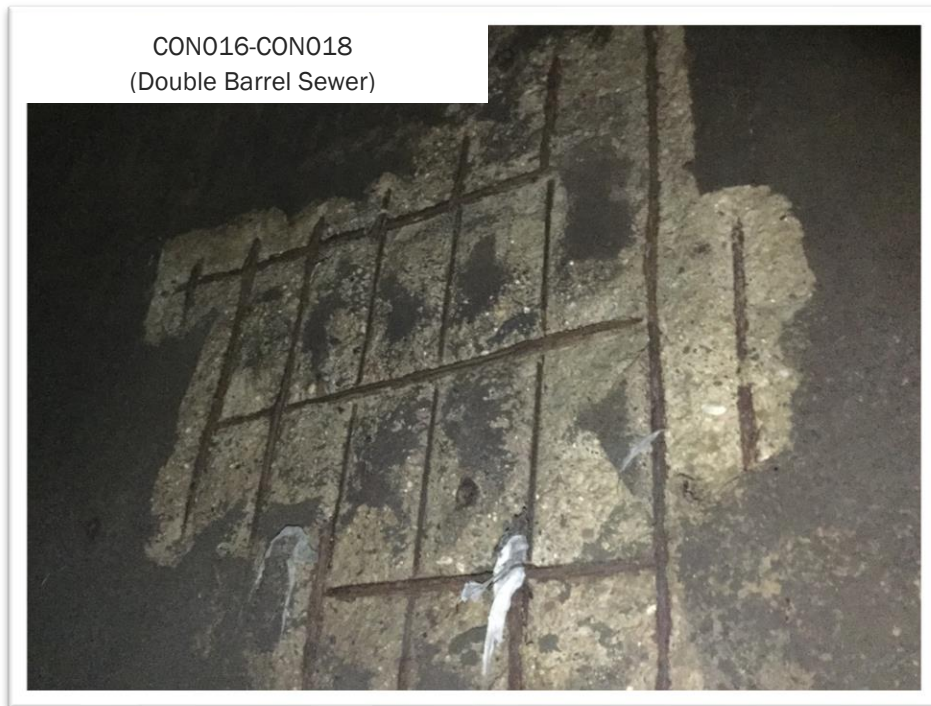
Figure 1-11. Typical Defect - Surface Damage Reinforcement Visible with Spalling
