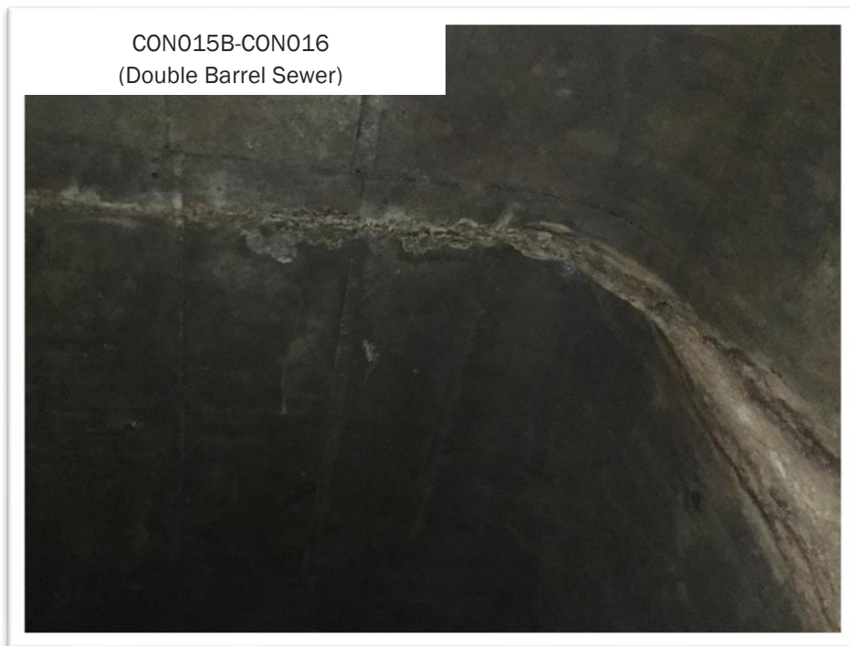
Figure 1-12. Typical Defect - Infiltration Runner
