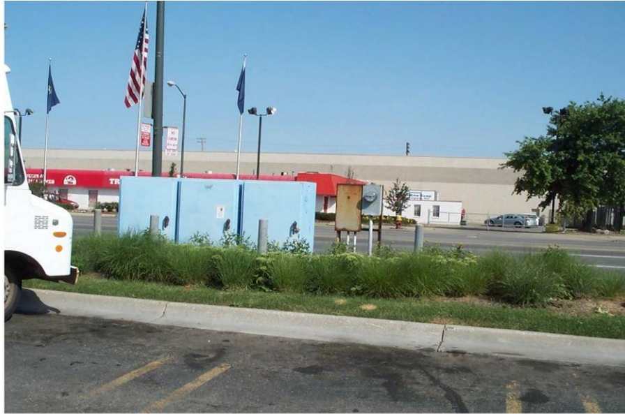
VR-04 Transformer Cabinet, Control Cabinets and Electrical Service Rack Looking North
