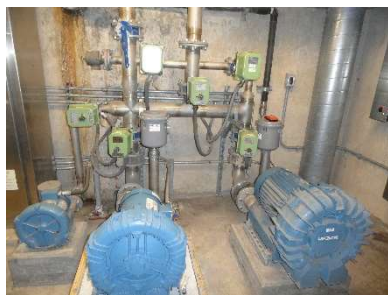
Blower 1 recently replaced
