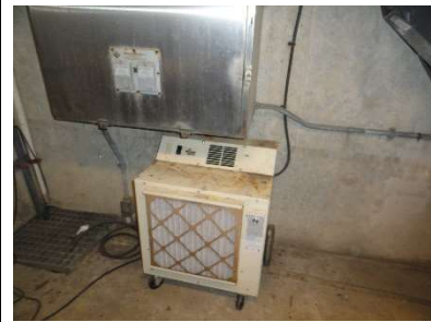
Dehumidifier not working
