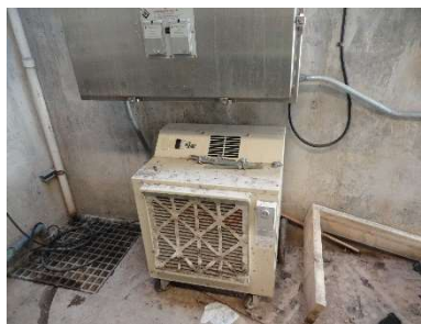
Dehumidifier not working
