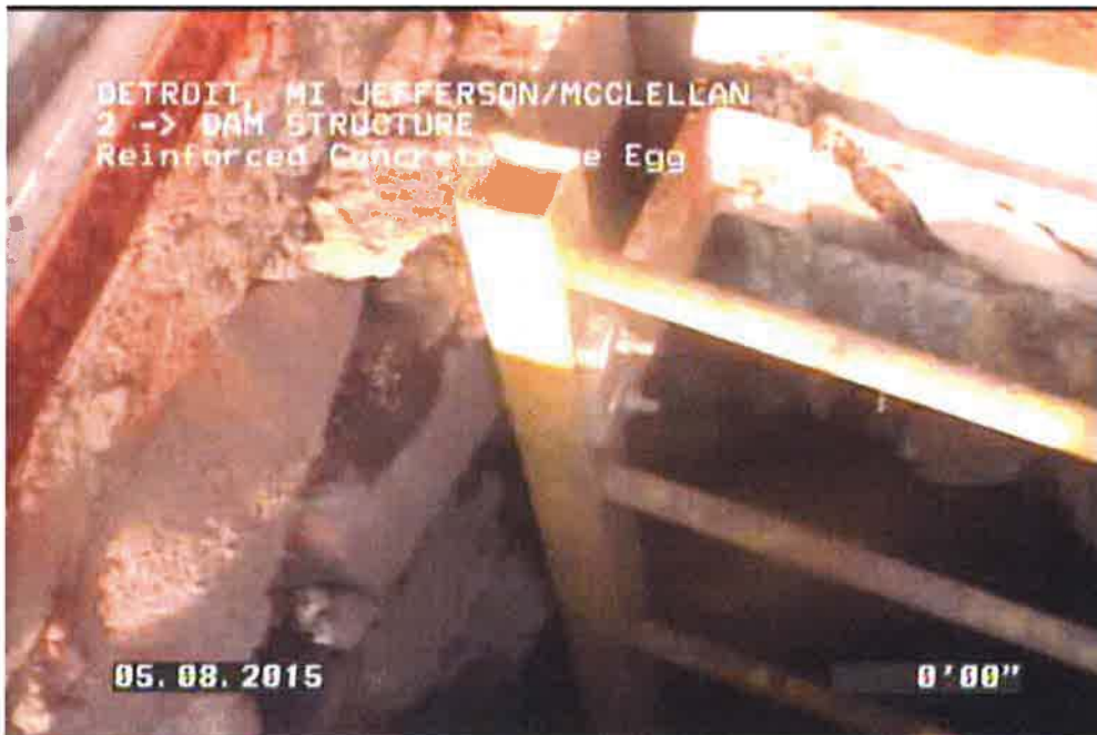
WHAT APPEARS TO BE BRICK, BLOCK, AND BROKEN CONCRETE – THIS HATCH IS LOCATED WITHIN THE SIDEWALK
