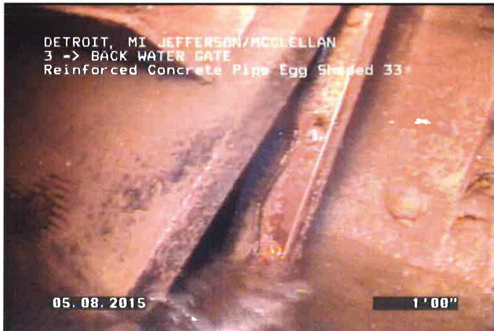
CLOSE-UP VIEW OF RUBBER FLAP ALLOWING FLOW TO PASS THROUGH
