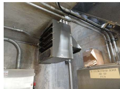
Corrosion on exterior of heater motor
