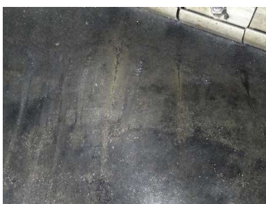
Abrasions in rubber from anchor bolts as dam inflates
