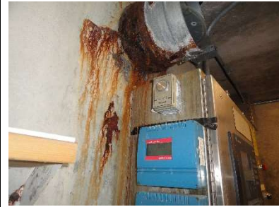
Significant water corrosion due to water leaks
