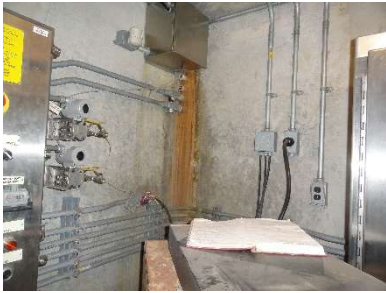
Slight water leaks through control vault pipes
