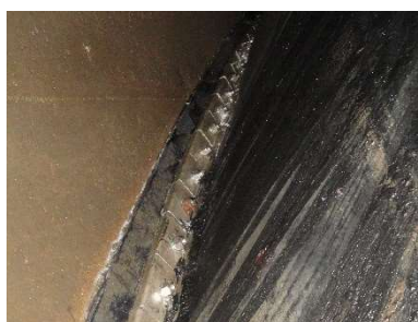
Corroded anchor bolts
