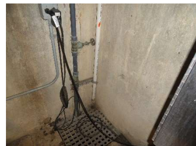
Sump pump is working
