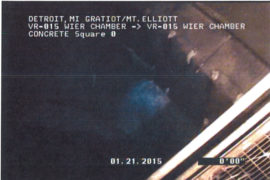
Leakage under weir segment is minimal but should be sealed
