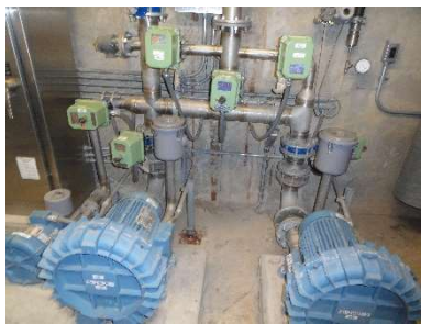
All blower and vacuum equipment working
