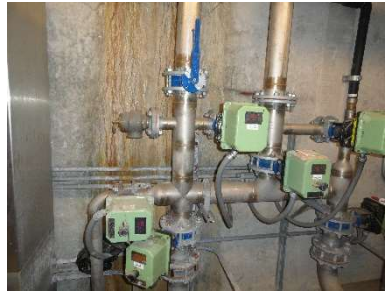
Water leaks along control vault walls
