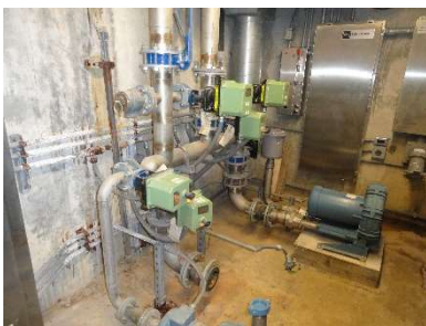
Blower No. 1 is missing
