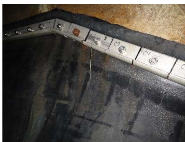
Corroded anchor bolts
