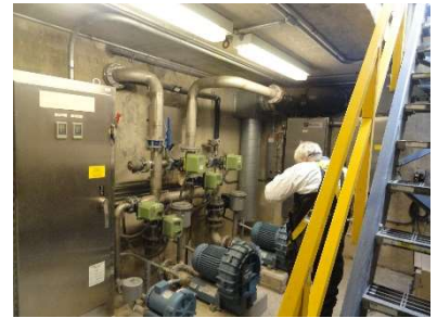
Vault appears to be in good condition
