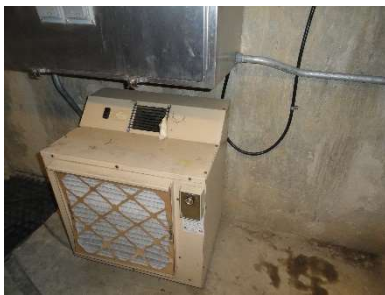
Dehumidifier is working, but the heater is not
