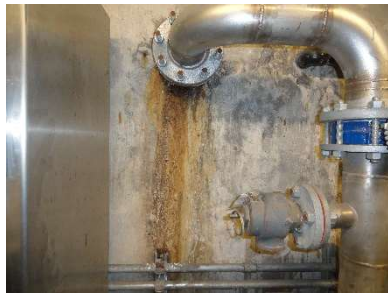
Slight leaks in the control vault
