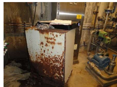
Old UPS cabinet is corroded and no longer used
