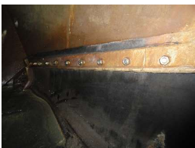
Stalagmites collecting on anchor bolts
