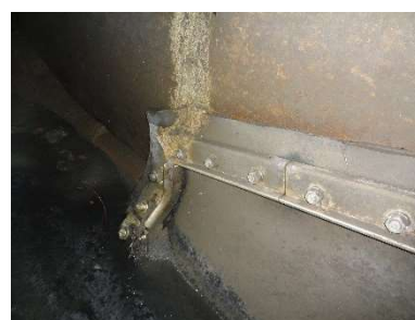
Small amount of stalagmites over anchor bolts
