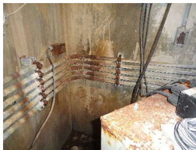
Conduits below leak are corroded and falling apart
