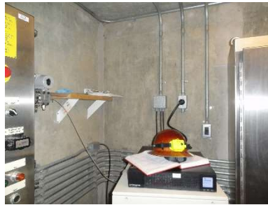
Conduits are in good condition
