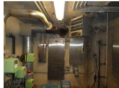
Besides leaks, control vault in good condition
