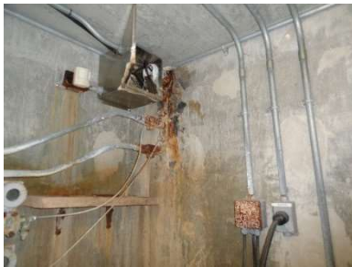
Leak through 4-inch pipe in top corner of chamber
