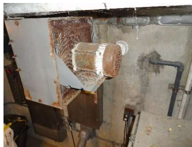
Heater not working and corroded
