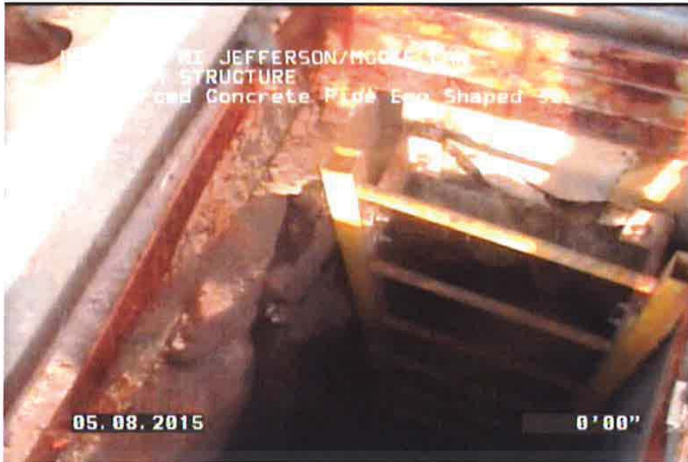
ACCESS HATCH TO DIVERSION STRUCTURE – CONCRETE IS IN NEED OF REPAIR
