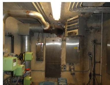
Heater, ventilation system and dehumidifier not working
