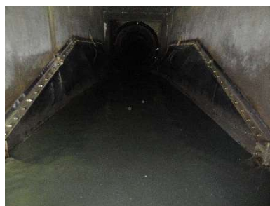
Dam material appears to be in good condition
