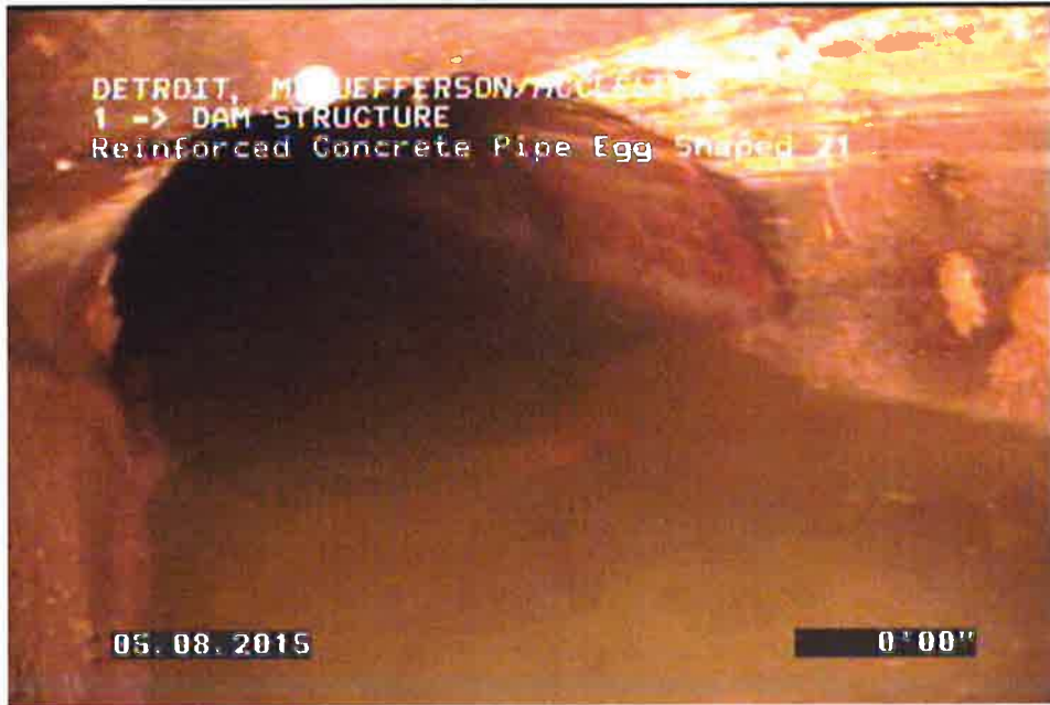
2'-9" EGG SEWER WITH DRY WEATHER FLOW GOING FROM CADILLAC DIVERSION CHAMBER TO THE McCLELLAN DIVERSION CHAMBER
