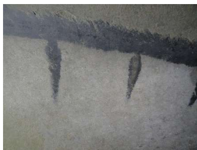
Minor abrasions found in dam material
