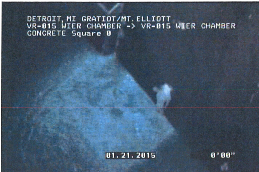
Leakage under weir segment is minimal but should be sealed
