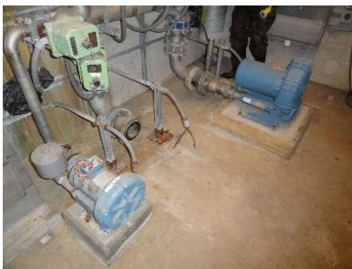
Vacuum pump disconnected and blower 1 is missing
