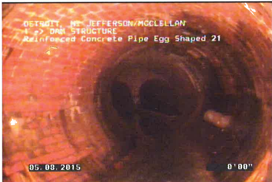
5'-9" CADILLAC SEWER DOWNSTREAM OF DAM TRANSITIONING TO TWO 60" SEWERS UNDER PARKVIEW AVE TO DETROIT RIVER (STORM FLOW)
