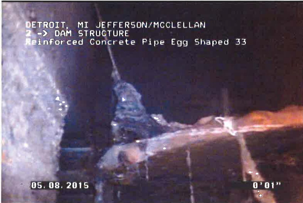
CABLE ATTACHED TO FLAP VALVE
