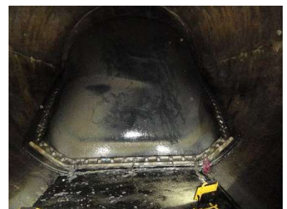
No air leaks observed on downstream side of dam
