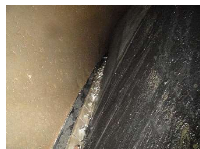
Slight air leaks along the side edges of dam
