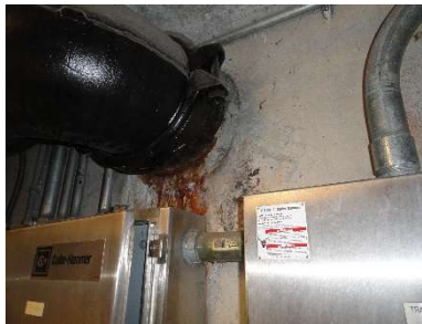
Slight leaks in the control vault
