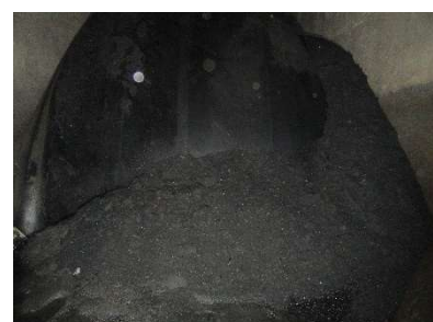
Significant silt on dam and air leaks along edges of dam
