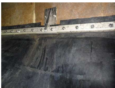
Rubber appears to be in good condition
