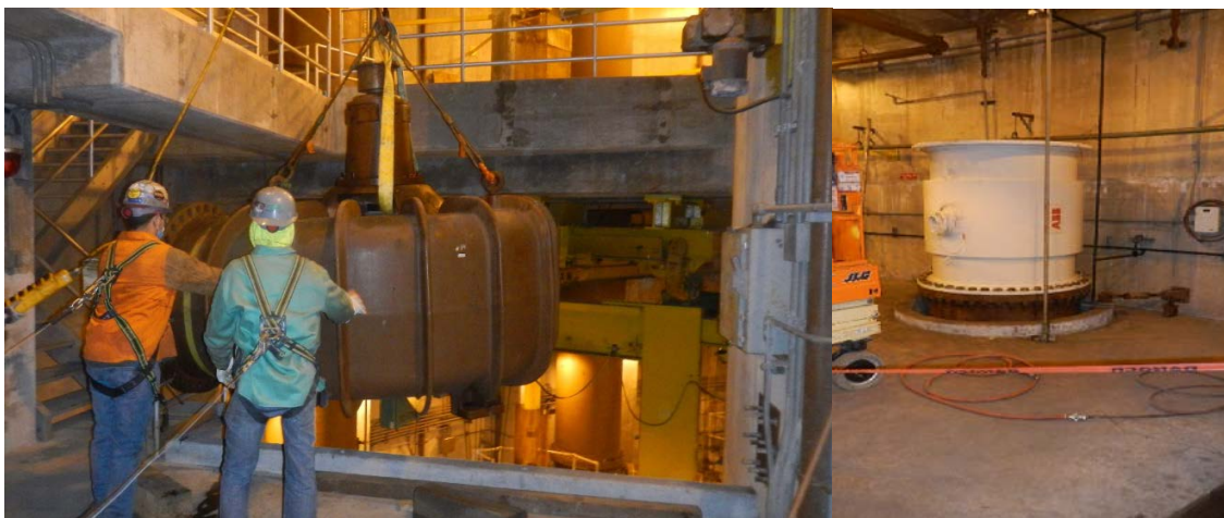
Removal of old pump No. 14 and installation of a new flowmeter on pump # 14 discharge
