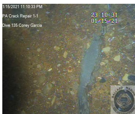
Pennsylvania Crack Repair-After Injection
