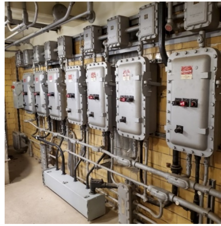
Starter panels for clarifiers (Typical of 12 clarifiers)
