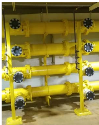
Pipelines for Sulphur Dioxide Solution water
