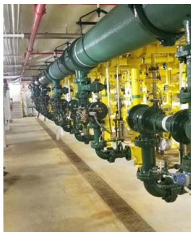
Sulphur Dioxide Injectors
