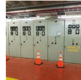
Representative Switchgear to be Replaced under CIP 111001
