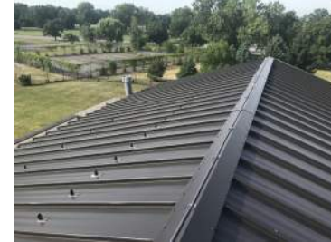
New Metal Roof
