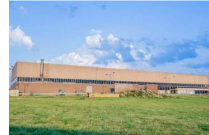
SW SCADA System Upgrade
