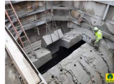
DRI Shaft Construction
