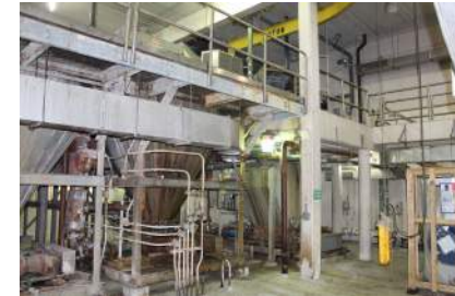
Primary Circular Scum House, Inside
