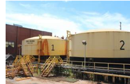
Ferric Chloride Storage and Containment Area
