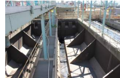
Pump Station 2, Grit channels
