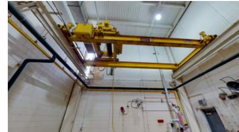
Corroded building crane from failed HVAC system
