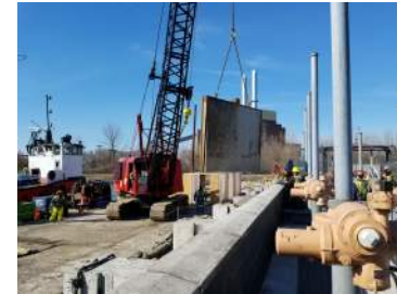
Effluent Relief Gate Repair
