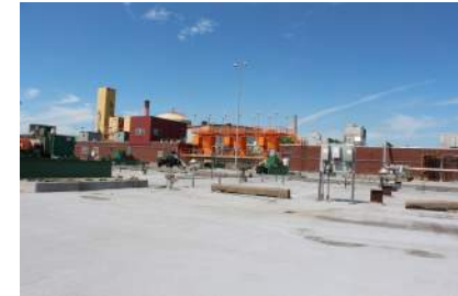
Aeration Basin 4, and ILP's 3, 4, and 7
