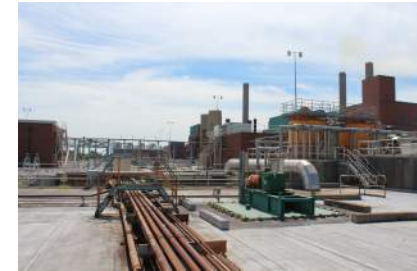
Aeration Basin 1 and ILP's 1 and 2
