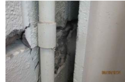
Existing Structural Condition
