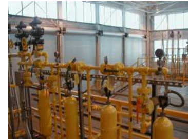
Chlorination Building, Inside
