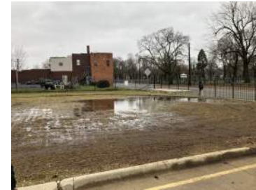
Poor Drainage at Leib
