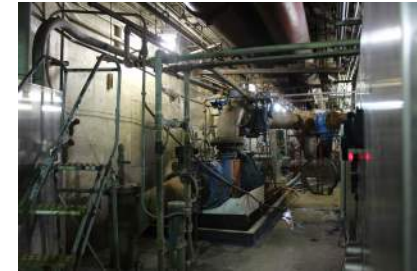
Sludge Feed pump in Complex A
