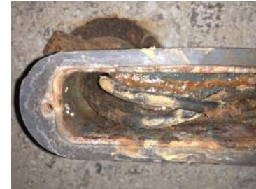
Leaking Conduit in Drain Vault
