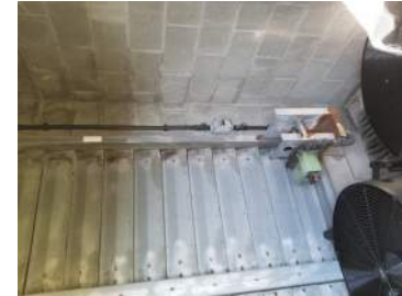
Leib HVAC - Frozen Dampers
