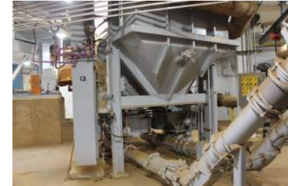
Incineration Complex II, Ash System
