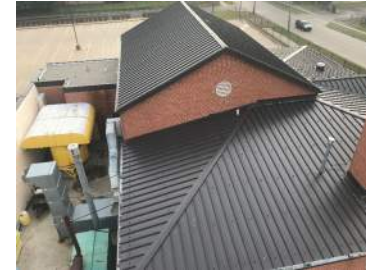
New metal roof
