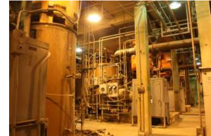
SFE Building, Basement
