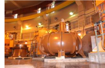
Main Raw Sewage Pumps at Pump Station 2
