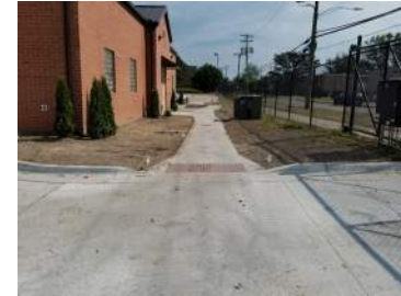
New Parking Lot and Hatch Work
