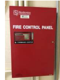
Seven Mile Failed and Outdated Fire Panel
