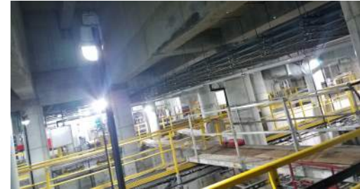
Leib Electrical Improvements
