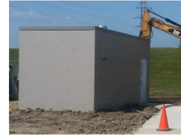
New staircase well access to Tunnel
