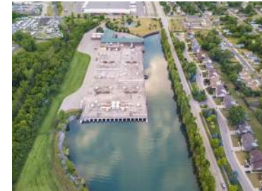
Conner Creek CSO Facility
