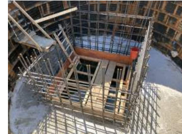
Phase IV construction at Outfall B-19
