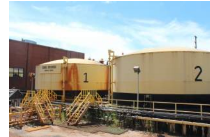
Ferric Chloride Storage and Containment Area
