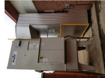
New Air Handling Unit
