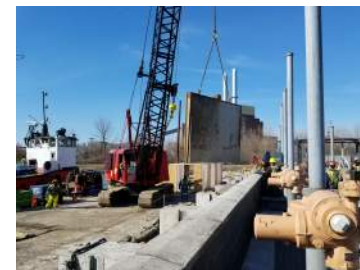
Effluent Relief Gate Repair
