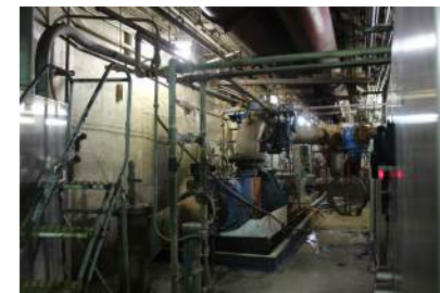
Sludge Feed pump in Complex A
