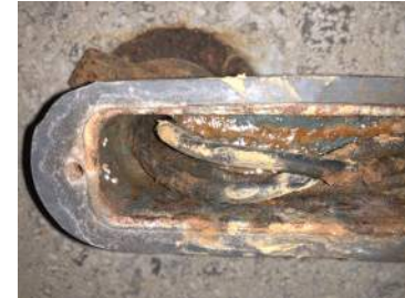
Leaking Conduit in Drain Vault
