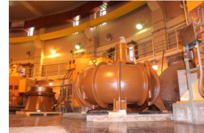
Main Raw Sewage Pumps at Pump Station 2
