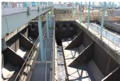
Pump Station 2, Grit channels
