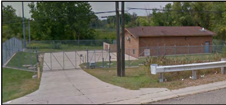
Figure 32. Orion Pump Station
