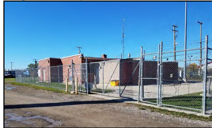
Figure 26. Michigan Avenue Pump Station
