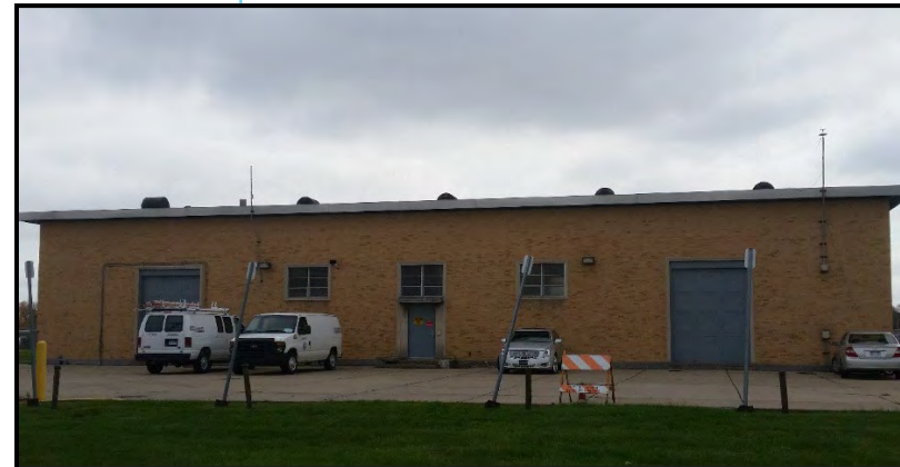
Figure 30. Northwest Pump Station
