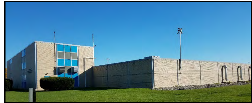
Figure 24. Ford Road Pump Station
