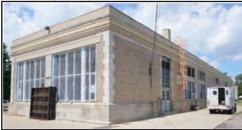
Figure 57. Fairview Pump Station
