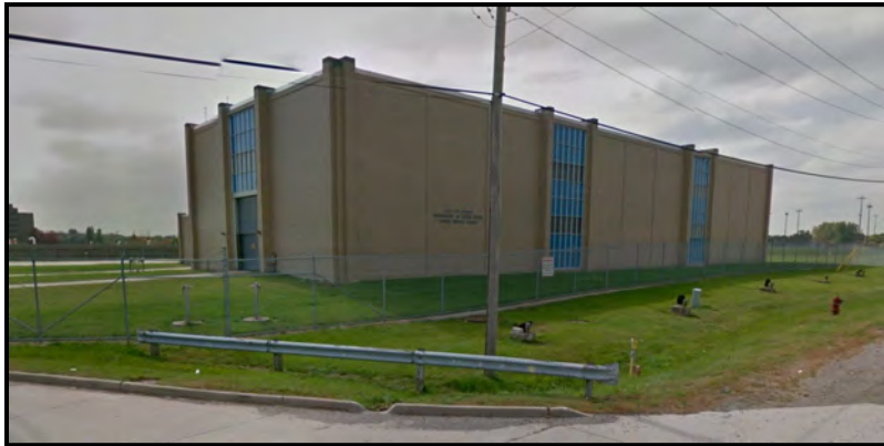
Figure 31. North Service Center
