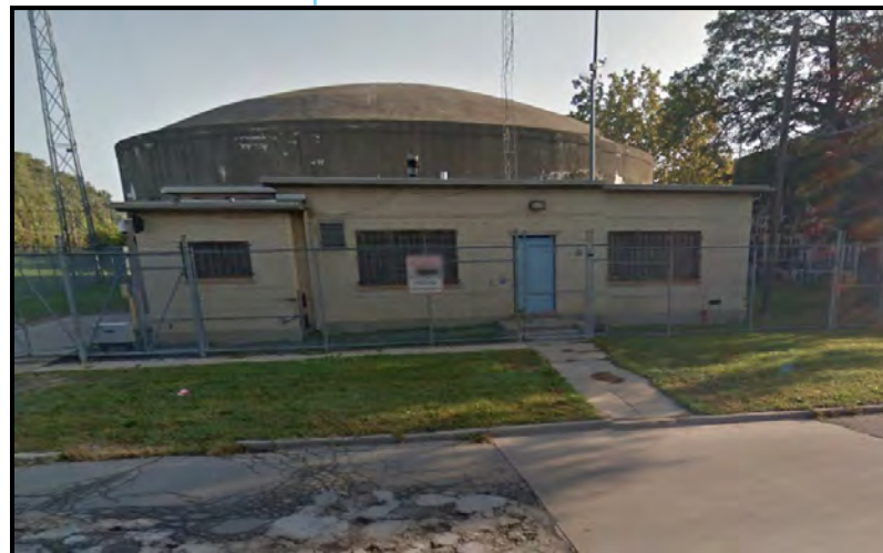
Figure 22. Electric Avenue Pump Station
