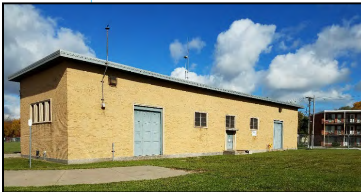
Figure 21. Eastside Pump Station
