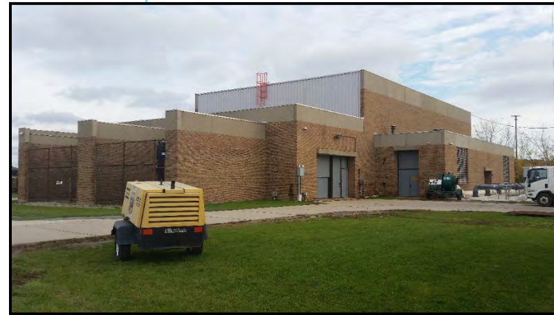
Figure 61. Northeast Pump Station
