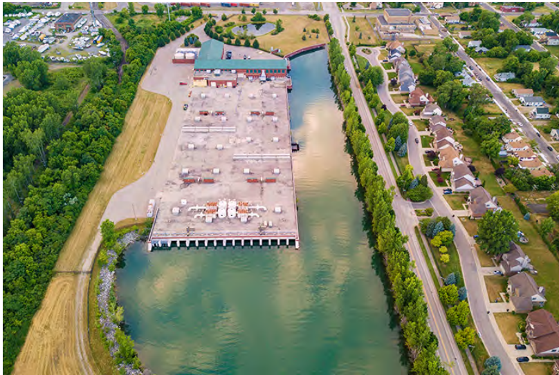
Figure 40. Conner Creek CSO RTB
