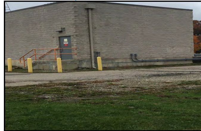
Figure 20. Adams Road Pump Station
