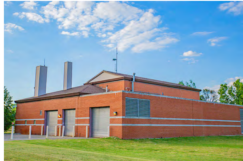
Figure 43. Puritan-Fenkell CSO RTB
