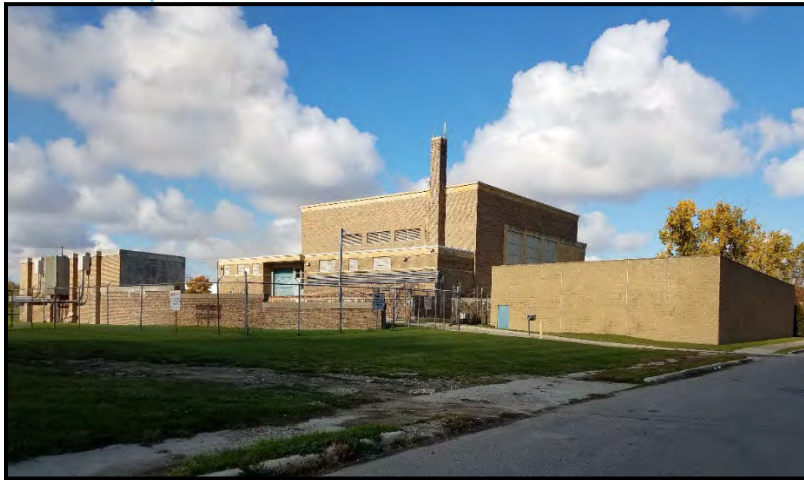
Figure 59. Freud Pump Station
