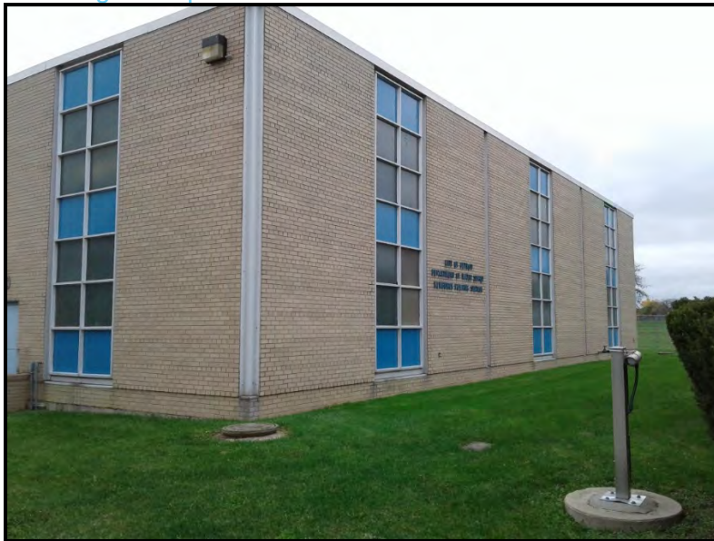
Figure 29. Newburgh Pump Station
