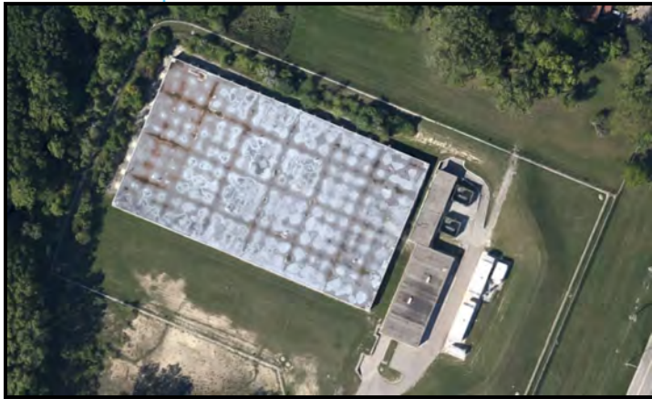
Figure 25. Franklin Pump Station
