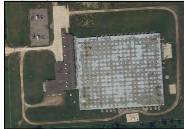
Figure 28. Imlay Pump Station
