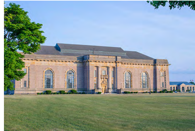
Figure 10. Water Works Park WTP
