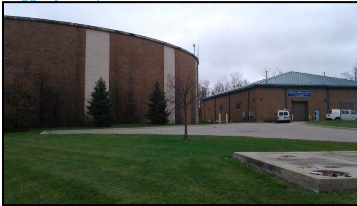
Figure 23. Haggerty Pump Station
