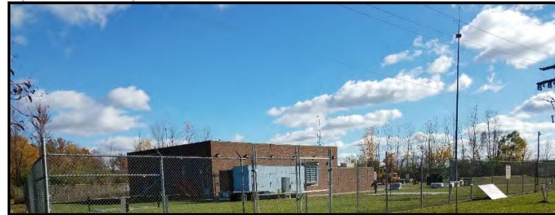
Figure 38. Ypsilanti Pump Station
