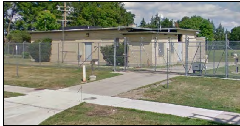
Figure 36. West Chicago Pump Station
