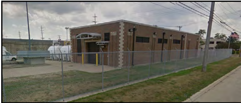
Figure 35. Schoolcraft Pump Station
