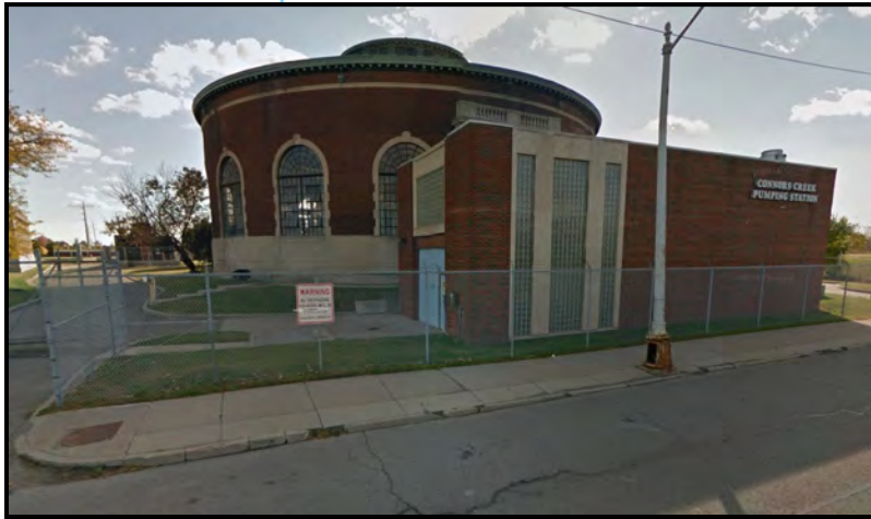
Figure 55. Conner Creek Pump Station
