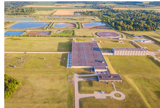
Figure 3. Lake Huron WTP
