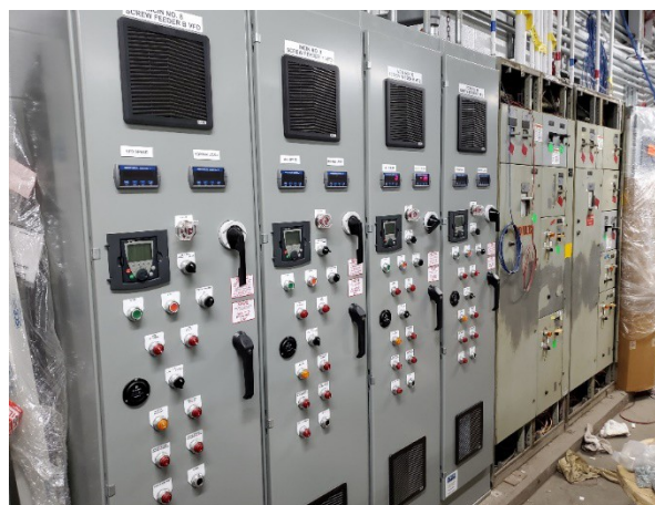
Newly installed and commissioned screw conveyor VFDs
