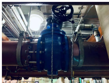
Newly installed SFE isolation plug valve
