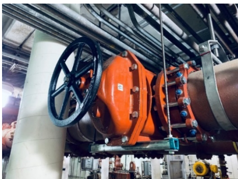
Newly installed SFE isolation gate valve
