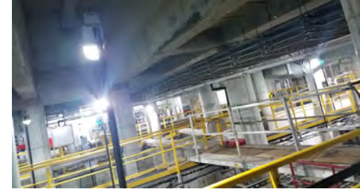
Leib Electrical Improvements
