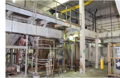
Primary Circular Scum House, Inside
