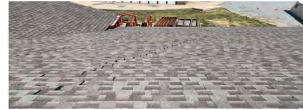
• The previous installment on roof area 2 also failed to follow the required "step-down" installation method. As seen in the picture above, the shingle seams fall >4" from each other. This is a very common mistake found on
