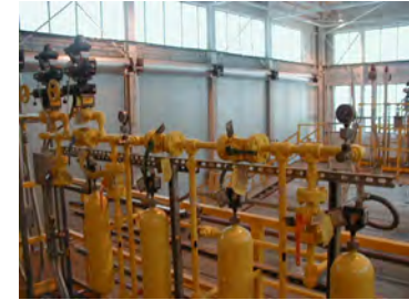
Chlorination Building, Inside
