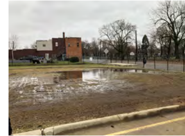
Poor Drainage at Leib
