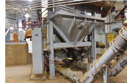
Incineration Complex II, Ash System
