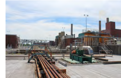
Aeration Basin 1 and ILP's 1 and 2
