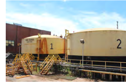
Ferric Chloride Storage and Containment Area
