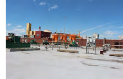
Aeration Basin 4, and ILP's 3, 4, and 7
