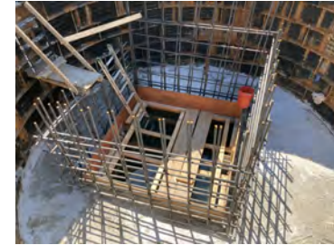
Phase IV construction at Outfall B-19
