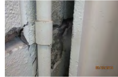
Existing Structural Condition
