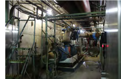
Sludge Feed pump in Complex A
