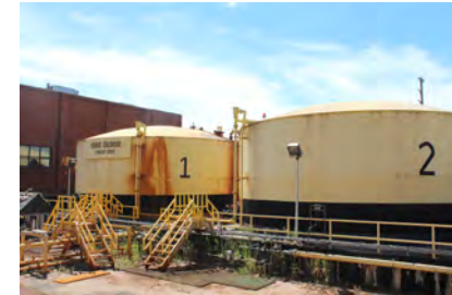
Ferric Chloride Storage and Containment Area
