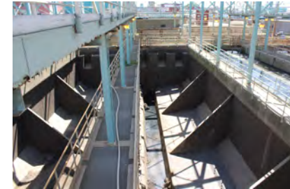
Pump Station 2, Grit channels
