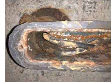
Leaking Conduit in Drain Vault
