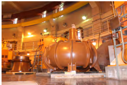
Main Raw Sewage Pumps at Pump Station 2
