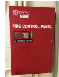
Seven Mile Failed and Outdated Fire Panel
