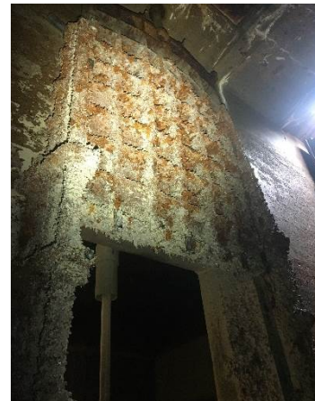
View from the other side of the wall showing the sluice gate in the open position.
