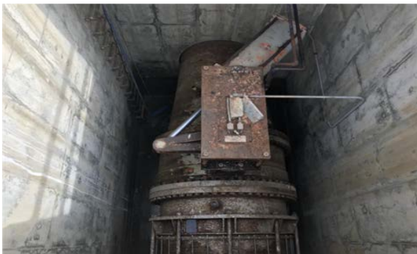
Visual of Valve V-6 to be removed and replaced as part of ESR-015 (R1)
