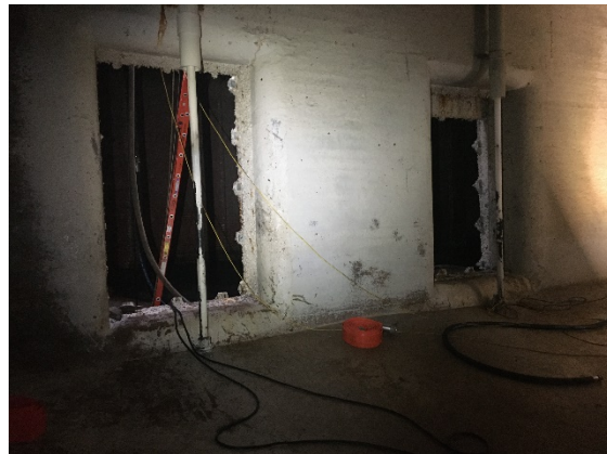
A view inside the 1930 Mixing Chamber Shown are the injection points for PAC
