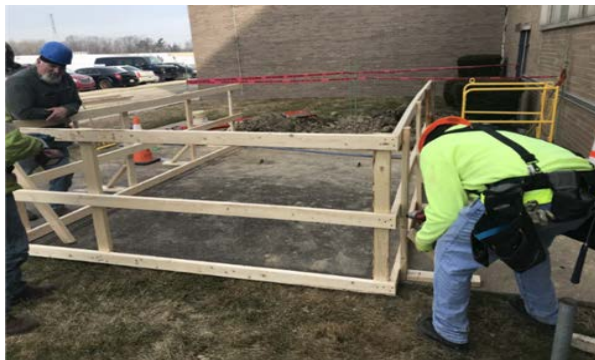
Temporary safety support railing built around V-6 vault opening
