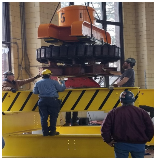
Placing the main lift pump motor #5 rotor into a support stand
