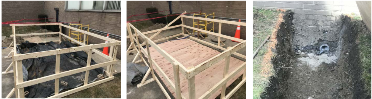
From left to right: Vault for V-6 covered with tarped to protect from elements; Vault for V-6 covered with plywood to protect from elements; and Core at the wall foundation (e.g. V-6 electrical service entrance conduit)
