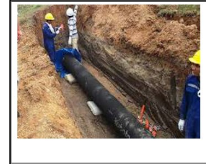
Water main being installed
