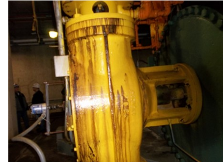
Oil hydraulic valve actuators leaking oil
