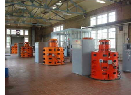
Sanitary pumps at Fairview Pumping Station
