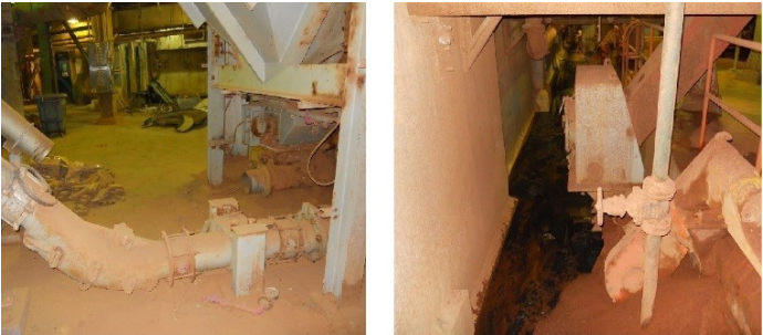
Ash crusher system was last rehabilitated 15 years ago and near the end of its useful life, due to Complex I decommissioning dry ash system needs to be reconfigured and rehabilitated
