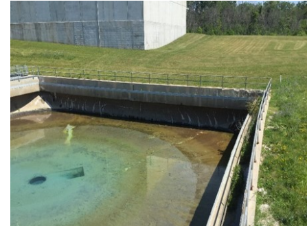
Raw sludge clarifier at Lake Huron WTP
