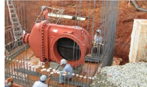
A large valve for a transmission pipe
