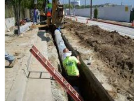
Water main being replaced
