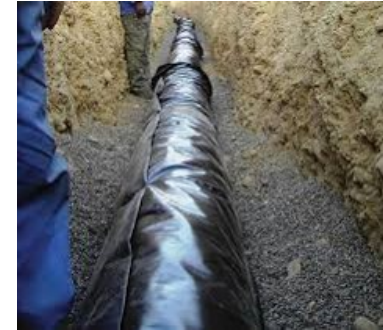
Water main being laid
