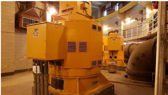
Main Raw Sewage Pumps at Pump Station 2
