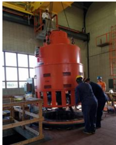
Attaching motor to pump
