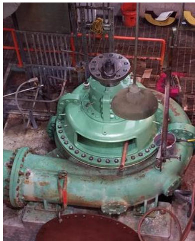
Pump insert now in place
