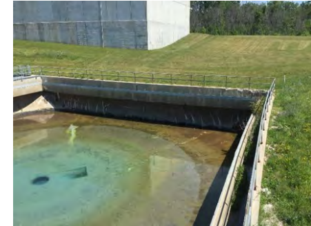
Raw sludge clarifier at Lake Huron WTP
