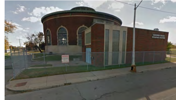
Freud Pump Station
