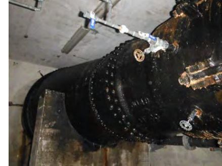
Water production flow metering device
