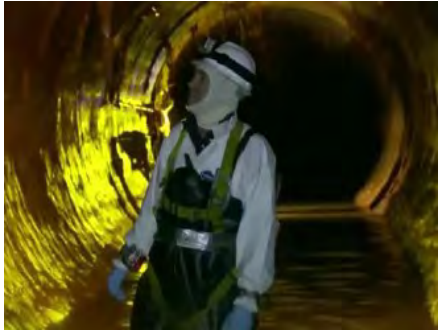
Example inspection of a large sewer
