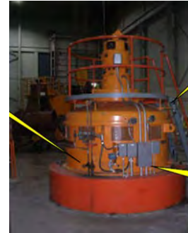
Pump at the Northeast Pumping Station
