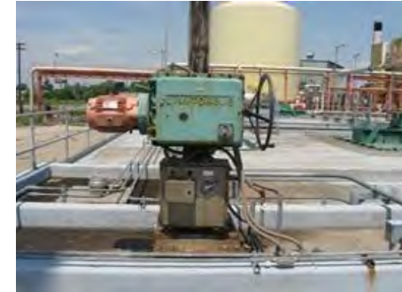
Equipment for aeration system
