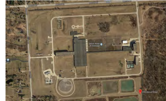
Lake Huron WTP Electrical Tunnel
