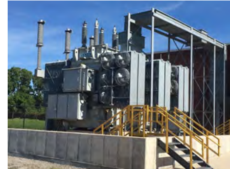
The new 3rd 120/13.8 kV Transformer installed and owned by the Great Lakes Water Authority waiting for the 3rd Primary Electric Feed Line to be installed and energized
