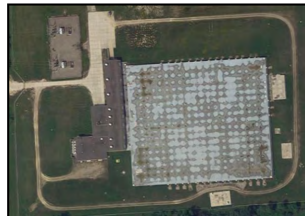
Figure VI-28. Imlay Pump Station
