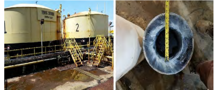
Ferric Chloride Tanks at Pump Station 1
