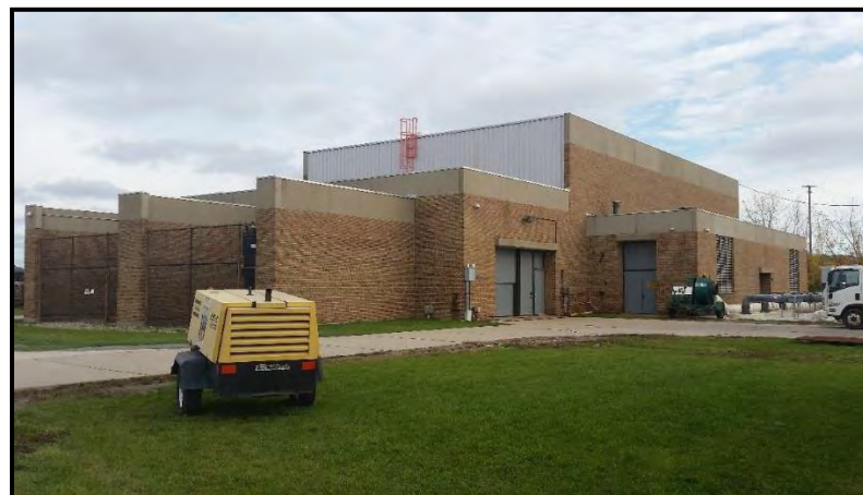
Figure VI-61. Northeast Pump Station
