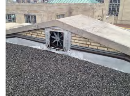
Filter Building roof
