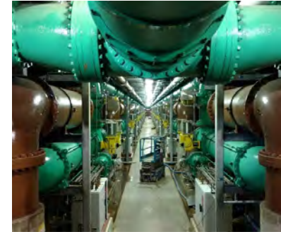
SP-563 – Rehabilitated 1958 Pipe Gallery (in progress)
