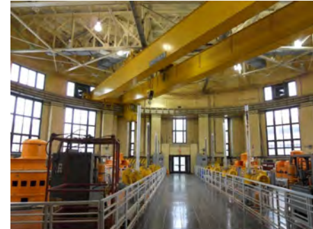
Pump Station 1 Interior
