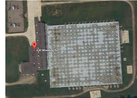
Imlay Pump Station
