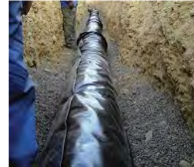
Water main being laid
