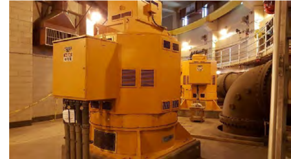
Main Raw Sewage Pumps at Pump Station 2
