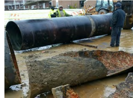
Water main replacement
