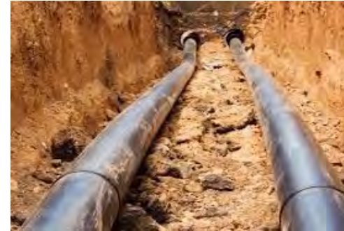
Example of pipe being laid
