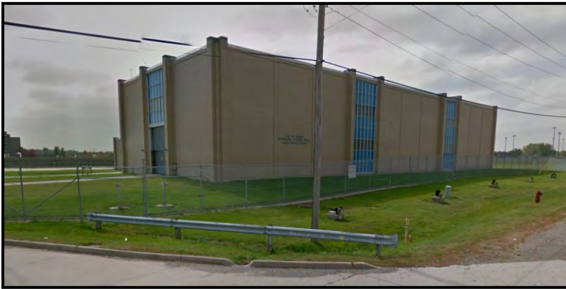
Figure VI-31. North Service Center
