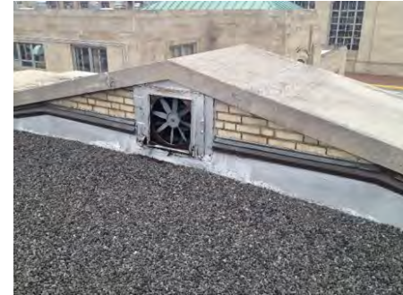
Roof in need of repair
