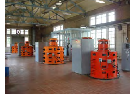
Sanitary pumps at Fairview Pumping Station
