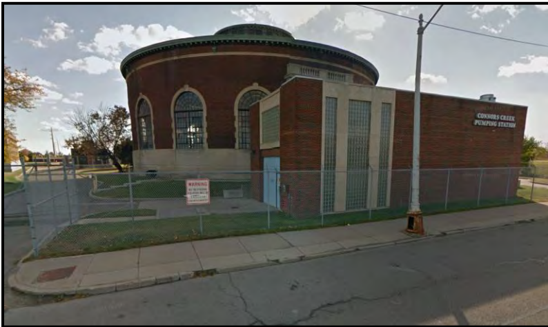
Figure VI-55. Conner Creek Pump Station
