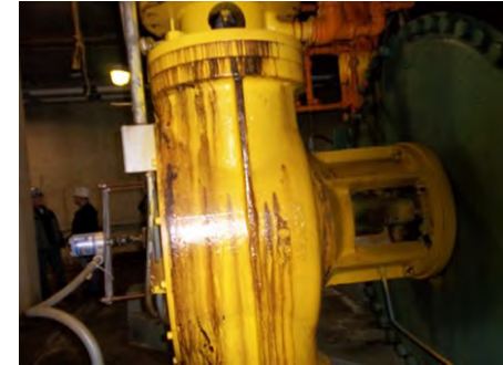
Oil hydraulic valve actuators leaking oil
