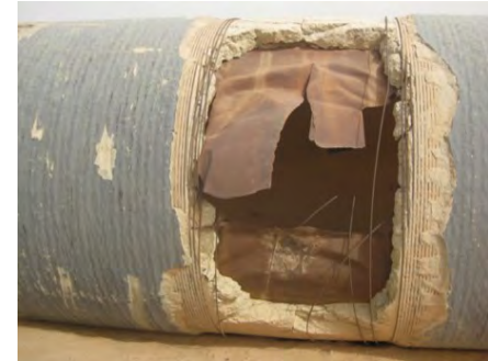
Example of a failed water main
