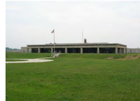
Lake Huron Water Treatment Plant
