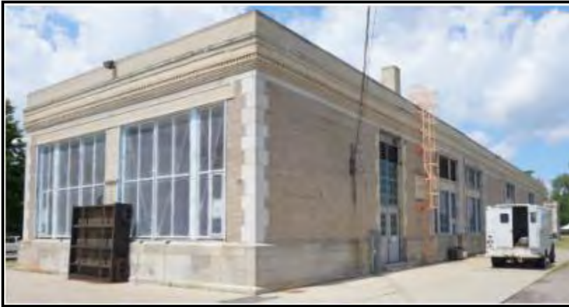
Figure VI-57. Fairview Pump Station
