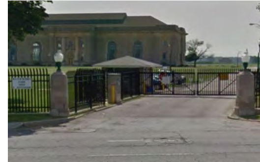
Water Works Park
