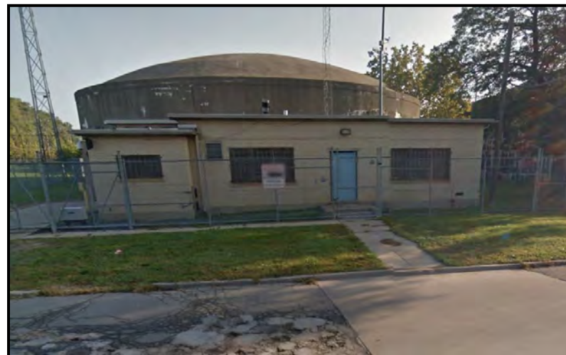
Figure VI-22. Electric Avenue Pump Station
