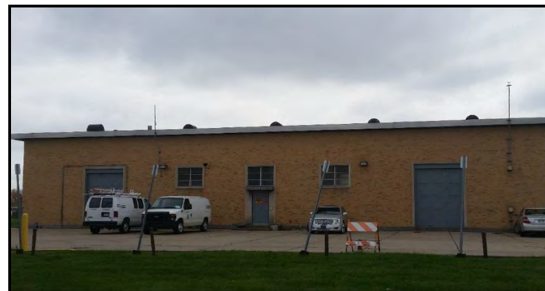
Figure VI-30. Northwest Pump Station
