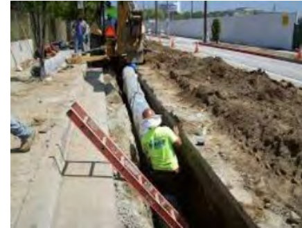
Water main being replaced
