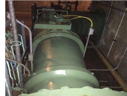
Raw Water Flow Meter
