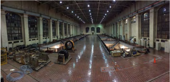
High Lift Station showing high lift pump pits and windows to be replaced.
