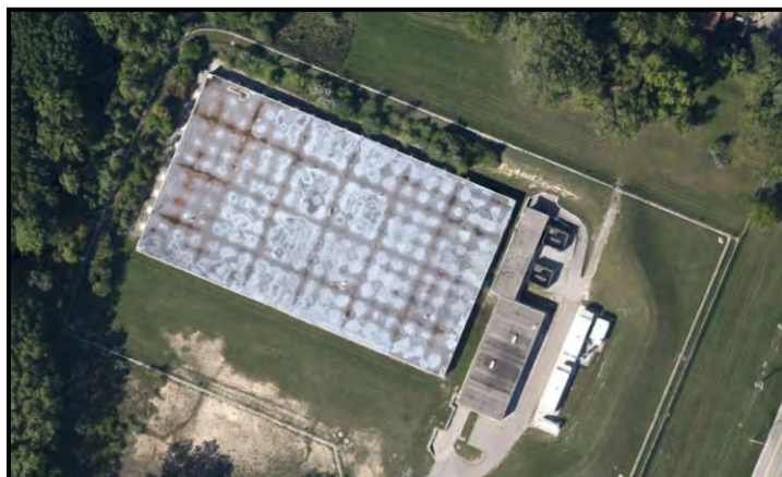
Figure VI-25. Franklin Pump Station
