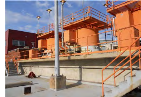
Intermediate Lift Pump Station N.2
