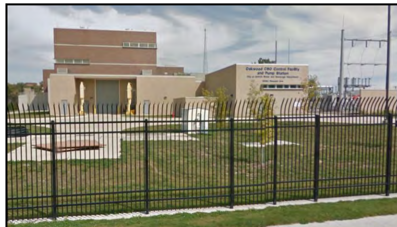
Figure VI-62. Oakwood Pump Station
