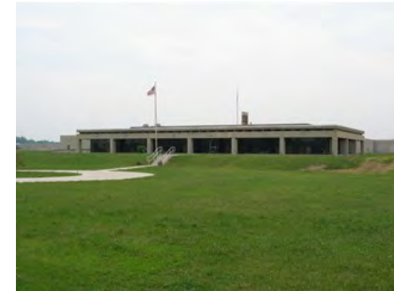
Lake Huron Water Treatment Plant
