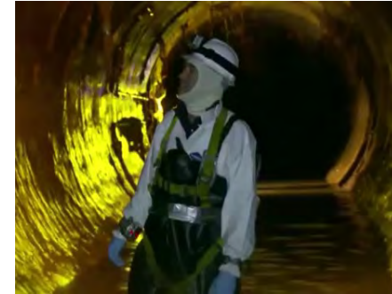
Visual inspection of a large sewer
