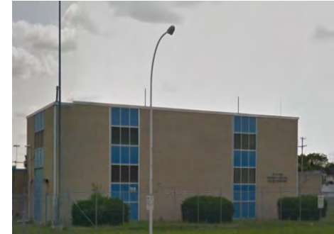
Ford Road Booster Pumping Station
