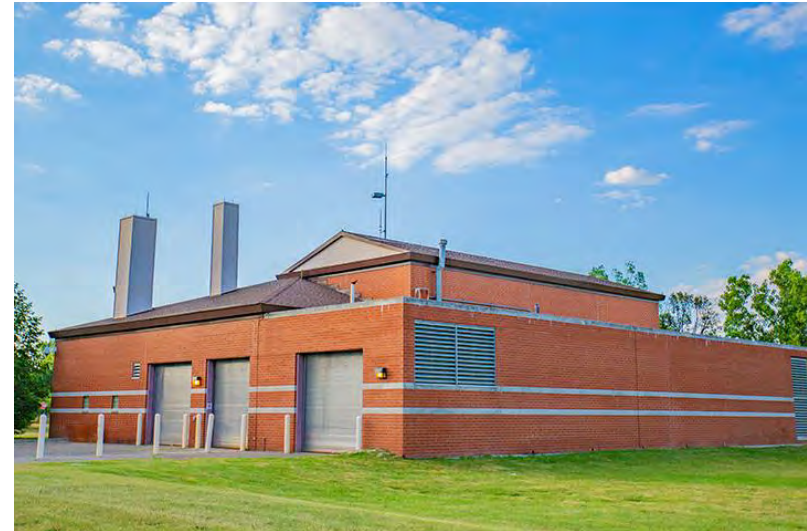
Figure VI-43. Puritan-Fenkell CSO RTB
