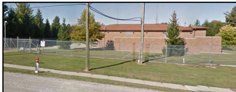
Figure VI-33. Rochester Pump Station
