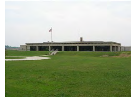
Lake Huron Water Treatment Plant
