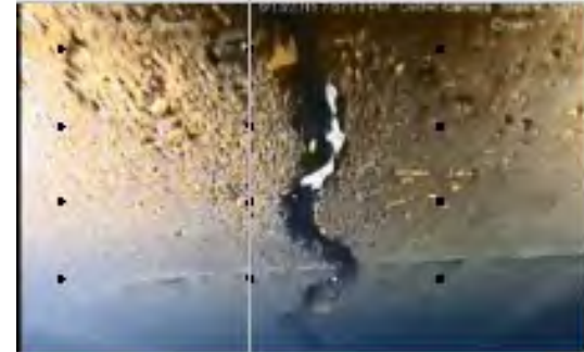
Crown cracks are especially concerning in the Springwells Raw Water Tunnel
