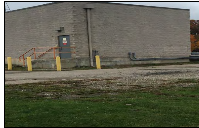
Figure VI-20. Adams Road Pump Station
