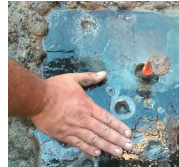
Springwells WTP - Pipe Main - Note the wood plug.
