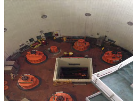
Low Lift Pumping Plant at Northeast WTP
