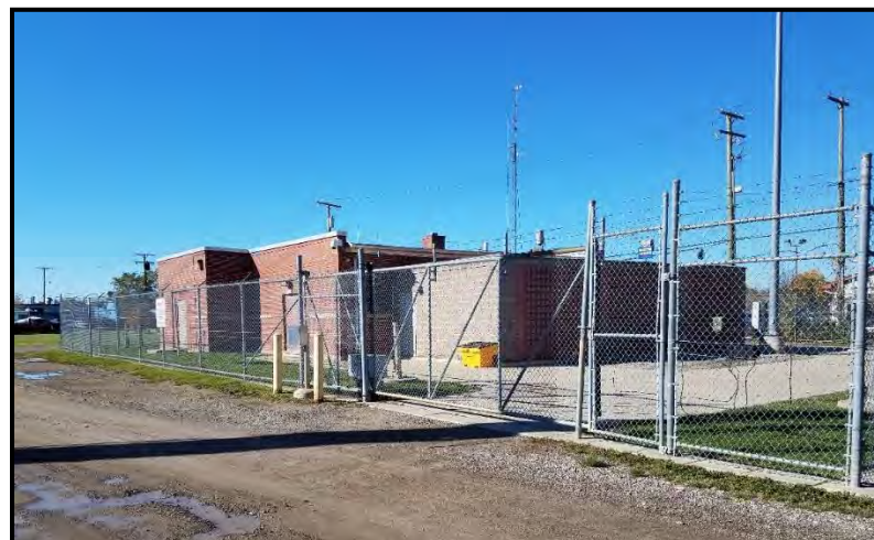
Figure VI-26. Michigan Avenue Pump Station
