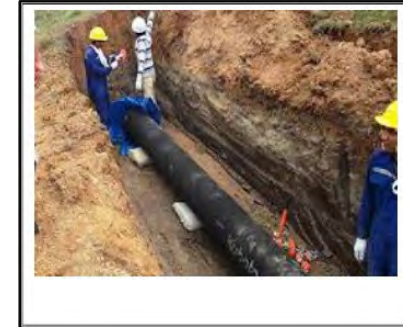
Water main being installed
