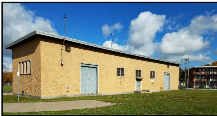
Figure VI-21. Eastside Pump Station
