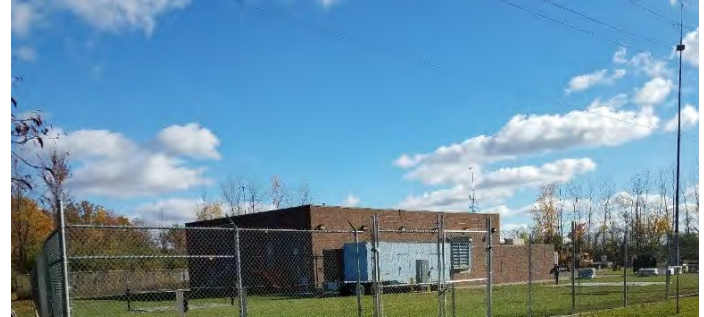
Ypsilanti Pump Station
