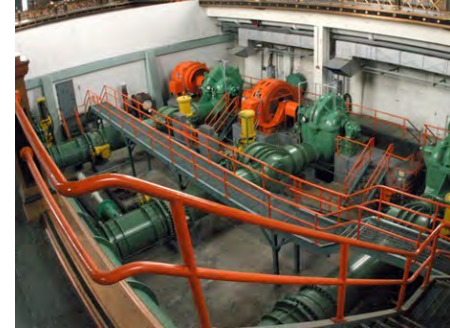
Pumps and Piping
