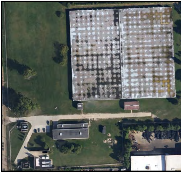
Figure VI-34. West Service Center
