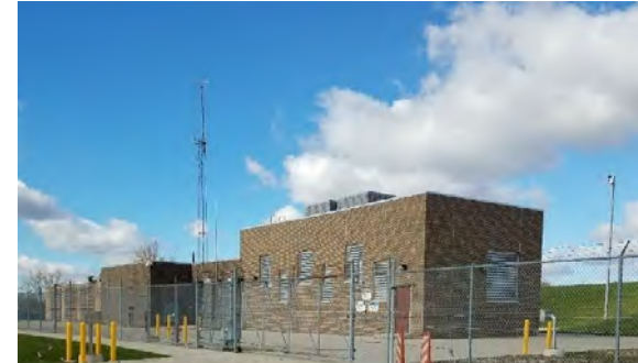
Wick Road Station
