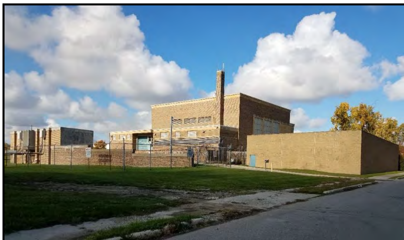
Figure VI-59. Freud Pump Station
