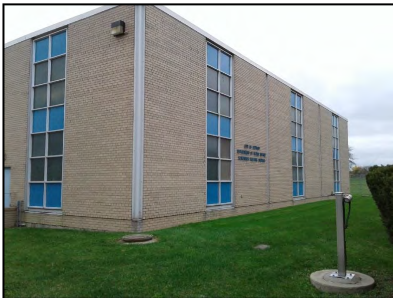
Figure VI-29. Newburgh Pump Station
