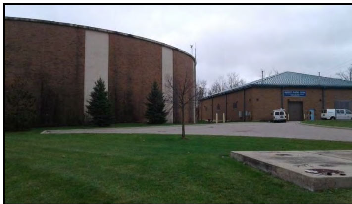
Figure VI-23. Haggerty Pump Station
