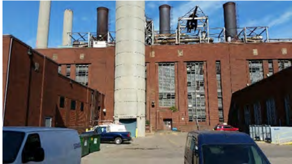
Complex – I Incinerator Building at the WRRF
