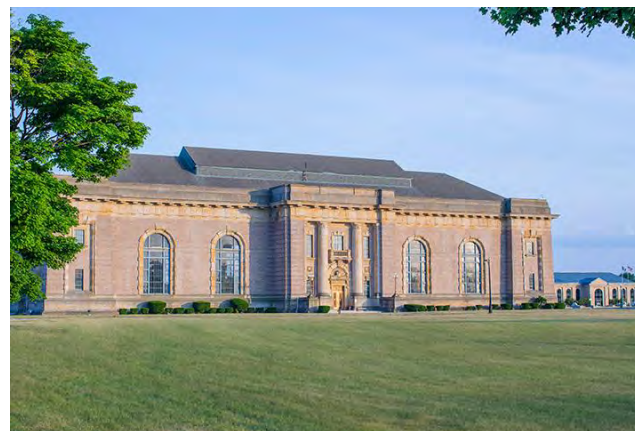
Figure VI-10. Water Works Park WTP
