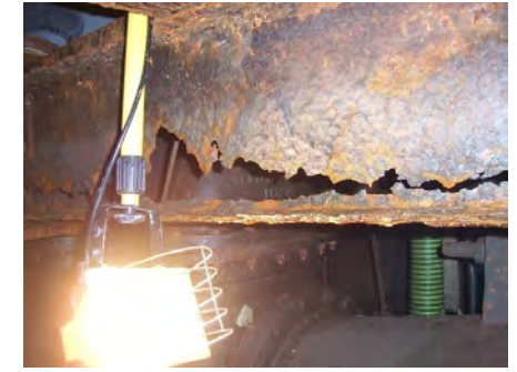
Deteriorated support beams holding up Low Lift Station. Dewatering and Sump Pumps at Elev. 42'-0" (left). Deteriorated grating and access ship's ladder in Low Lift Station - Looking down at Elev. 50'-0" and 42'-0" from Elev. 62'-0" (right).
