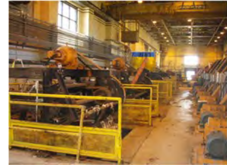
Rack and Grit
