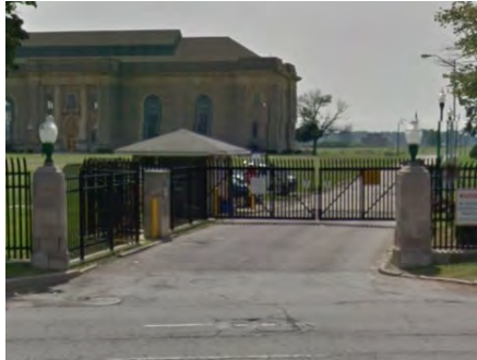
Water Works Park
