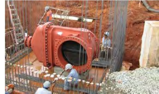
A large valve for a transmission pipe
