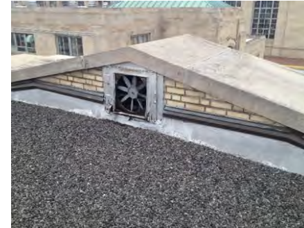
Springwells filter building
