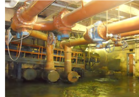
Sludge Feed Pumps
