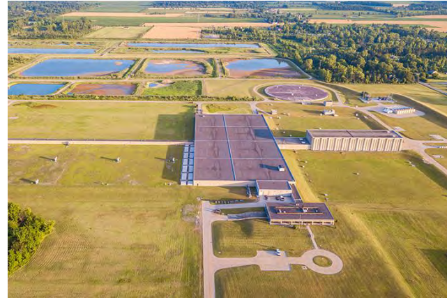
Figure VI-3. Lake Huron WTP
