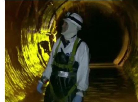
Example inspection of a large sewer
