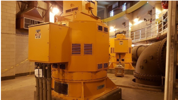
Main Raw Sewage Pumps at Pump Station 2
