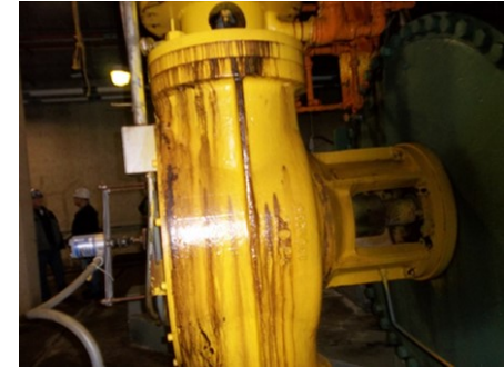
Oil hydraulic valve actuators leaking oil
