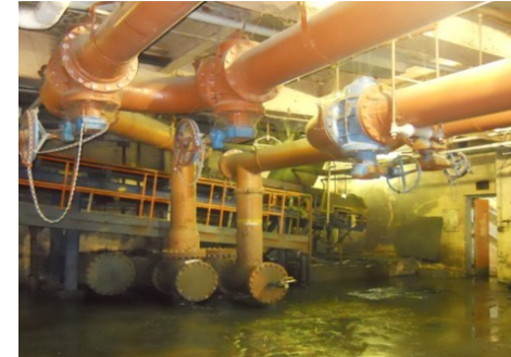
Sludge Feed Pumps
