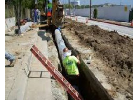
Water main being replaced
