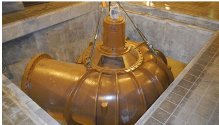
Pump No. 11 installation
