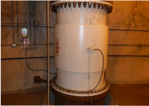
New Flowmeter for Pump No. 11
