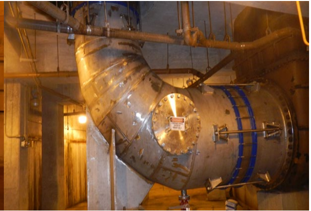
New Suction Elbow for Pump No.
