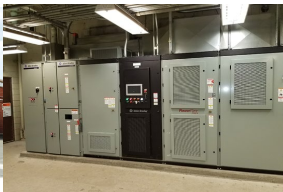
NEW VFD INSTALLED
