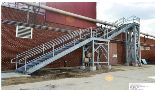
NEW EGRESS STAIRS INSTALLED FOR ROOF ACCESS, EB-10
