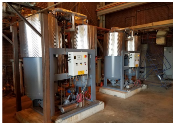
NEW AIR DRYERS INSTALLED
