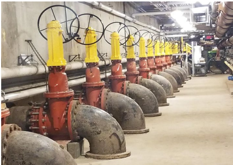
PIPE GALLERY: New Influent Gate Valves for clarifiers 7 and 8 – Phase III
