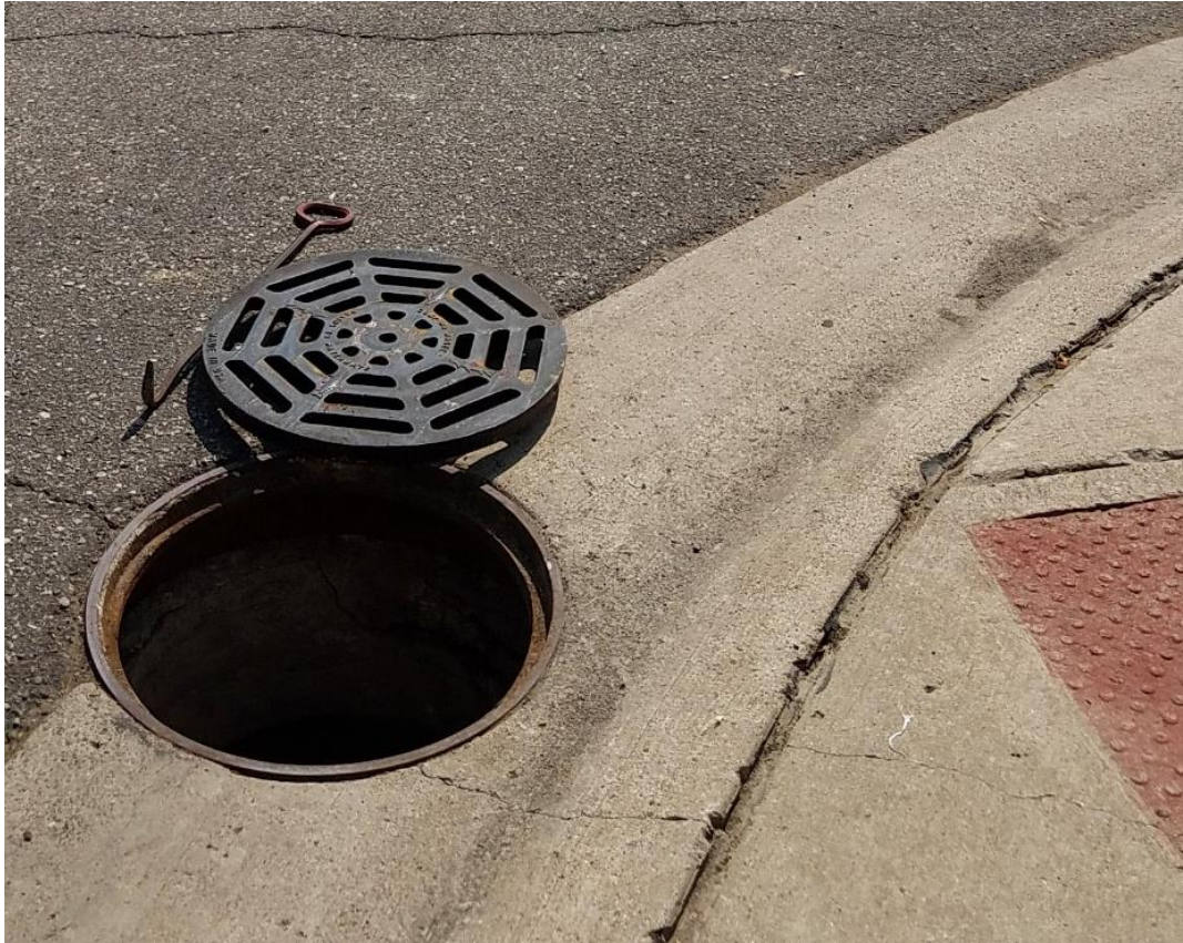
Figure 2-18 Grated Manhole to Enable Cellular Communication of DMA data
