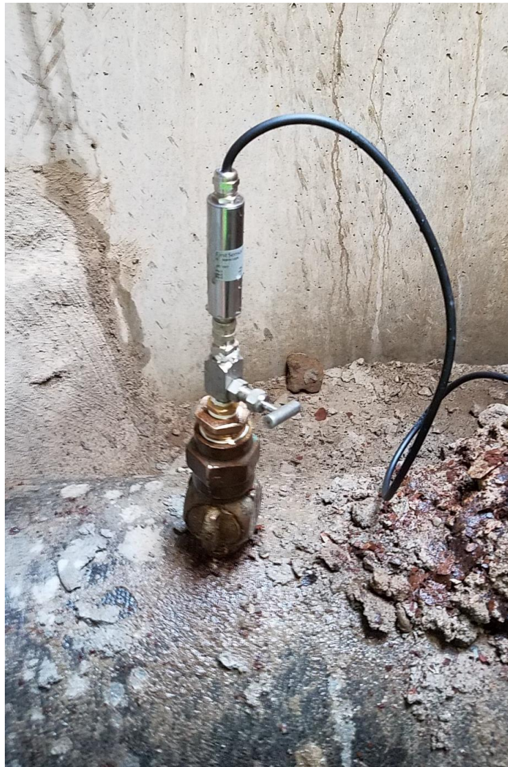
Figure 2-22 Example Installation of Pressure Logging Infrastructure
