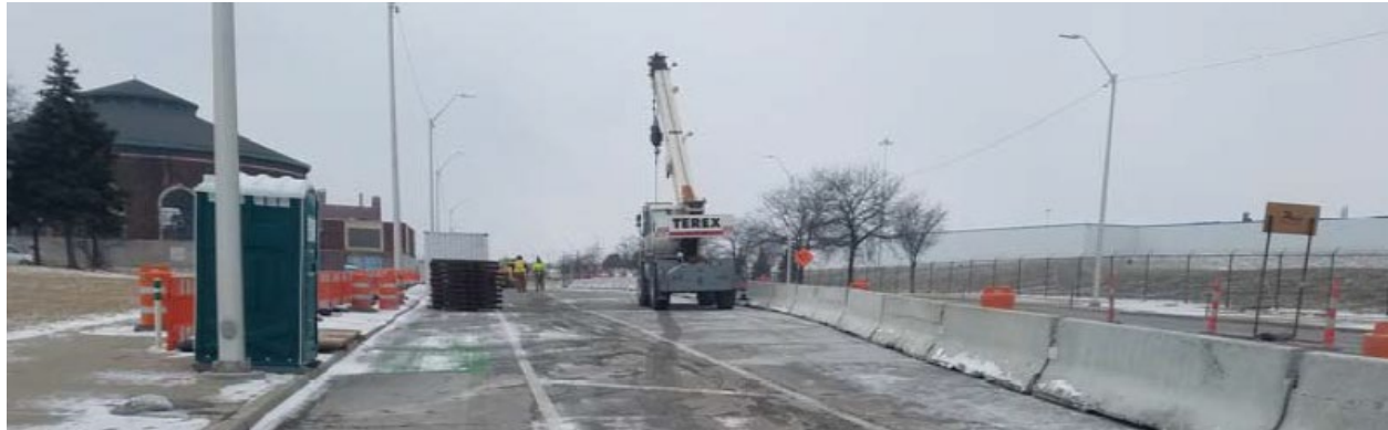
Barrier Installed at work zone east bound Jefferson at Connor for Access Shaft
