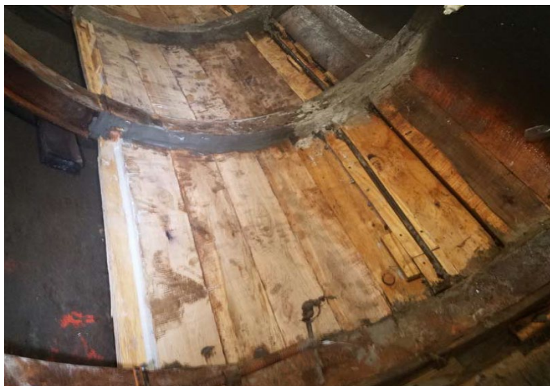
Lagging Installation between Ribs
