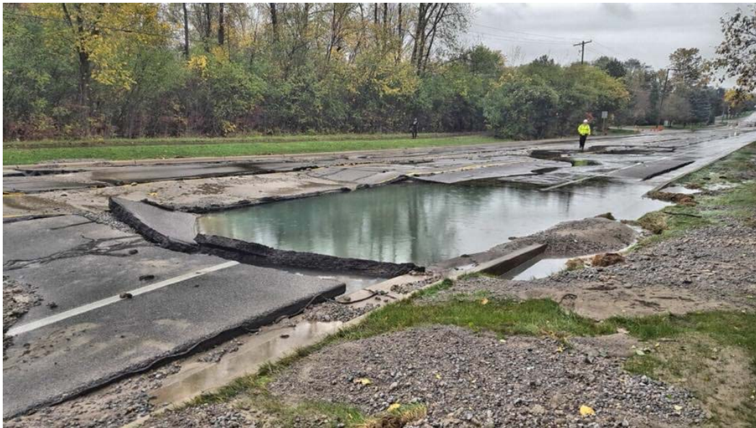
Figure 4.1 – Aftermath of the 2017 14 Mile TM pipeline failure
