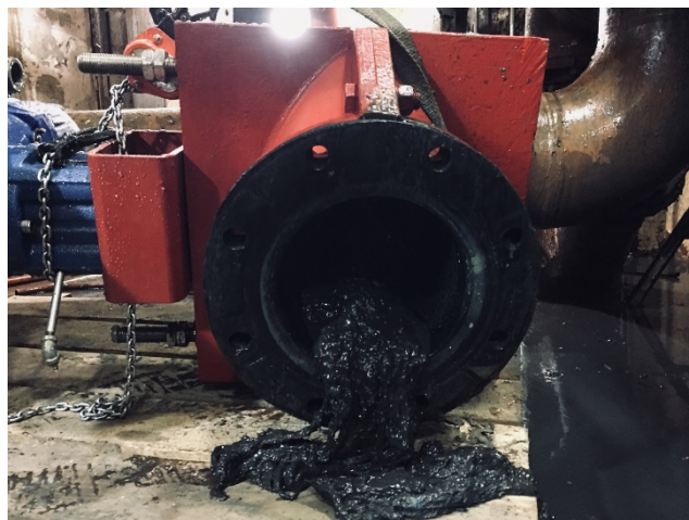
Fully ragged sludge flow control valve
