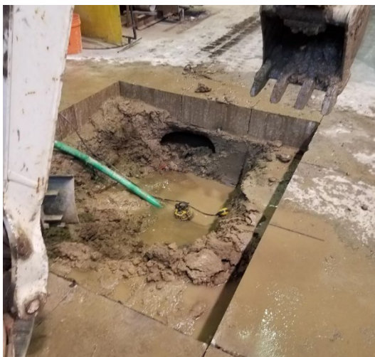
4" water main repair under floor of the maintenance building.
