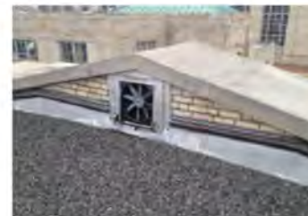
Springwells filter building
