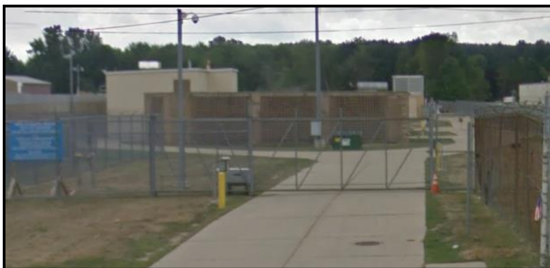
Figure VI-27. Joy Road Pump Station
