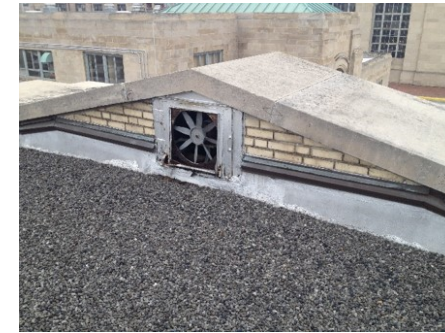
Filter Building roof
