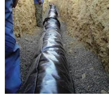
Water main being laid
