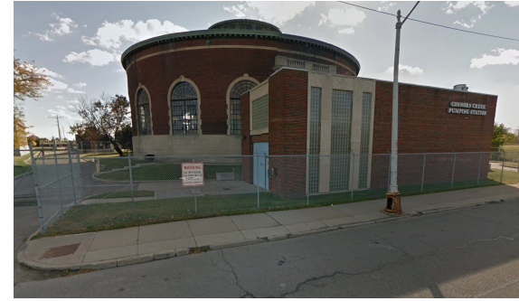
Freud Pump Station
