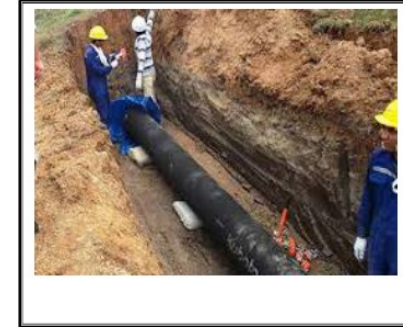
Water main being installed
