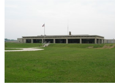
Lake Huron Water Treatment Plant
