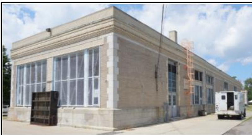
Figure VI-57. Fairview Pump Station
