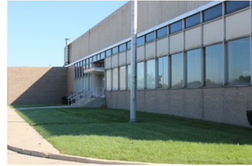
Southwest Water Treatment Plant
