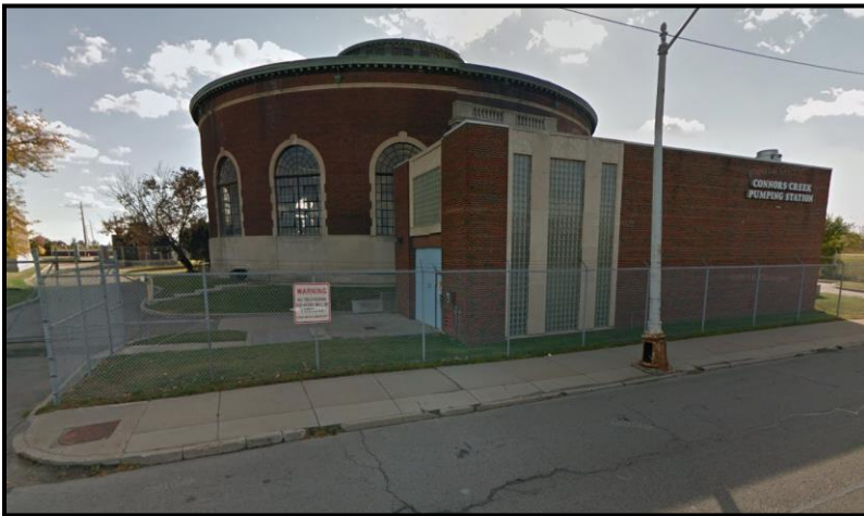
Figure VI-55. Conner Creek Pump Station
