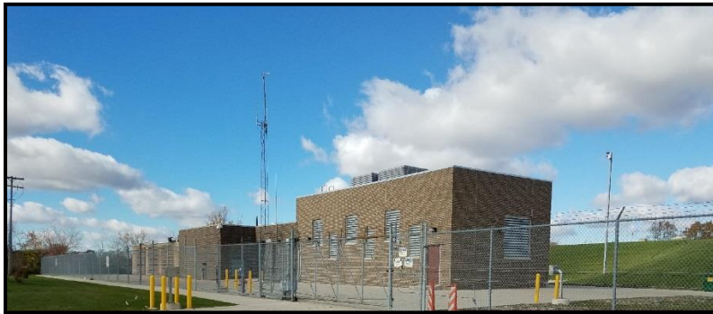
Figure VI-37. Wick Road Pump Station
