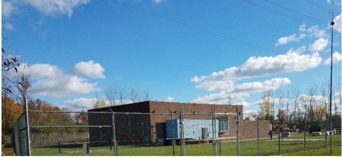
Ypsilanti Pump Station
