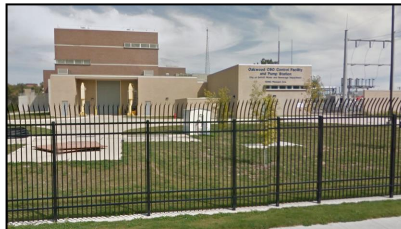
Figure VI-62. Oakwood Pump Station
