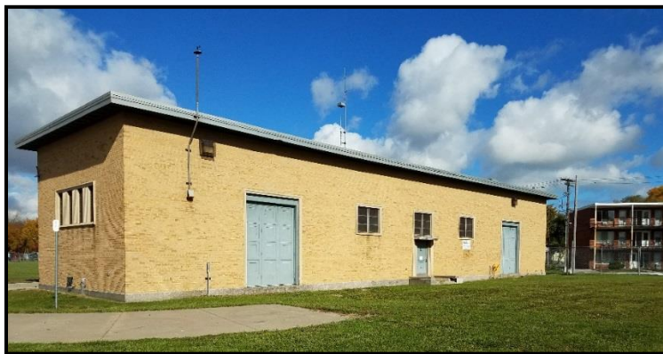
Figure VI-21. Eastside Pump Station
