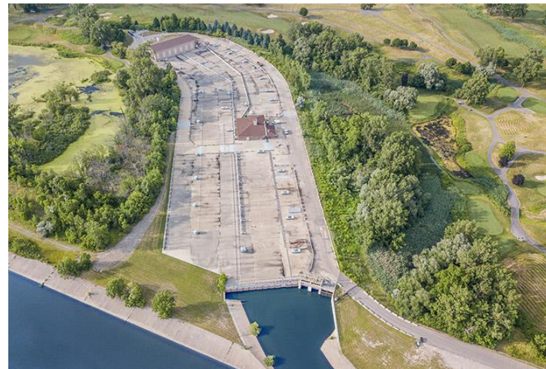
Figure VI-41. Hubbell-Southfield CSO RTB
