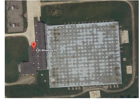
Imlay Pump Station
