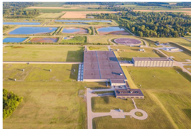
Figure VI-3. Lake Huron WTP
