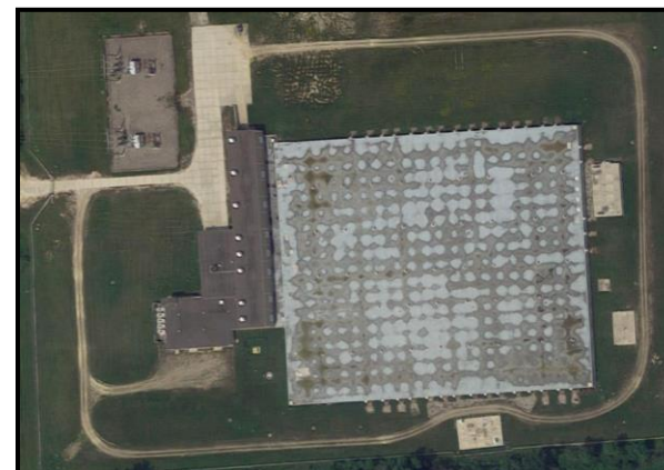
Figure VI-28. Imlay Pump Station
