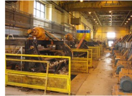
Rack and Grit
