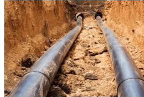
Water main installation
