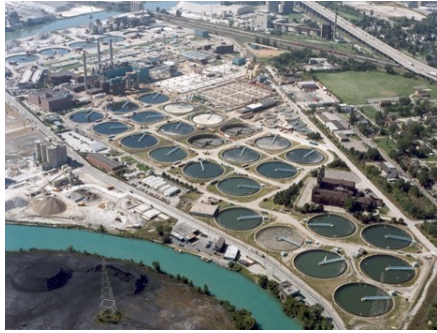
Aerial view of the WRRF
