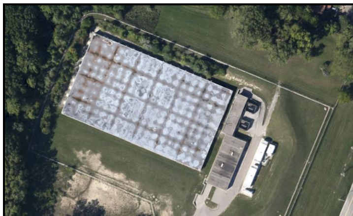
Figure VI-25. Franklin Pump Station
