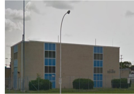
Ford Road Booster Pumping Station
