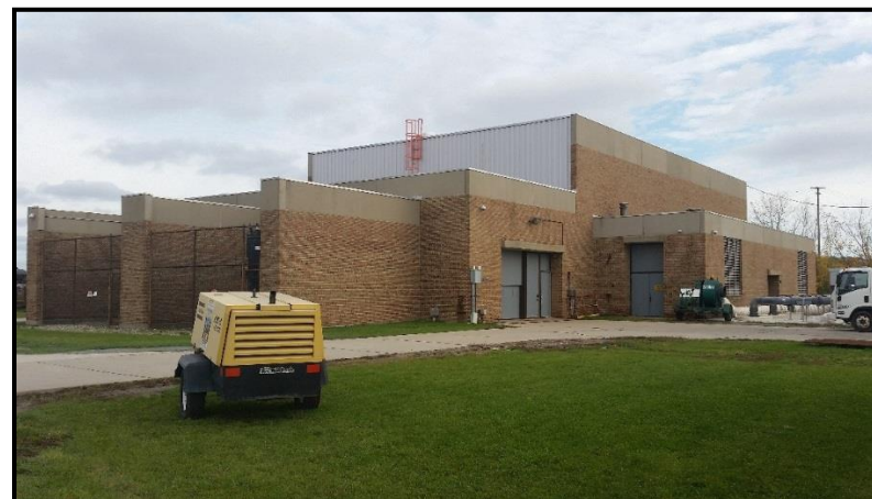
Figure VI-61. Northeast Pump Station
