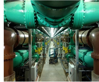
SP-563 – Rehabilitated 1958 Pipe Gallery (in progress)
