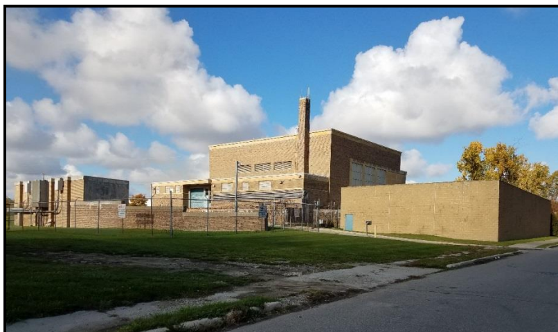
Figure VI-59. Freud Pump Station
