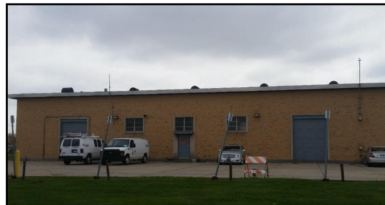
Figure VI-30. Northwest Pump Station
