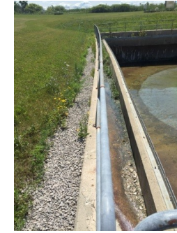
Example of concrete testing
