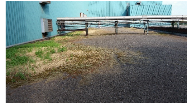
Photo of Complex – I Dewatering Roof at the WRRF.
