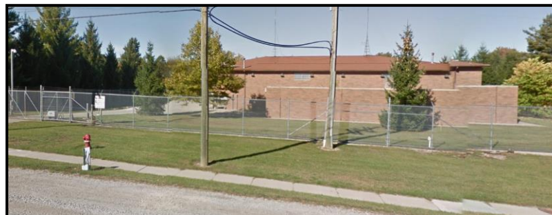
Figure VI-33. Rochester Pump Station
