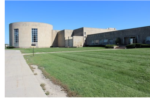
Northeast Water Treatment Plant
