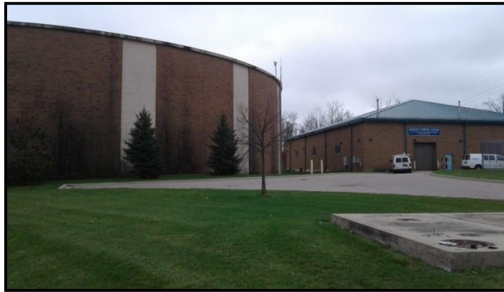
Figure VI-23. Haggerty Pump Station
