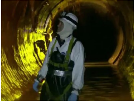
Example inspection of a large sewer
