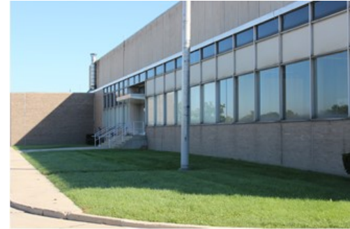
Southwest Water Treatment Plant
