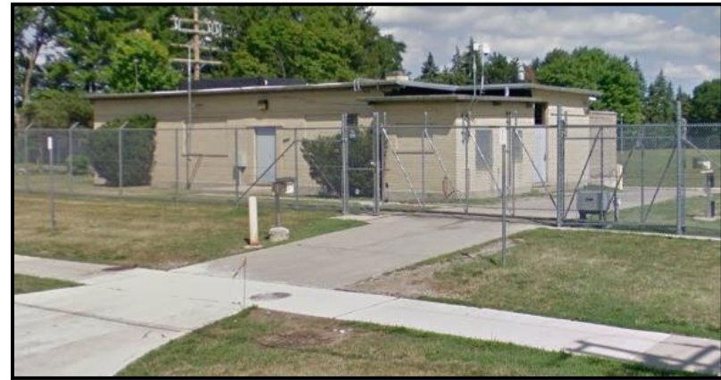
Figure VI-36. West Chicago Pump Station
