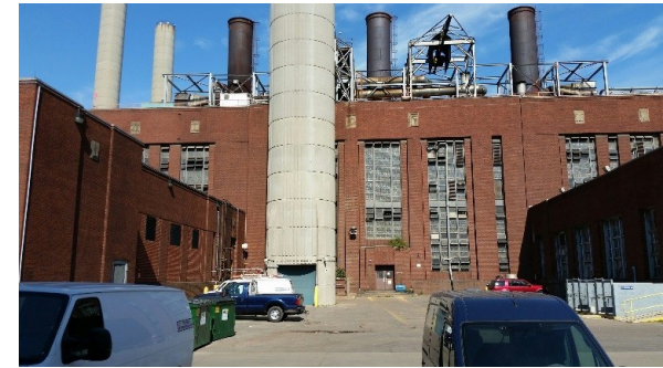
Complex – I Incinerator Building at the WRRF
