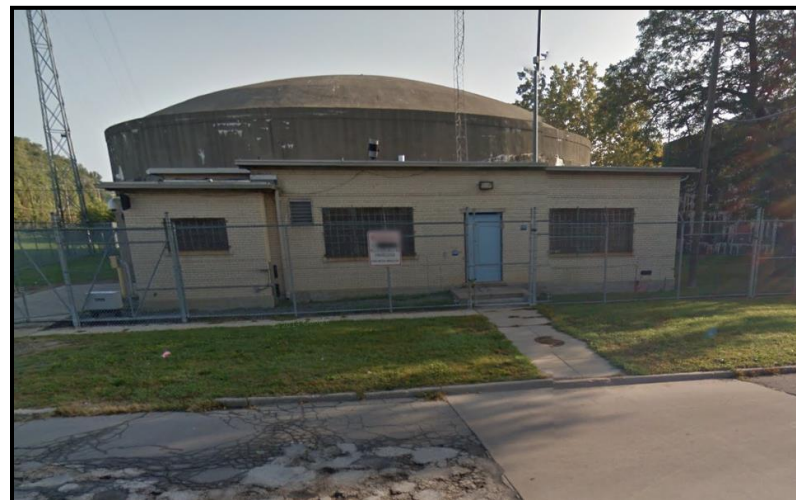
Figure VI-22. Electric Avenue Pump Station
