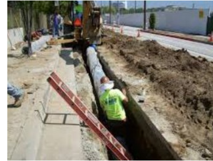
Water main being replaced
