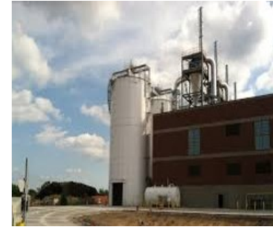
New GLWA Biosolids Dryer Facility
