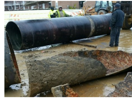
Water main replacement
