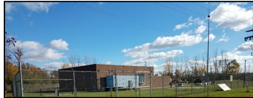
Figure VI-38. Ypsilanti Pump Station
