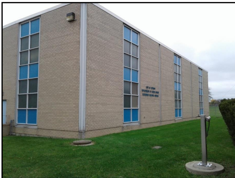
Figure VI-29. Newburgh Pump Station
