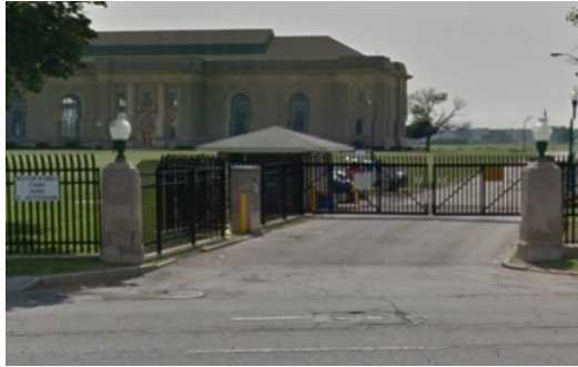
Waterworks Park WTP
