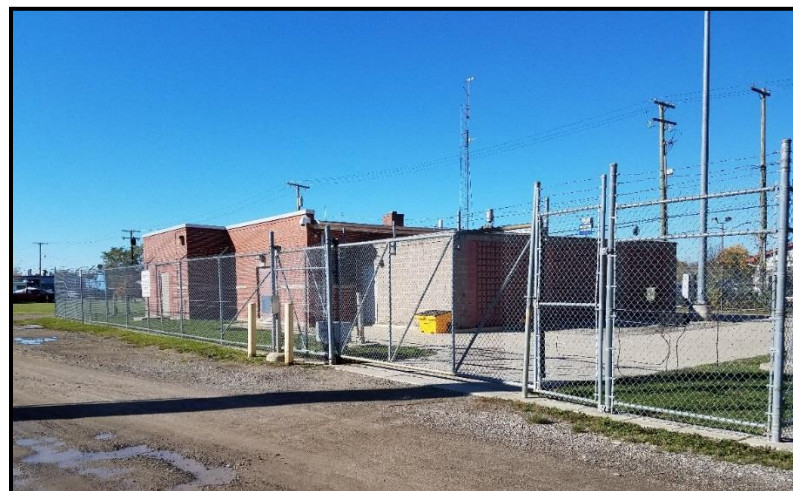
Figure VI-26. Michigan Avenue Pump Station
