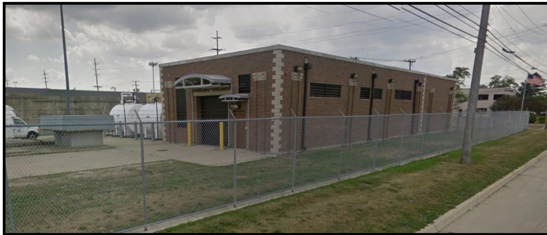
Figure VI-35. Schoolcraft Pump Station
