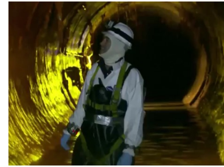
Visual inspection of a large sewer
