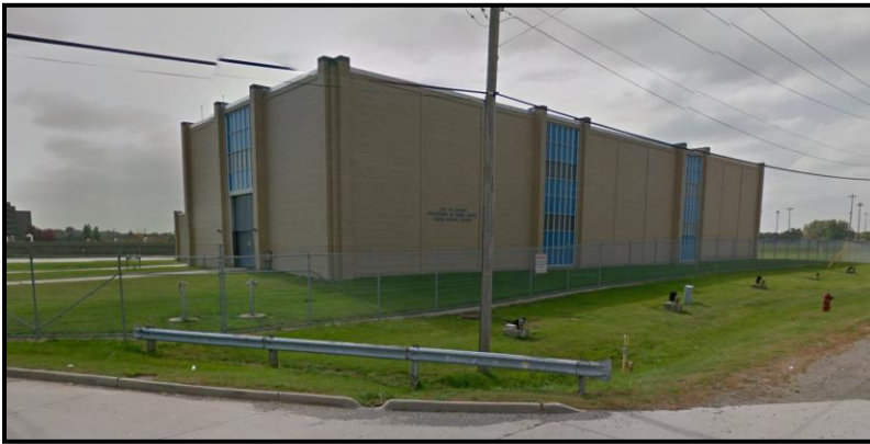
Figure VI-31. North Service Center
