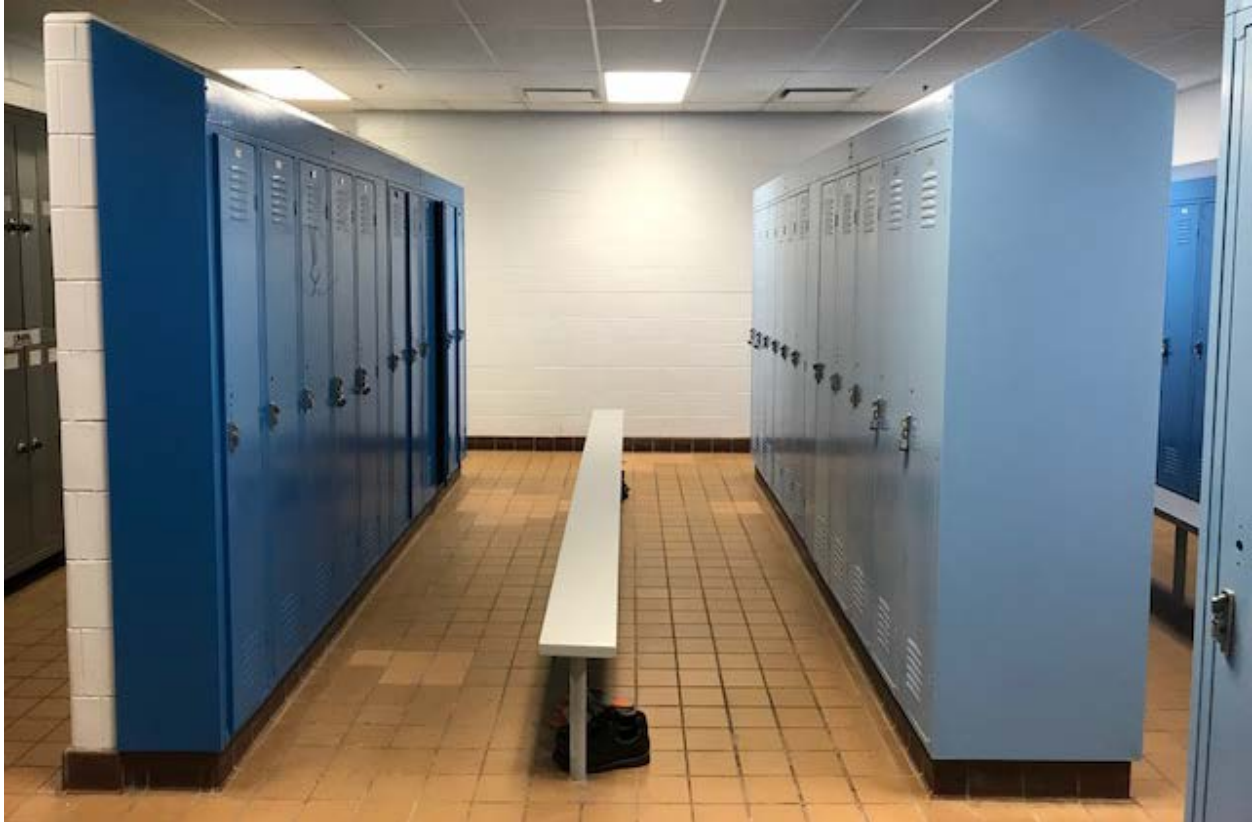
Newly repaired floors and repainted lockers at WRRF
