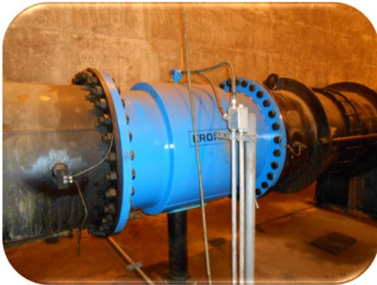
Magnetic flow meter on 36 inch force main
