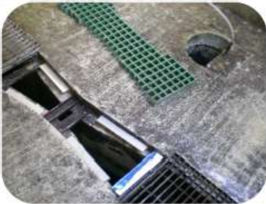
Parshall flume with bubbler tube and stilling well on the right
